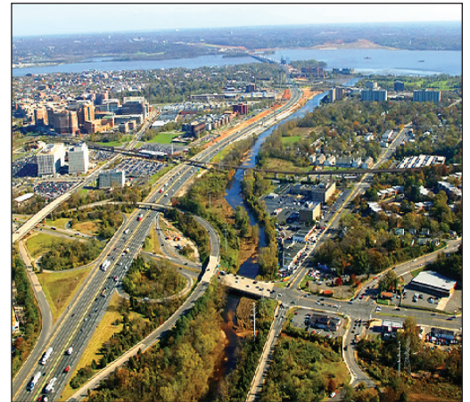
Capital Beltway/I-495 high-occupancy toll lanes was the first project to utilize PABs.
