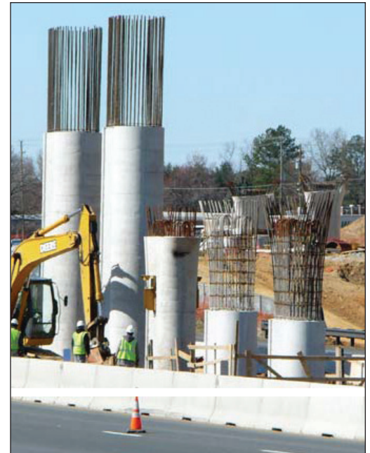
Maryland's Intercounty Connector uses GARVEEs.
