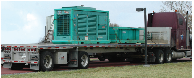
Following Hurricane Katrina, emergency generators were trucked to the devastated areas under special permits.
