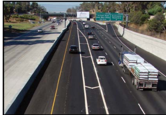
Figure 6-6: Slip Ramp Access to the I-680 HOT Lane, Alameda County, CA
