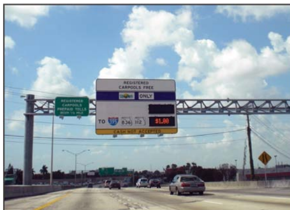
Figure 6-19: Variable Message Sign on the I-95 Express in Miami
