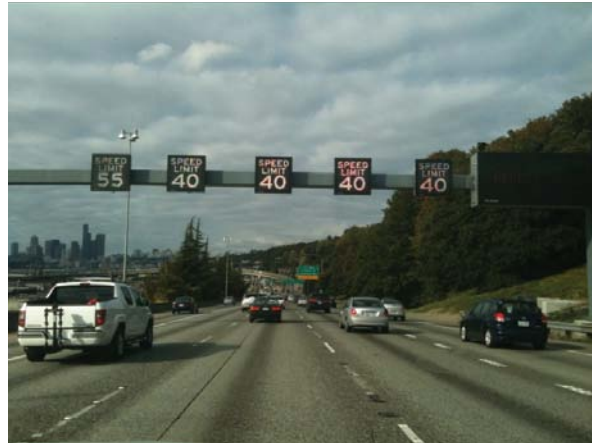
Figure 7-1: Active Traffic Management Deployed on I-5 in Seattle
