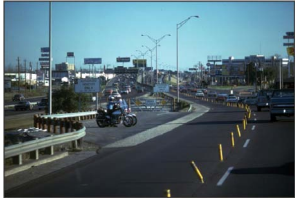
Figure 6-20: Enforcement Area on I-45 in Houston
