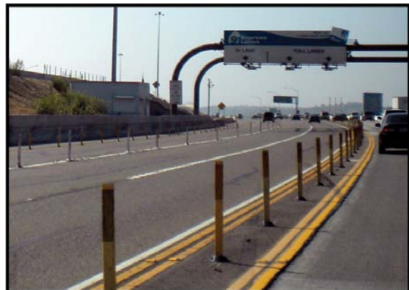
Figure 6-14: Individual Pylon Separation on the SR 91 Express Lanes
