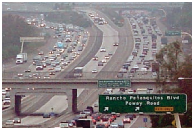
Barrier separation on 2-lane reversible I-15 Express Lanes
