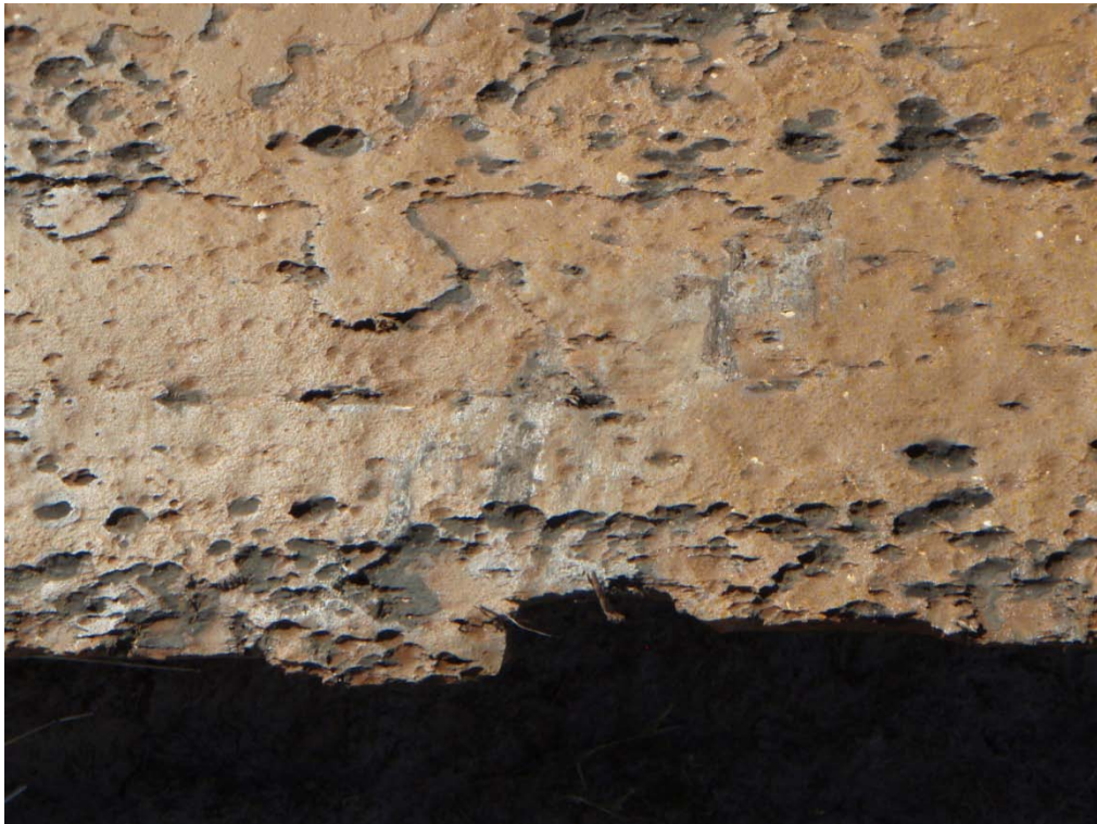
Figure D4 – Internal surface of pipe
