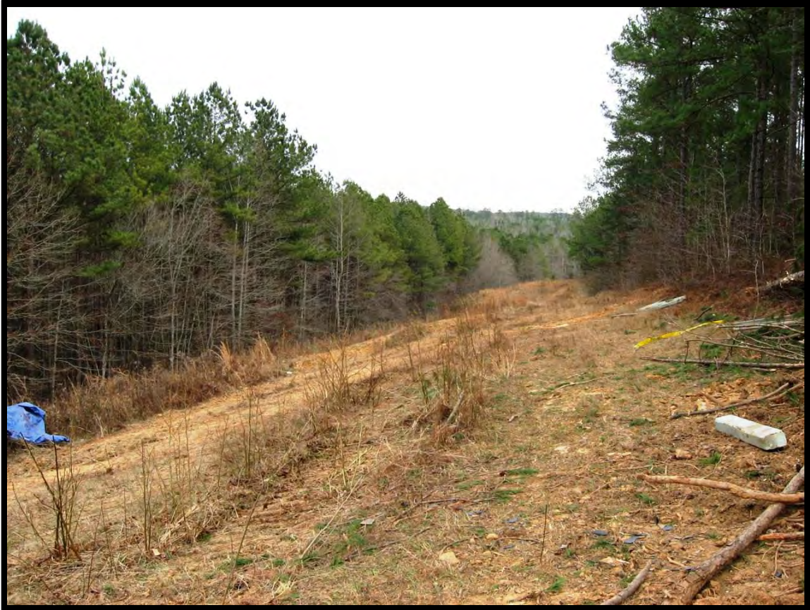
PHOTOGRAPH 1. PIPELINE RIGHT-OF-WAY EAST OF RUPTURE (VIEW IS TOWARD EAST)
