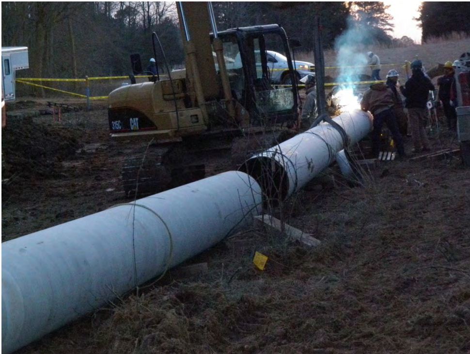
Welding of new replacement pipe
