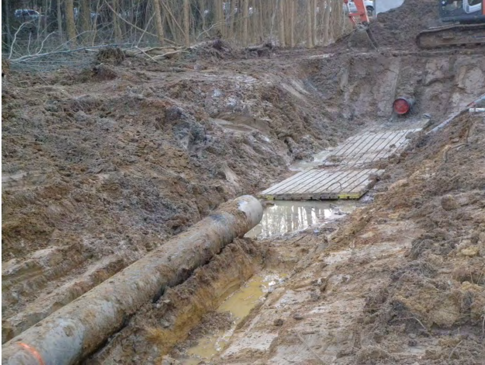
2 nd North Main Line failure area getting prepared for repair
