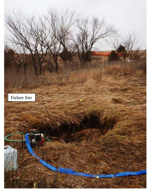
Pipeline rupture at wrinkle bend (underbend), looking southeast.
