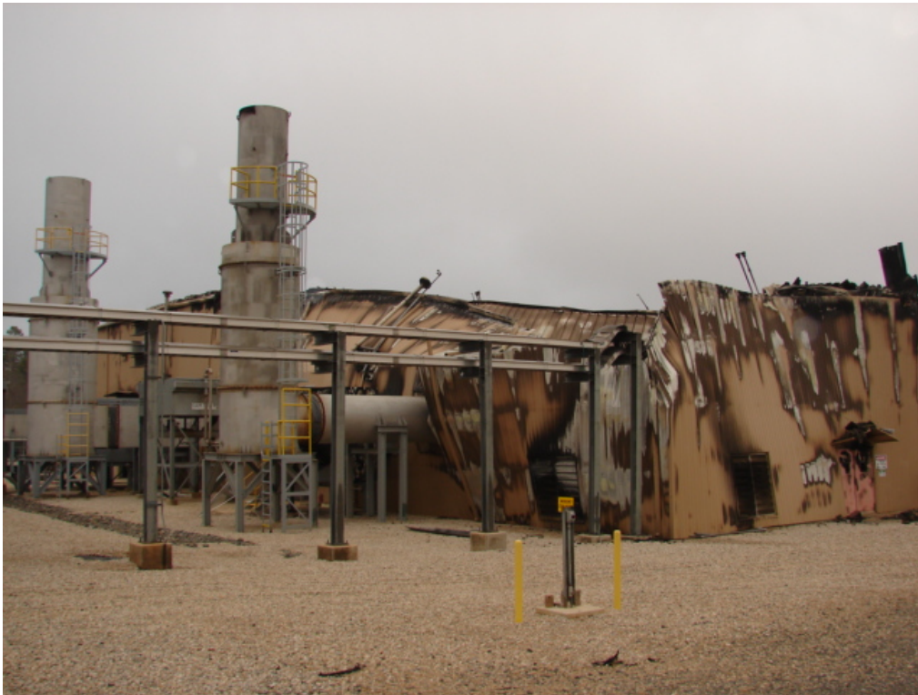
Figure 1-Carthage Junction Compressor Building
