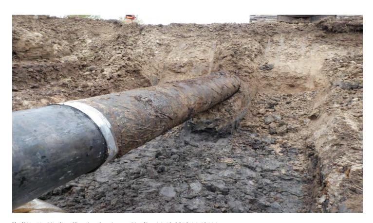
Shell Ho-Ho Pipeline Showing Coating on Pipeline 11-19-2010 11:43AM
