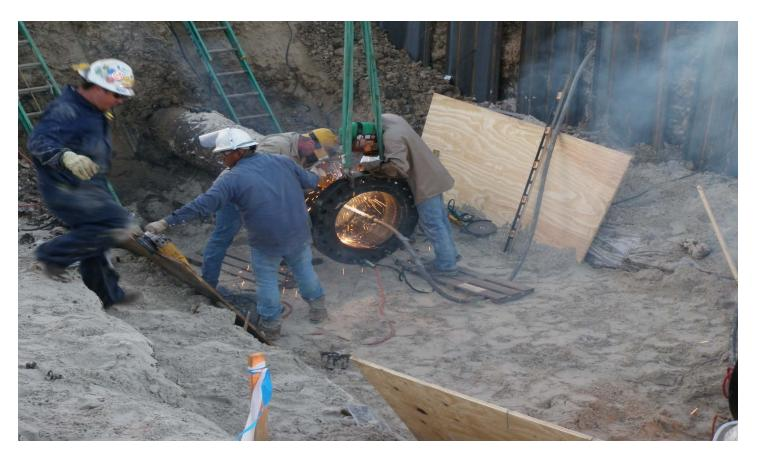
Shell Ho-Ho Pipeline Welding Flange for Spool-Type Repair 11-20-2010 5:51PM
