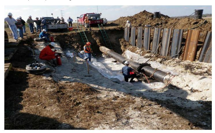
Shell Ho-Ho Pipeline Cold-Cutting Failed Segment 11-20-2010 2:44PM
