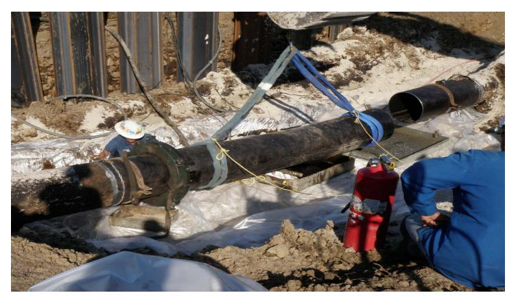
Shell Ho-Ho Pipeline Cold-Cutting Failed Segment 11-20-2010 3:24PM
