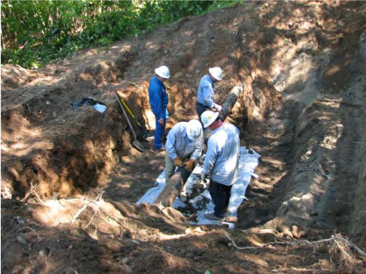
PHOTO 8: COATING REMOVAL DOWNSTREAM DIG 8/30/10
