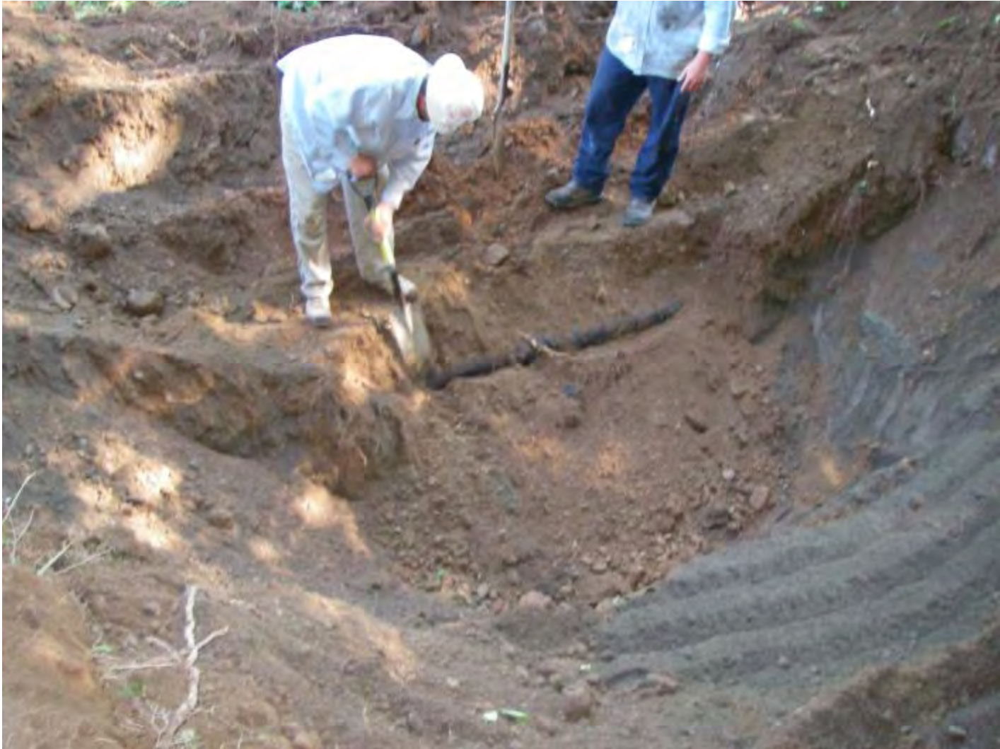
PHOTO 2: EXPOSING PIPE ON DOWNSTREAM DIG 8/29/10
