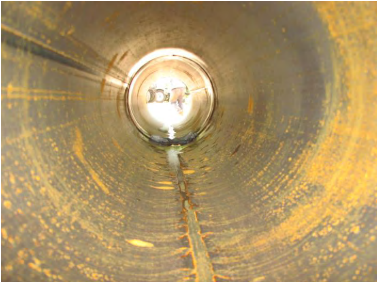
PHOTO 26: INTERNAL VIEW OF PIPE (WD 40 & PLASTIC WRAP VISIBLE) 09/02/10
