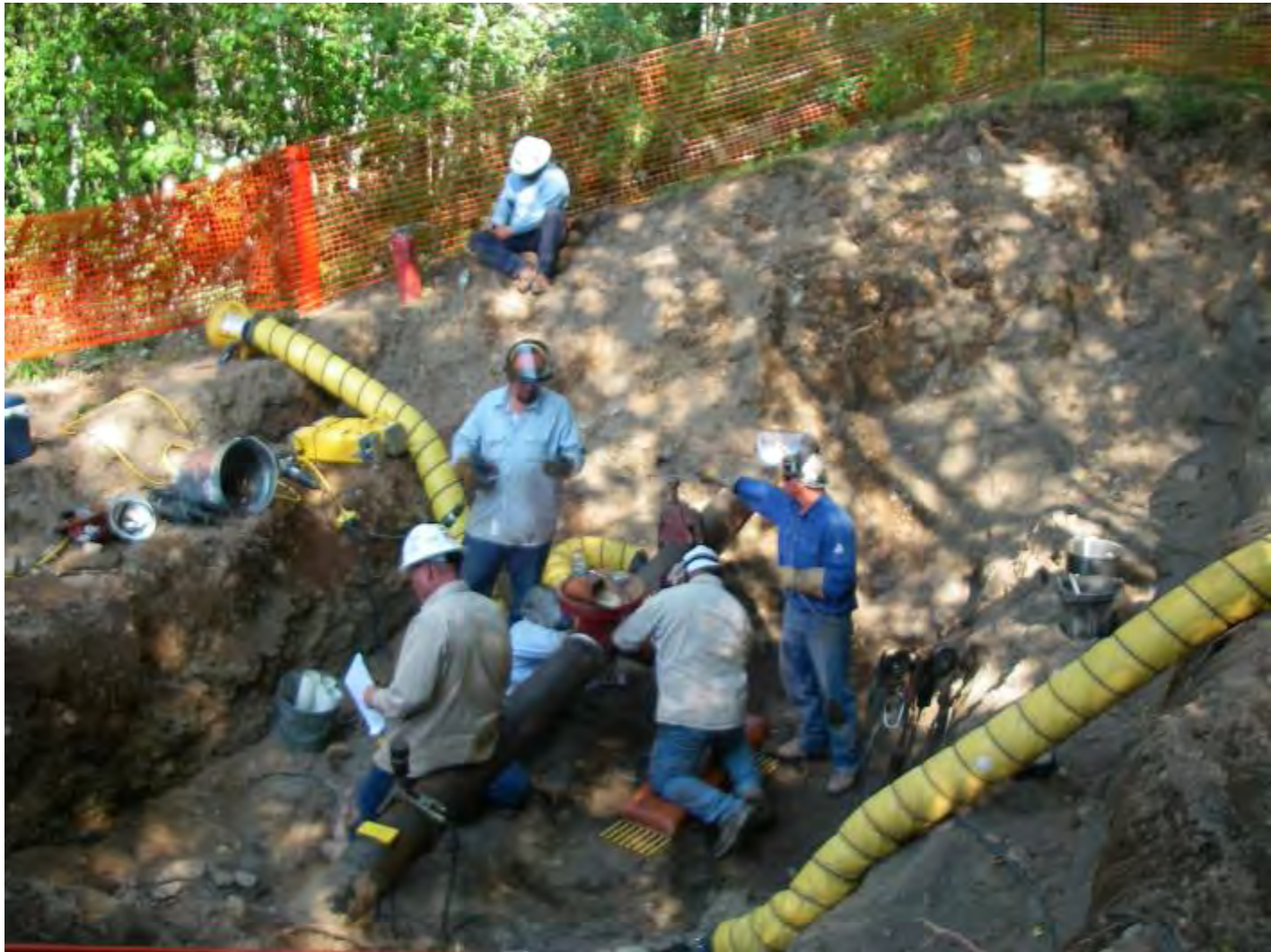
PHOTO 9: WELDING OF DOWNSTREAM STOPPLE 8/30/10
