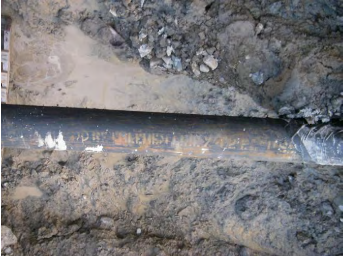
PHOTO 12: PIPE DATA ON TOP OF PIPE UPSTREAM DIG 8/30/10
