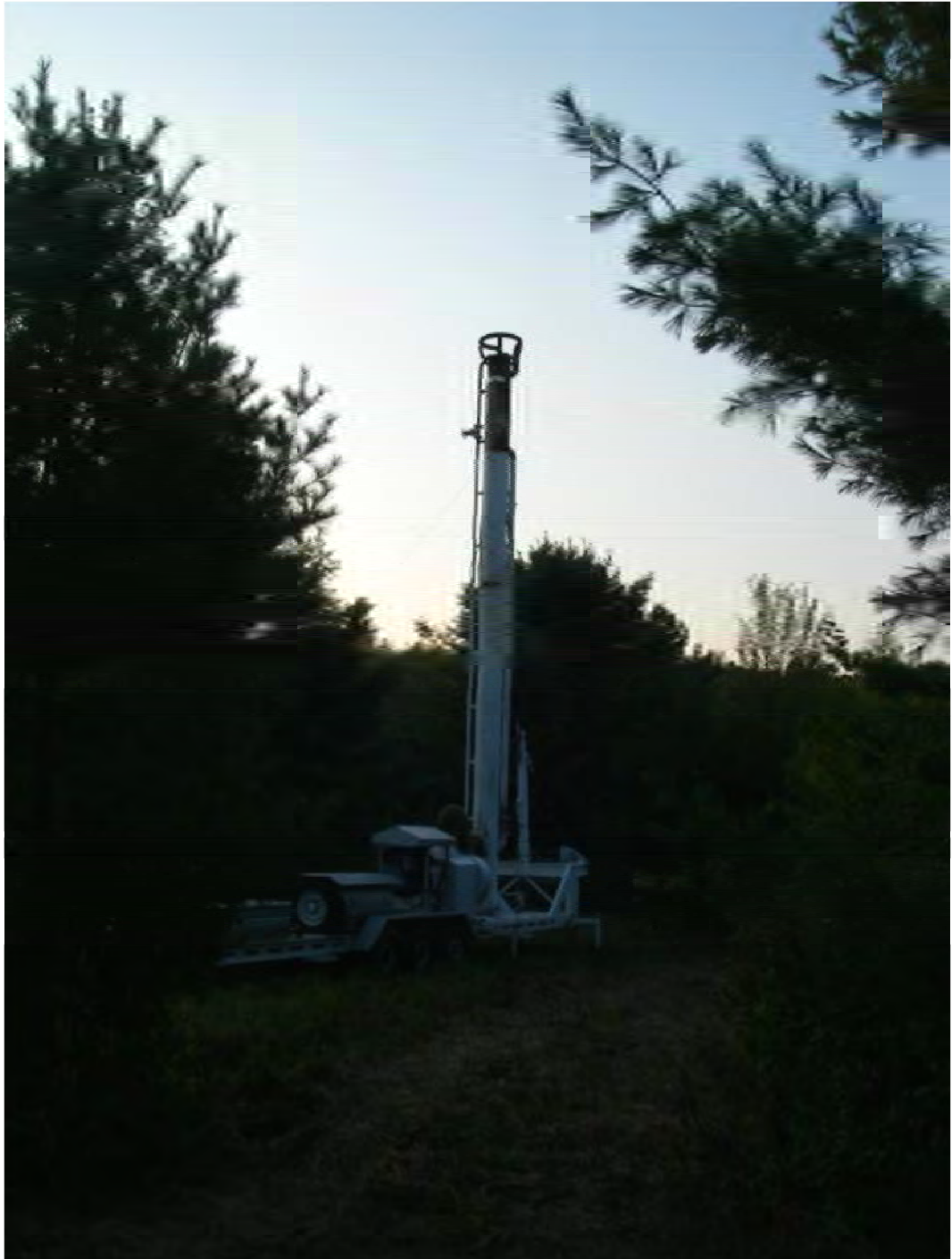
PHOTO 14: FLARE SET UP 8/30/10
