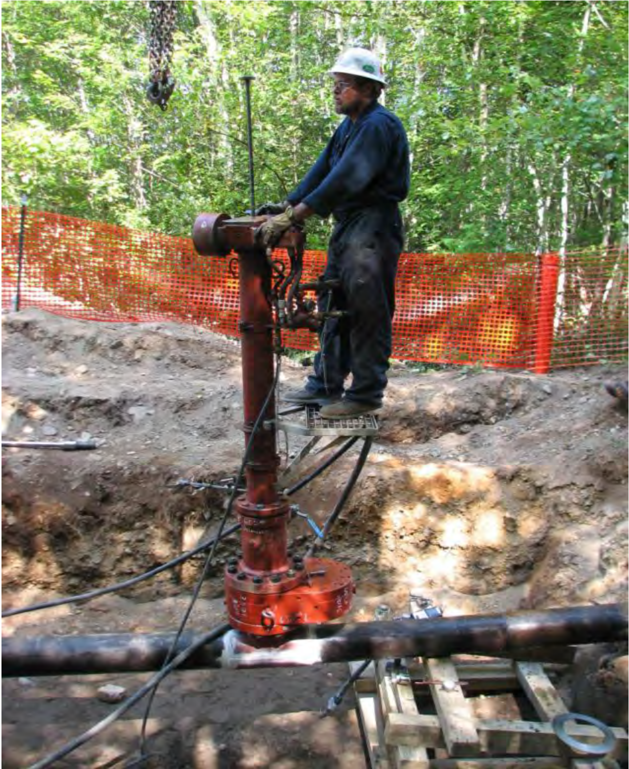
PHOTO 17: TAPPING PIPELINE UPSTREAM DIG 8/31/10
