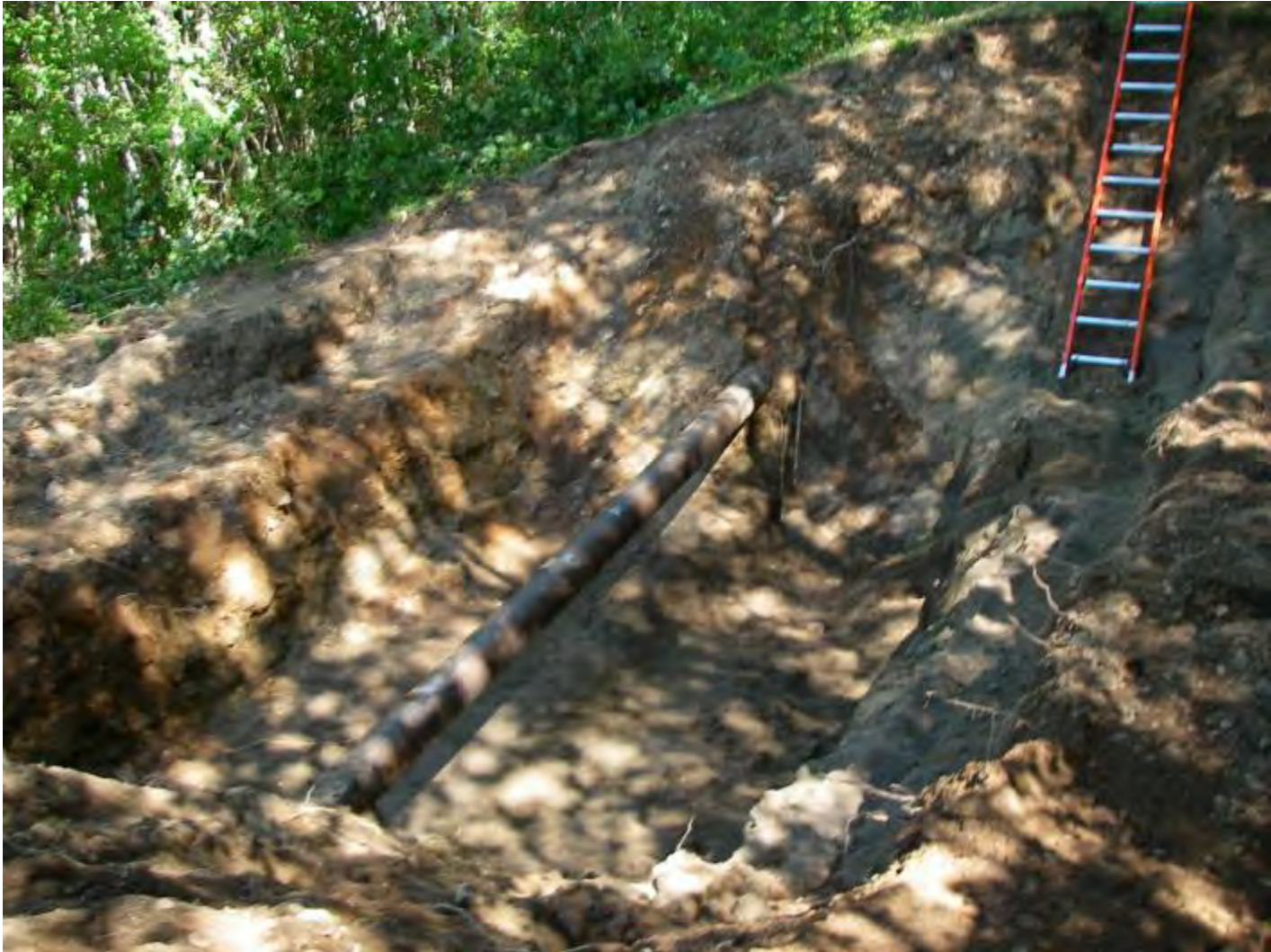
PHOTO 3: FINISHED EXCAVATION DOWNSTREAM DIG 8/29/10
