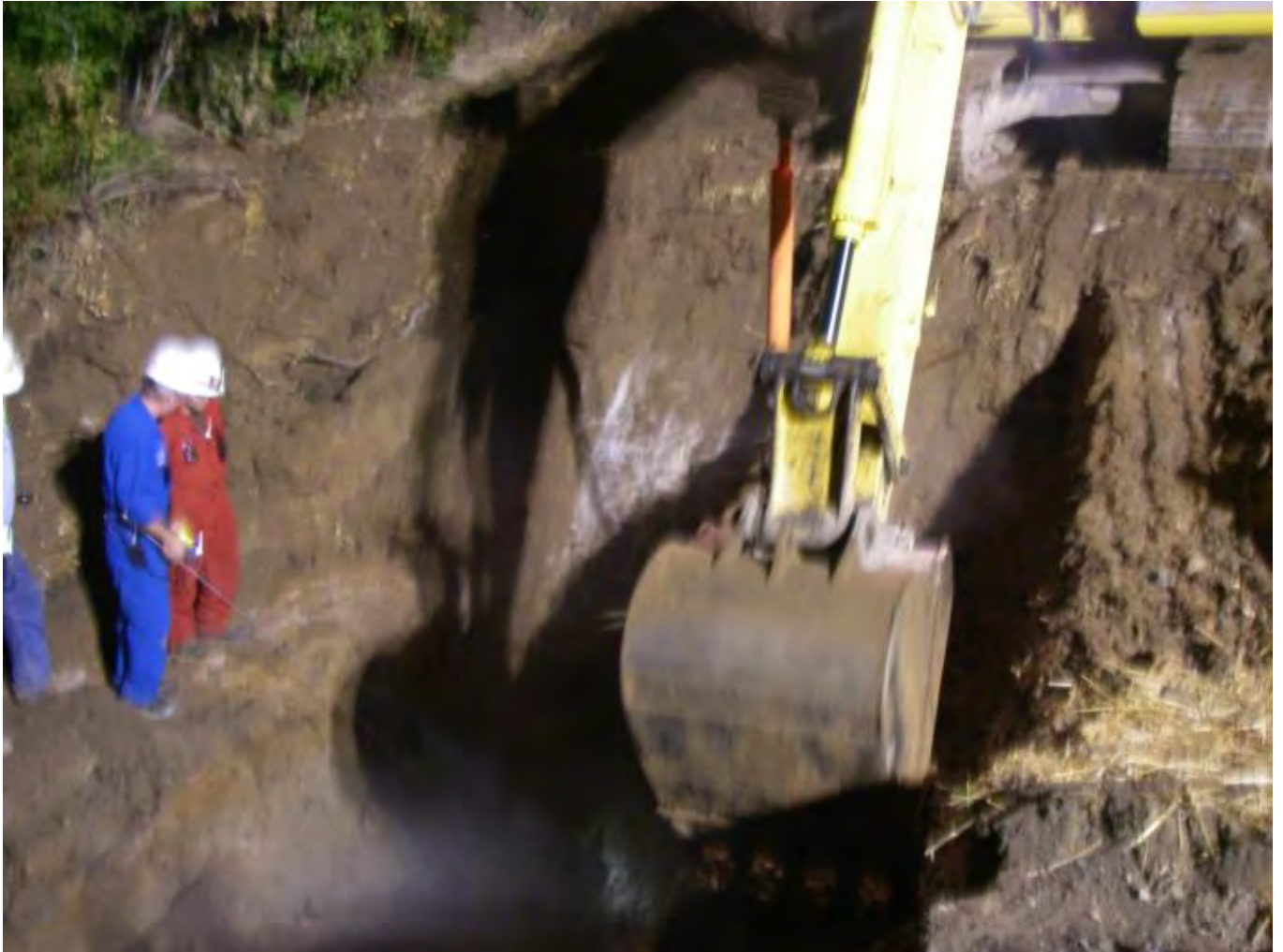
PHOTO 19: EXCAVATING FROST BALL AROUND PIPE 09/01/10
