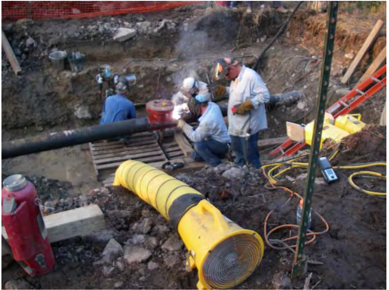
PHOTO 13: WELDING OF STOPPLE FITTING UPSTREAM DIG 8/30/10
