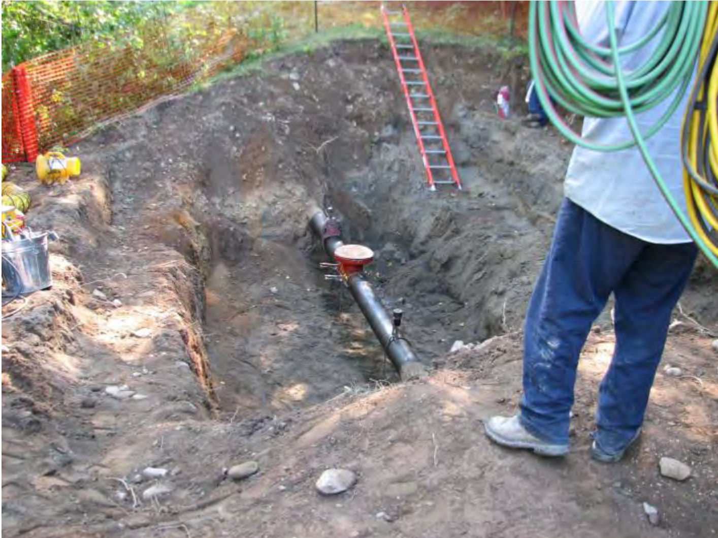
PHOTO 10: COMPLETED STOPPLE FITTING DOWNSTREAM 8/30/10
