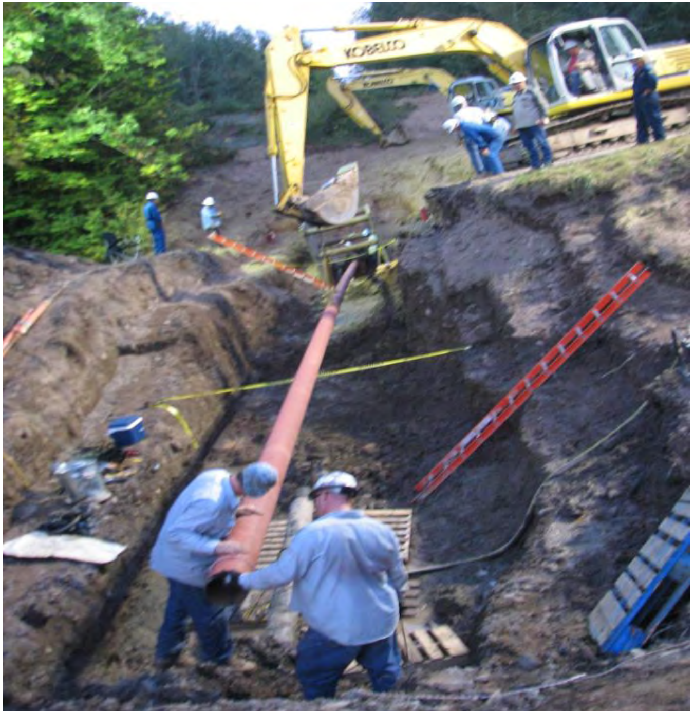
PHOTO 28: NEW PIPE BEING SPOOLED IN UNDER ROAD CROSSING 09/02/10
