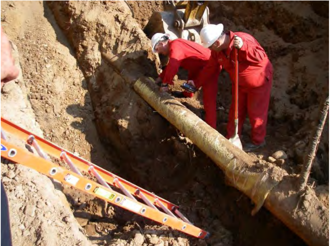
PHOTO 20: CASING, CARRIER PIPE AND VENT STACK EXPOSED, DOWNSTREAM SIDE 09/01/10
