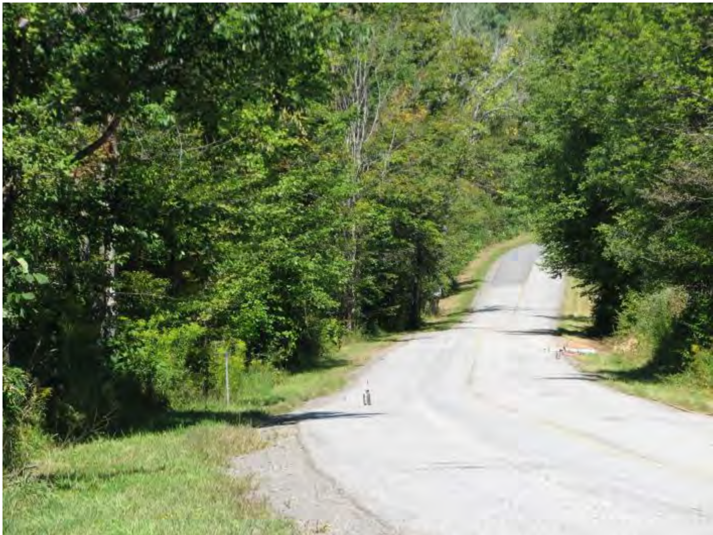
PHOTO 1: FACING NORTH ON KEYSERKILL ROAD (AIR MOVER @ 3:30 POSITION)
