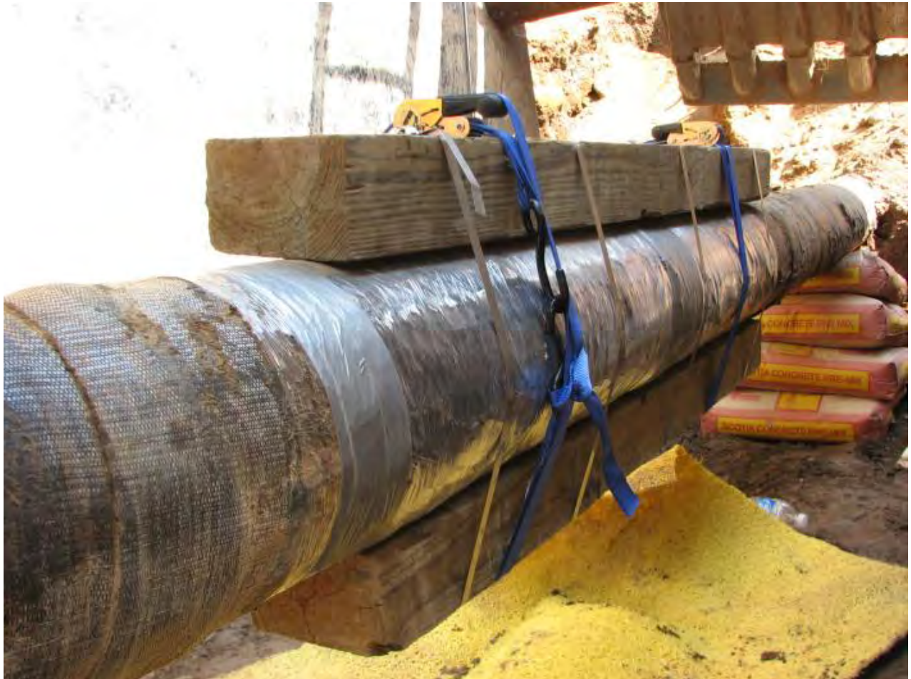
PHOTO 24: PIPE SPECIMEN PREPARED FOR REMOVAL 09/02/10
