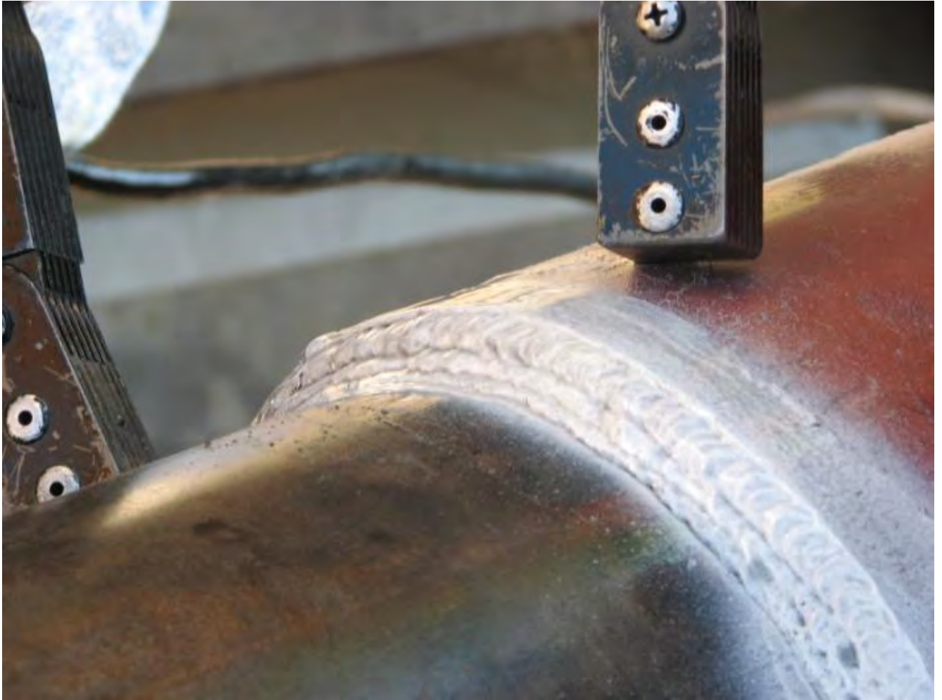
PHOTO 16: MAG PARTICLE 2 UPSTREAM DIG 8/31/10
