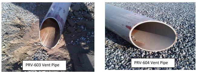
Four (4) Vent Stacks showing only PRV-603 possibly relieved. Operator stated that none of these relief devices have ever actuated prior to 5/2/12. Installation was circa 1991/1992.
