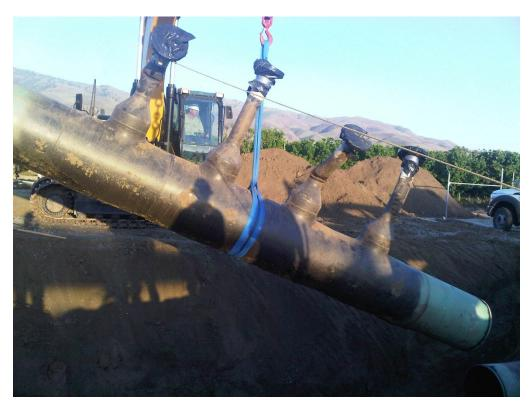
30" RV Header Pipe being removed. Tee outlets are 8" swedged down to 6".
