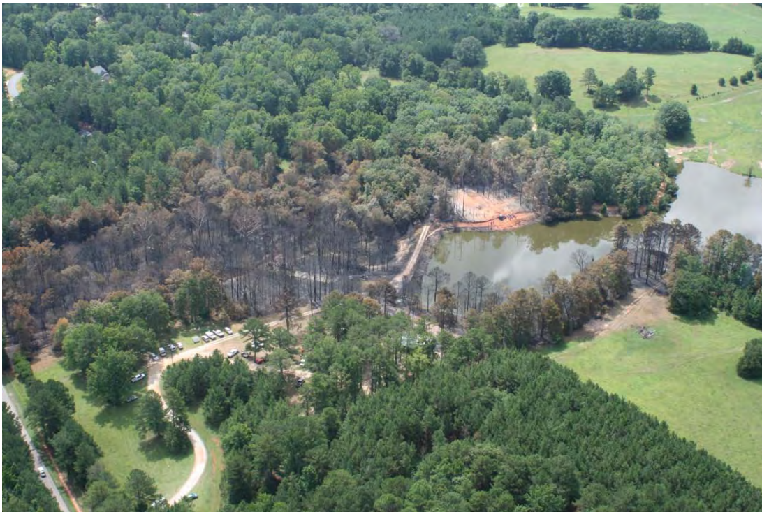
Aerial photo above zoomed in: 390 Stagecoach Road property after the propane fire
