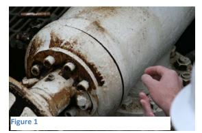
The 10" main line valve had an actuator and motor installed on it. CPL was asked to explain the operation of the valve. It was determined that the valve actuator was designed so during remote operation of the valve, the hand wheel could not move. In fact, the only way to move the hand wheel was to place the valve actuator in manual mode (disengage the motor operator) and then one is able to open or close the valve by moving the hand wheel.
