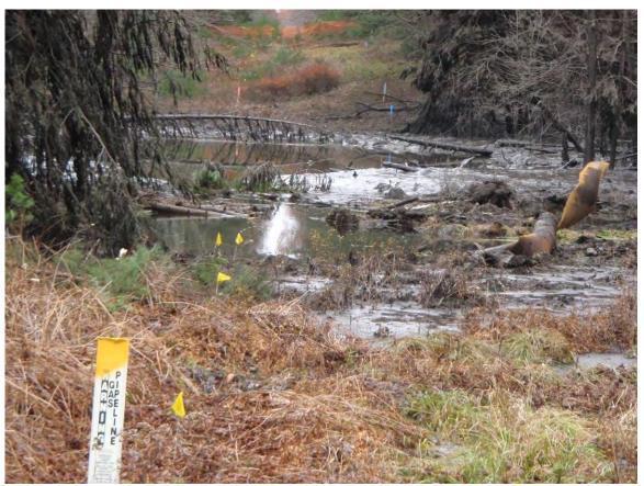
Figure 8: Ruptured pipe in swamp
