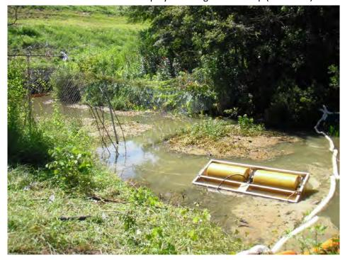
Under-flow dam constructed to prevent jet fuel progression into the Tampa Bypass Canal (Division 4)
