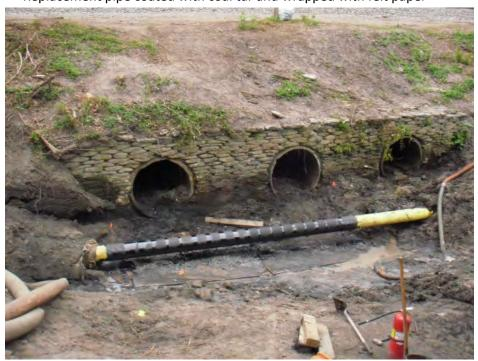
Rock shield installed to protect pipe exterior from future mechanical damage
