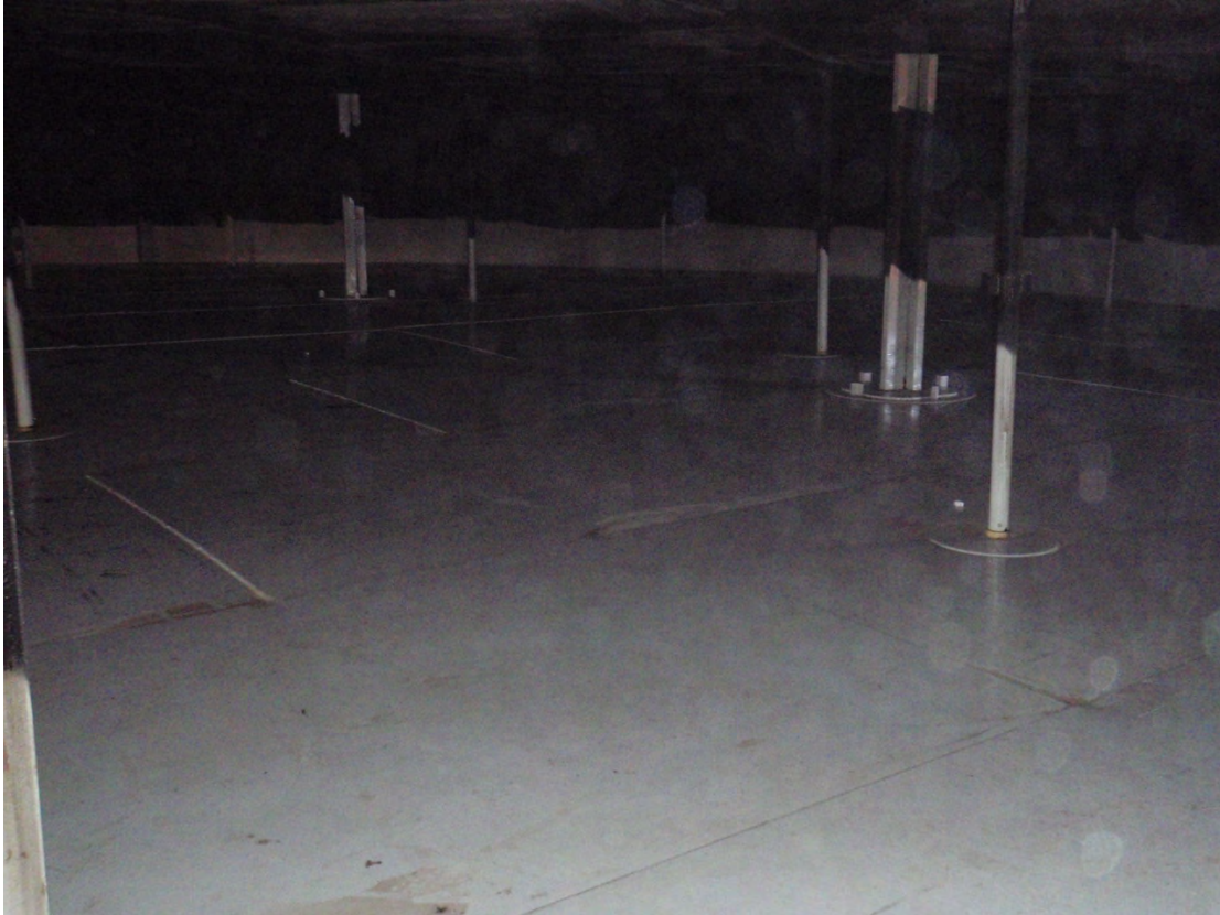
Inside floor of tank 1168. The gray is an internal liner.
