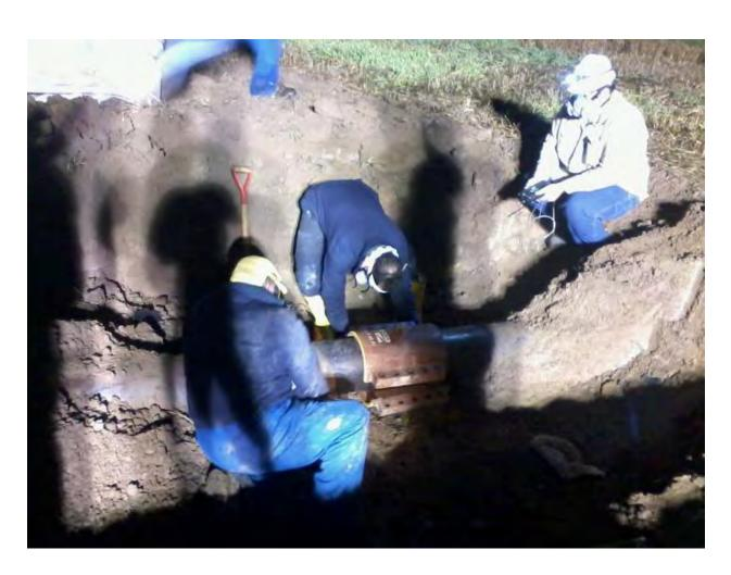
Photo #3: Temporary leak clamp being installed to facilitate evacuation of the line.
