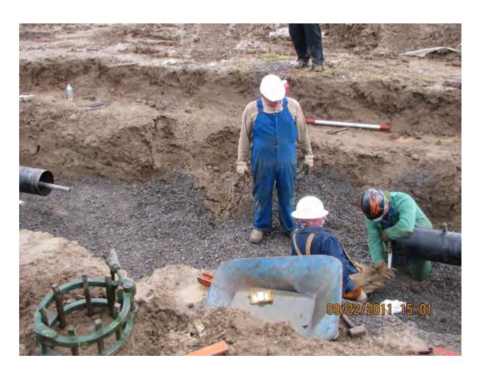
**Photo #5: Pipeline with the damaged section cut out.**
