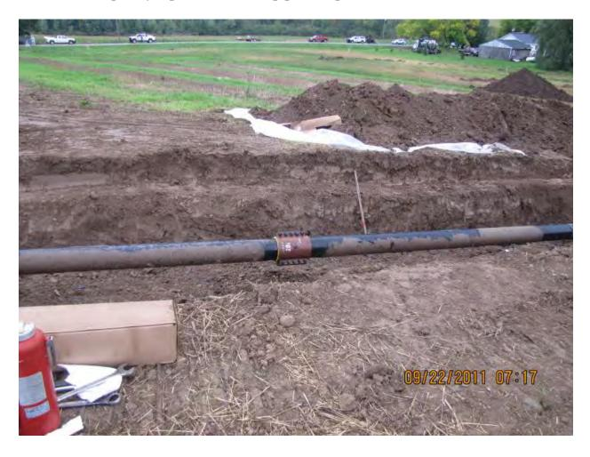
Photo #4: Temporary repair made to the pipe to stop the leak.
