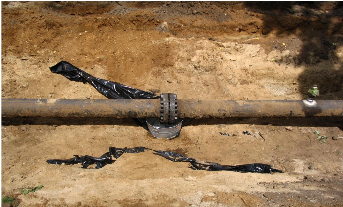
The Leaking Flange Excavated
