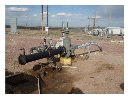
The end of line scraper receiver and associated valving.
