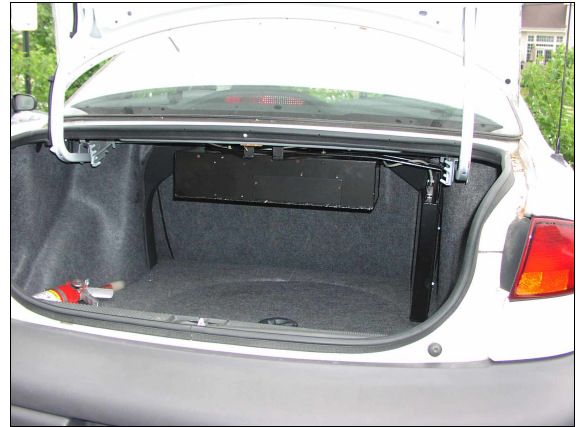
Figure 2. The main Data Acquisition System (DAS) unit mounted under the "package shelf" of the trunk.
