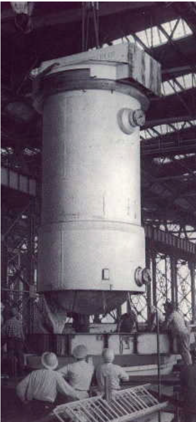
Figure 7-2 Reactor Vessel during Fabrication
