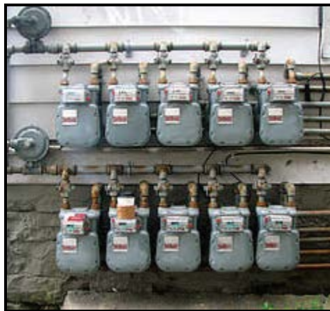
Figure 12 - Service through a Meter Manifold
