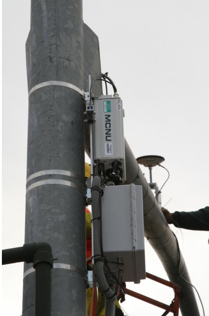
Figure 6: RSE Installation at the First California Intersection
