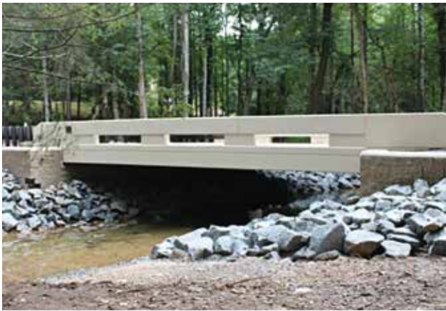
FHWA's bridge replacement research has reduced construction times, decreasing congestion and increasing the mobility of goods and passenger travel. (Image source: FHWA)
