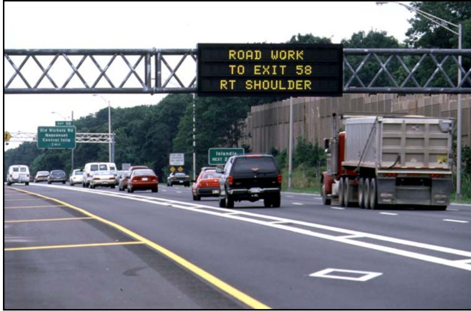
Figure 4-4 CMS on a freeway.
