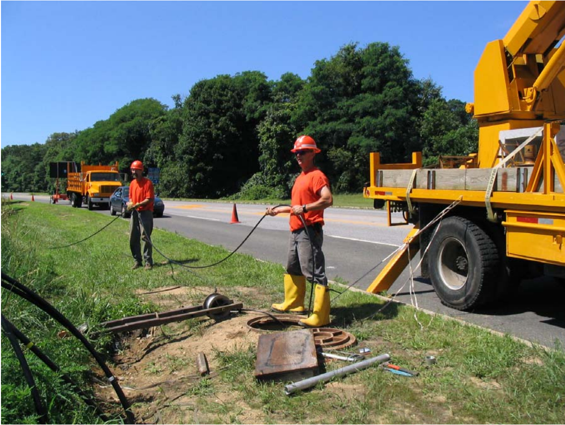
Figure 9-1 Installing communications cable.
