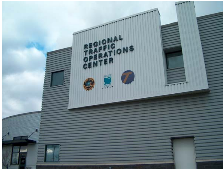
Figure 1-1 Rochester N.Y. Regional Traffic Operations Center.
