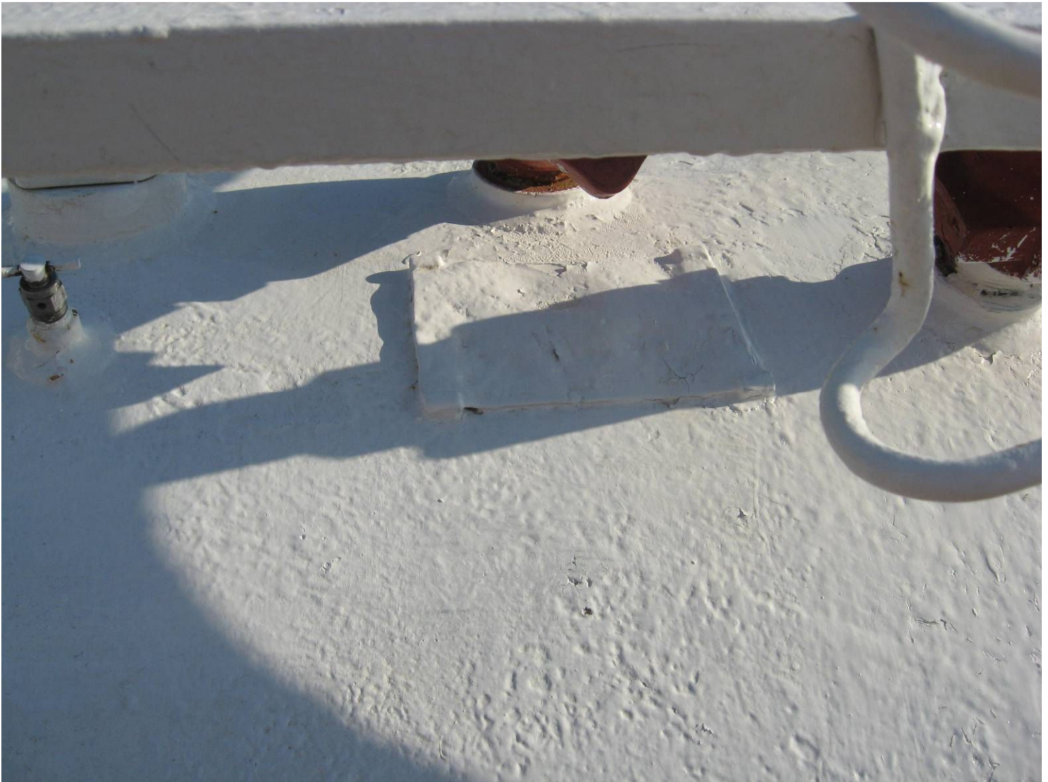
#G34 illegible ASME data plate
