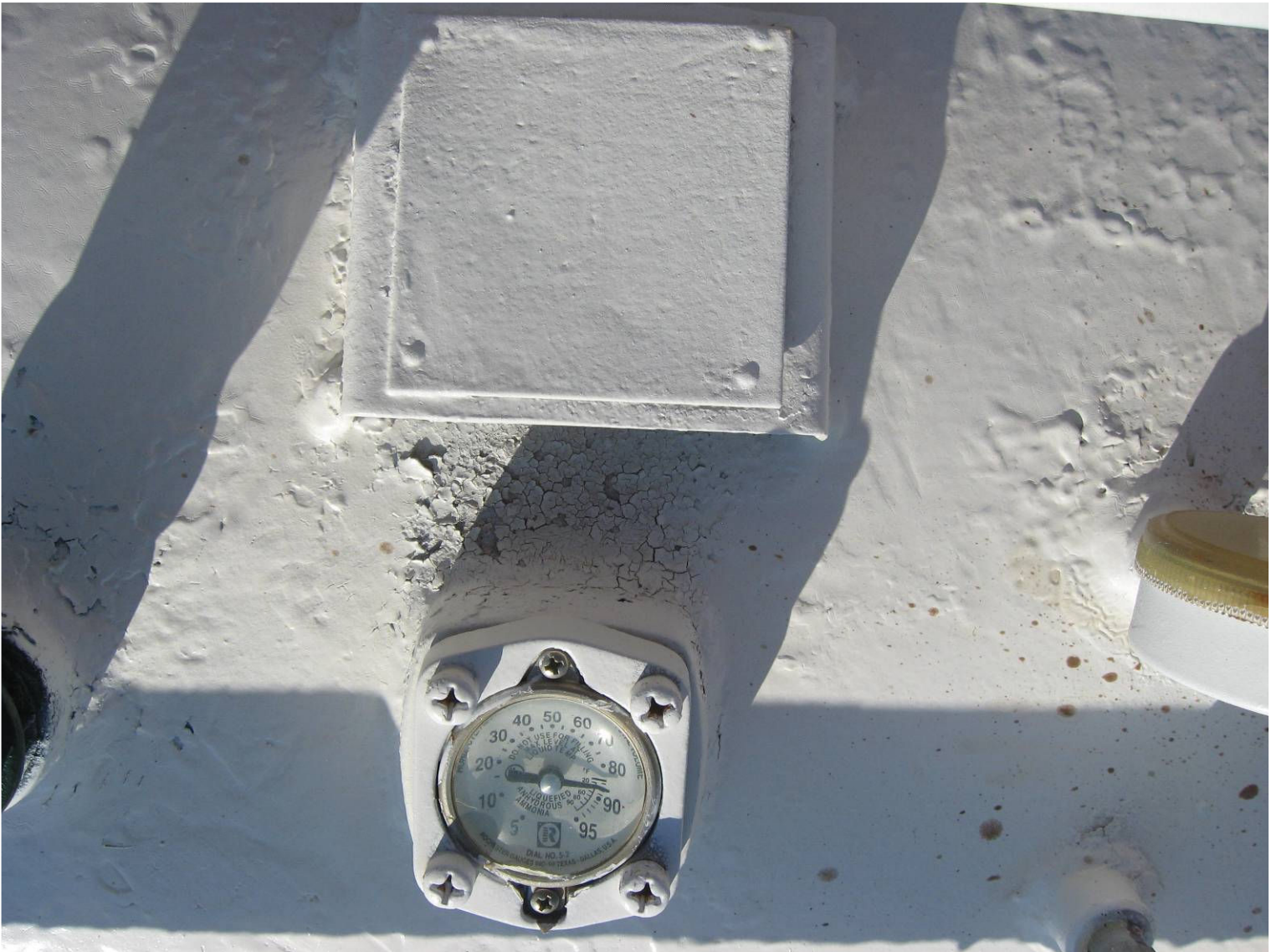
#53 with illegible ASME data plate
