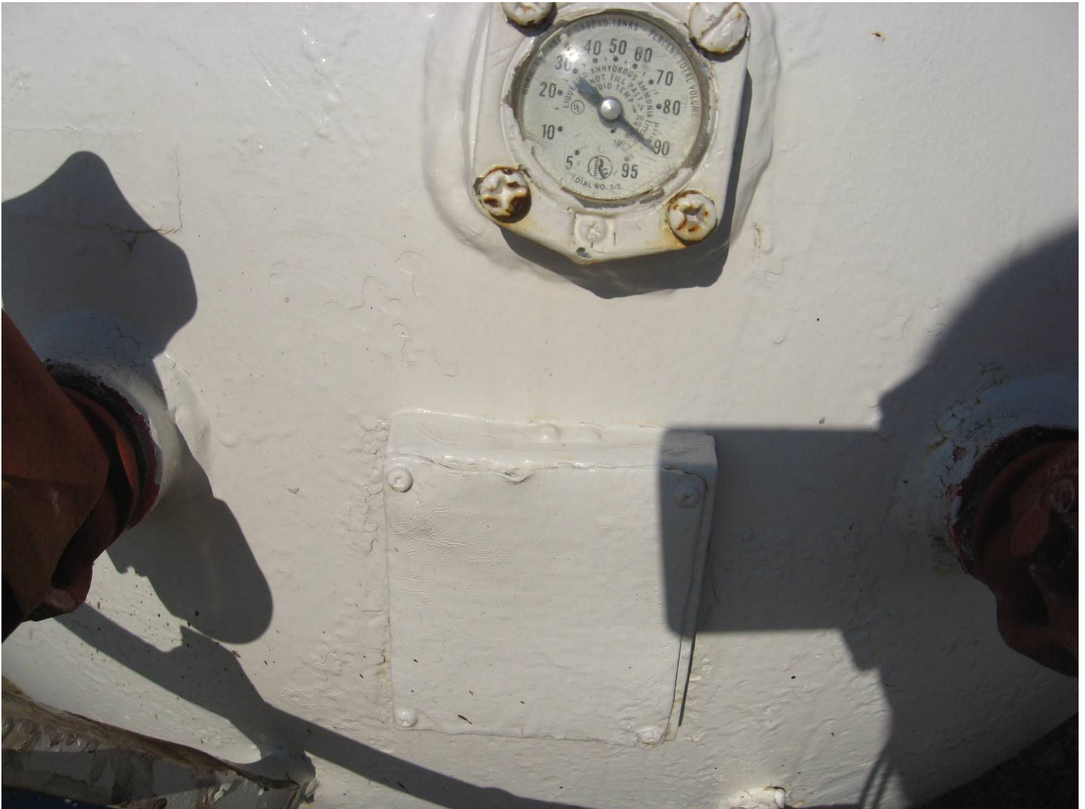
#60 with illegible ASME data plate
