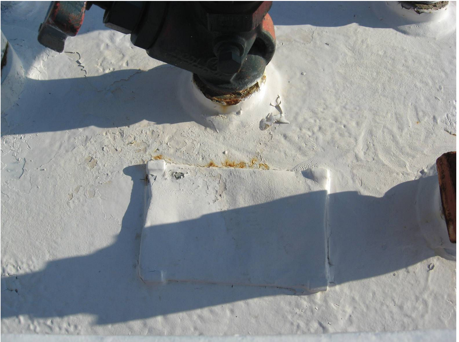
#71 illegible ASME data plate
