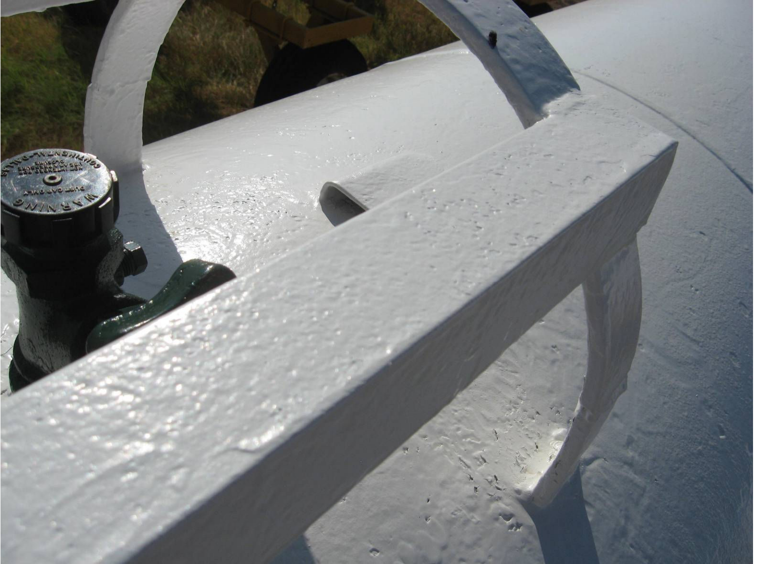
#G9 with illegible ASME data plate
