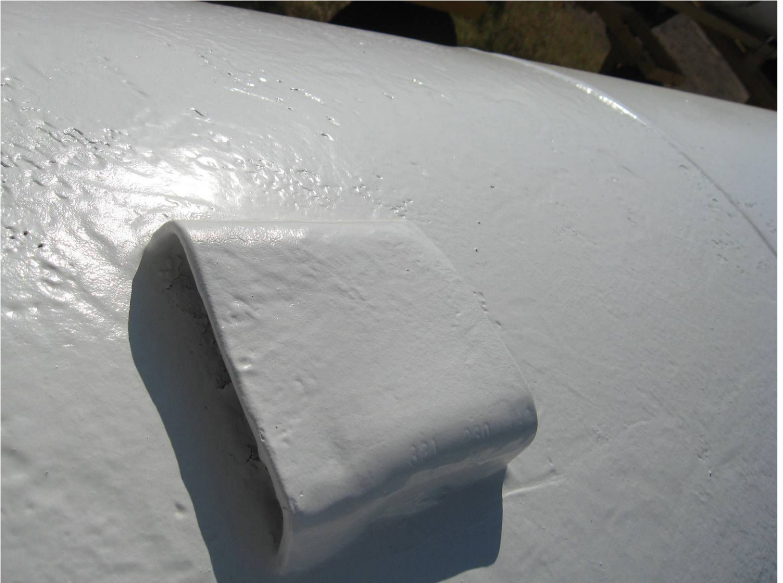
#G9 with illegible ASME data plate
