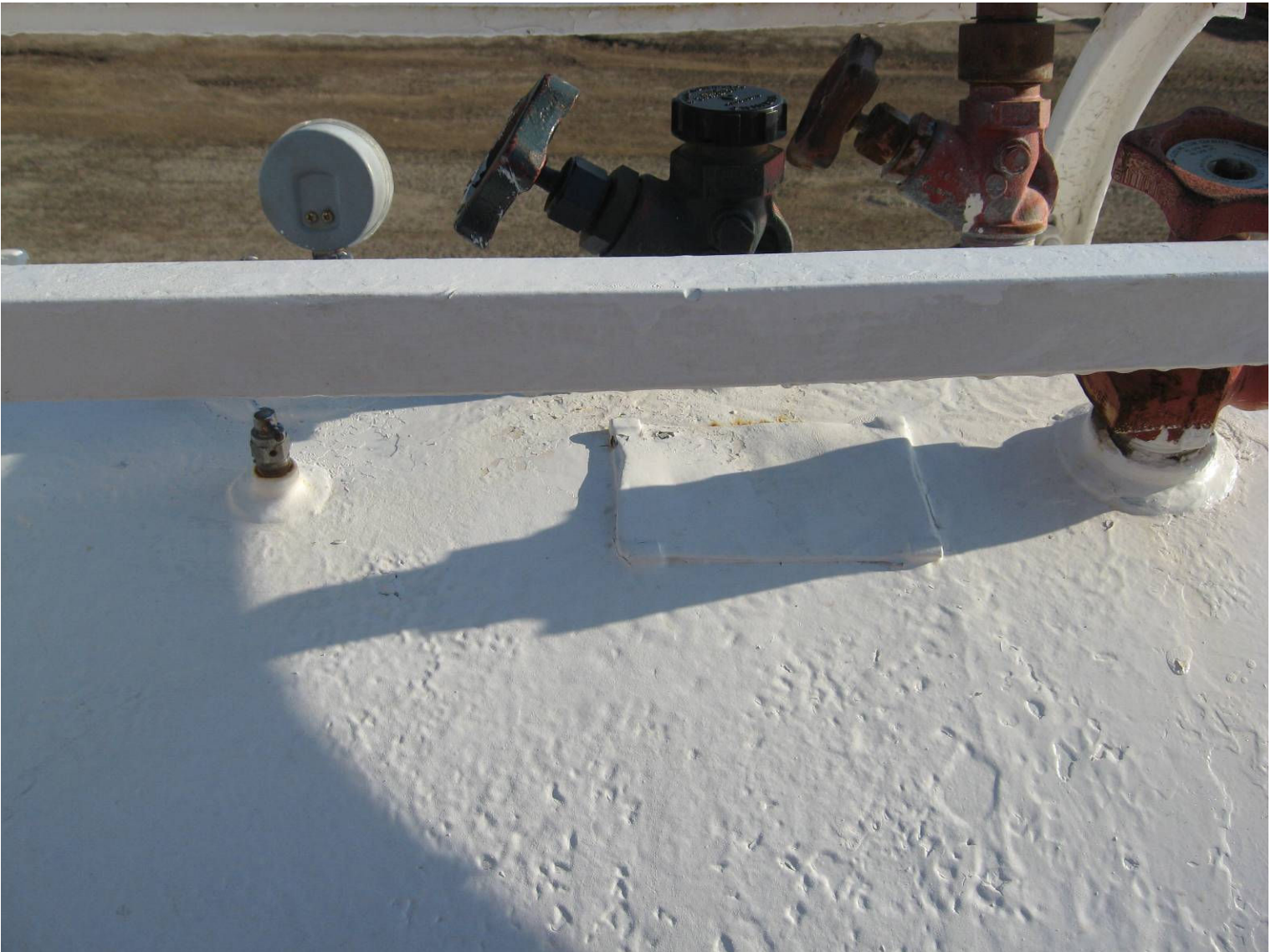
#71 illegible ASME data plate
