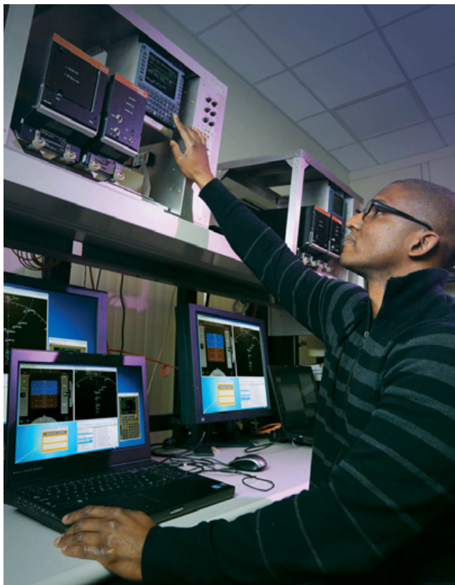
Testing in the Data Comm laboratory at the FAA's William J. Hughes Technical Center. Photo: FAA
