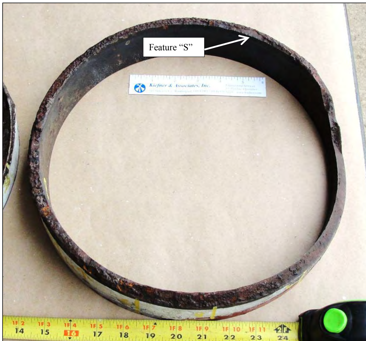
Figure 21. Fracture surface of Pipe 014
