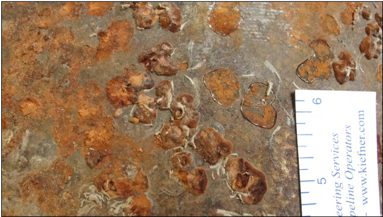
Figure 9. Corrosion under biotic mass
