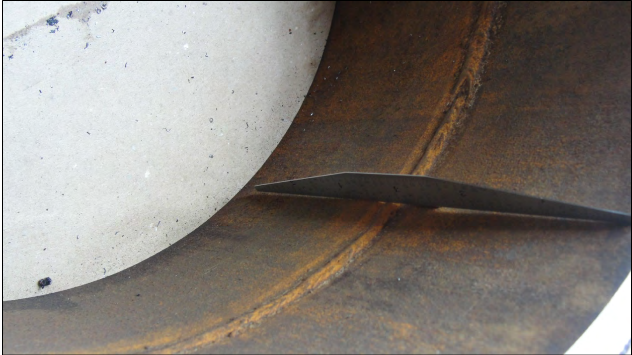
Figure 18. Fit-up Across Weld 030
