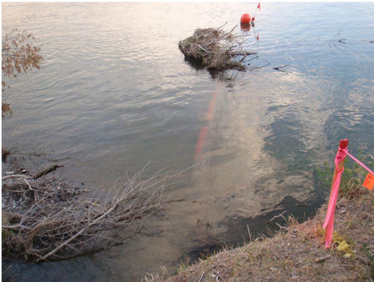
Picture taken on Thursday, September 29, 2011, 2:56:30 PM. Close up of the pipe from the south bank. Buoy is marking the north end of the rupture from the south bank pipe.
