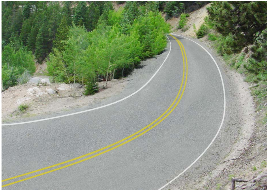
Figure III-16 Station 37+700 Chip Seal Surface
