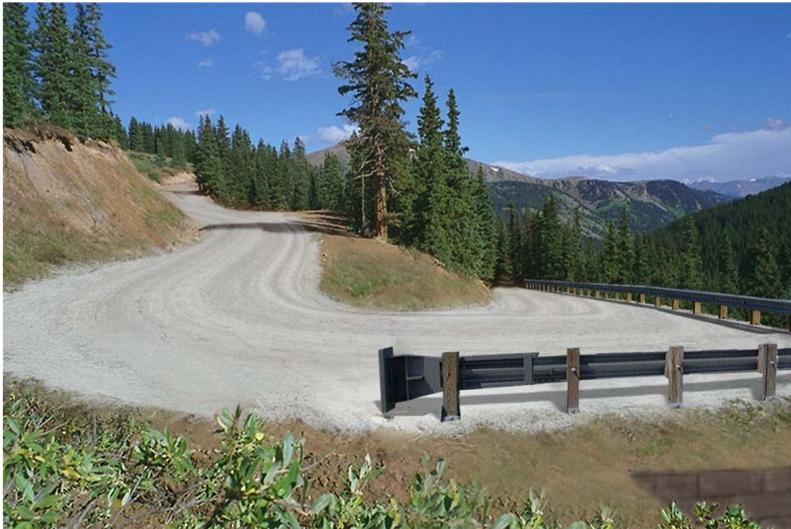
Figure III-12 Station 22+900 Light Reconstruction, Macadam Surface Second Switchback North of Guanella Pass Summit
