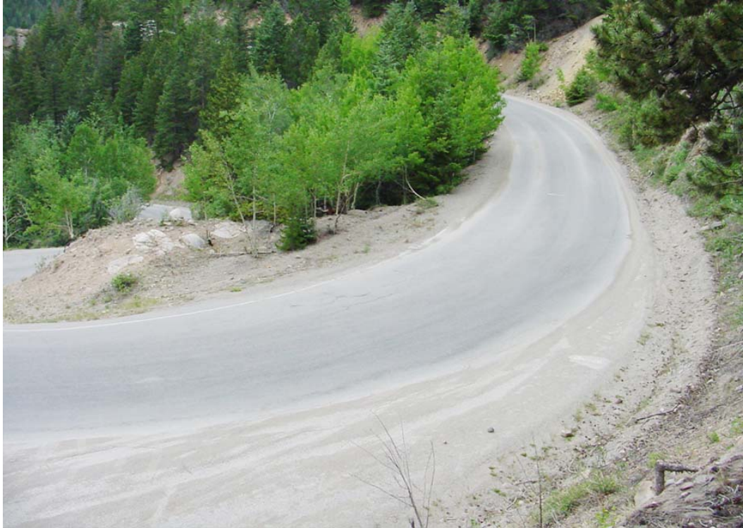
Figure III-16 Station 37+700 Chip Seal Surface
