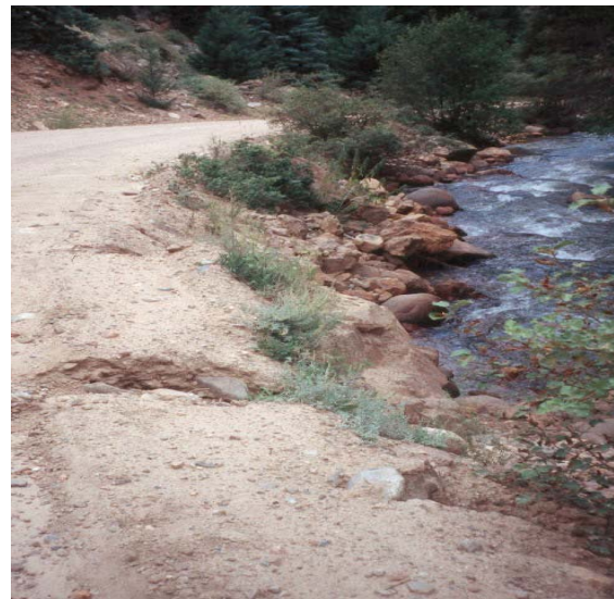
Figure III-5d: Area of Guanella Pass Road where the roadbed erodes directly into Geneva Creek.
