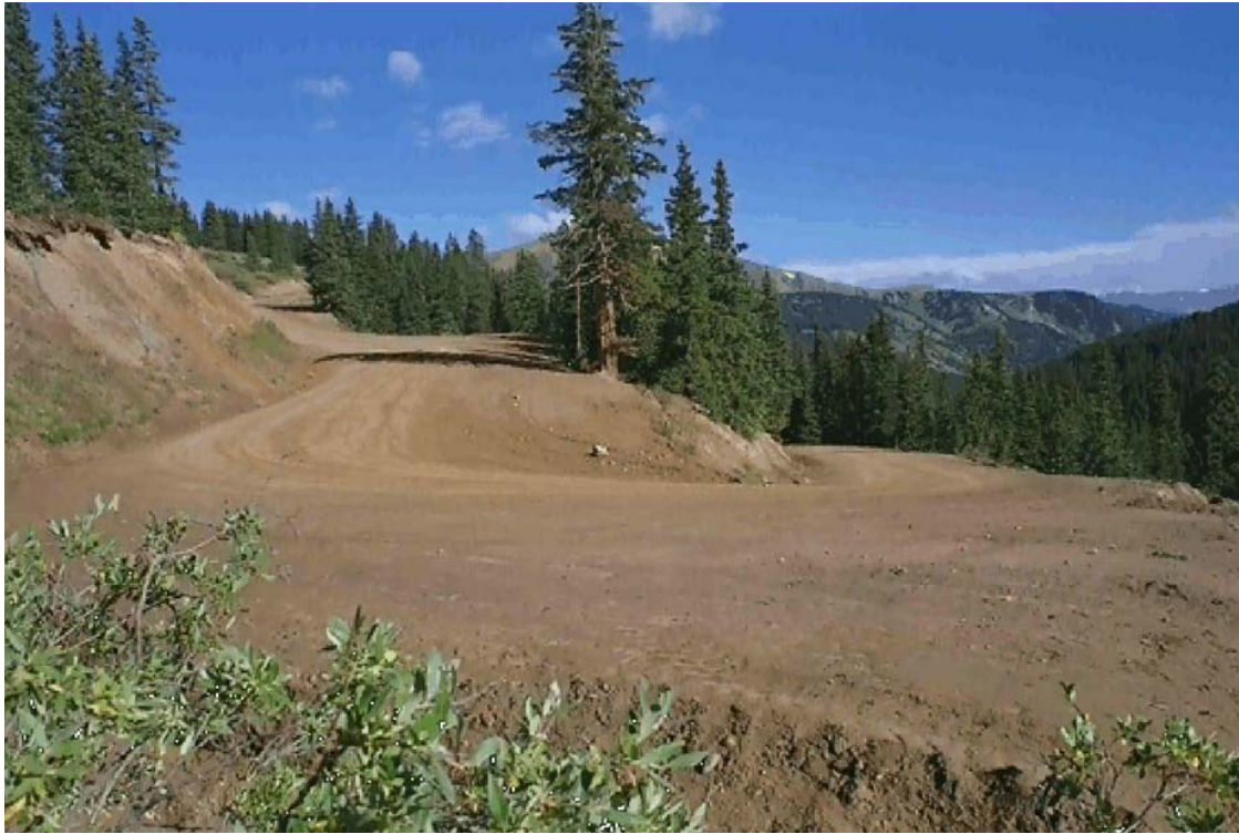
Figure III-12 Station 22+900 Light Reconstruction, Macadam Surface Second Switchback North of Guanella Pass Summit
