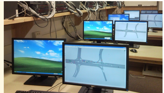
Pictured is NIATT's Controller Interface Device, which is used to test traffic control strategies. Photo courtesy of NIATT/University of Idaho.
