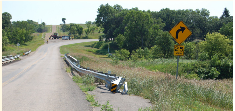
Rural road safety audits, following a blueprint developed in North Dakota, identify low-cost/high-value safety improvements for rural roads. Signage, sight-line impediments, pavement markings, and missing or damaged safety equipment are among the items considered. (Photo courtesy of Mountain-Plains Consortium)
