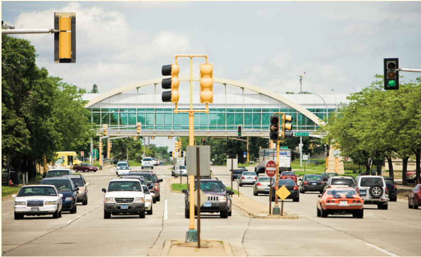
The SMART Signal system, installed on France Avenue in Edina, Minnesota, collects signal-phase change events. Photo courtesy of Jonathan Chapman.
