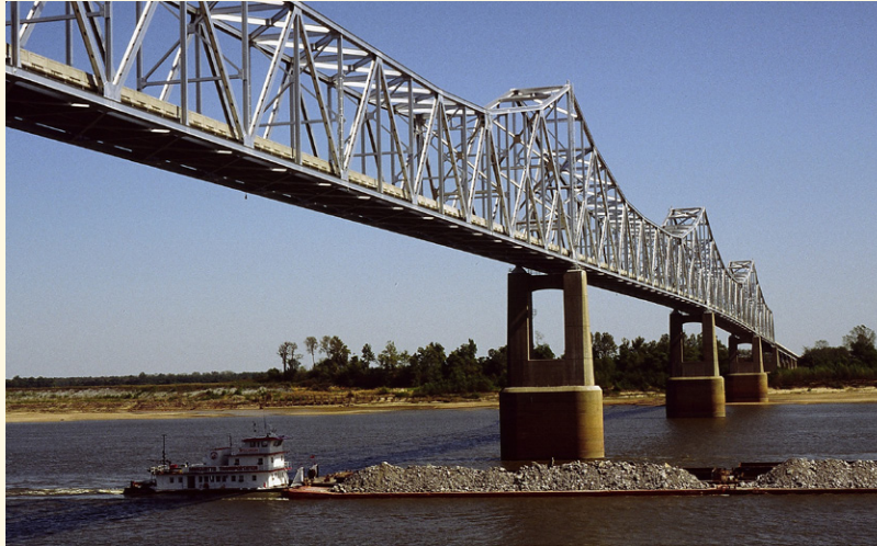
Pictured is the Mississippi River Bridge in Helena, Arkansas. Photo courtesy of the Arkansas State Highway and Transportation Department.
