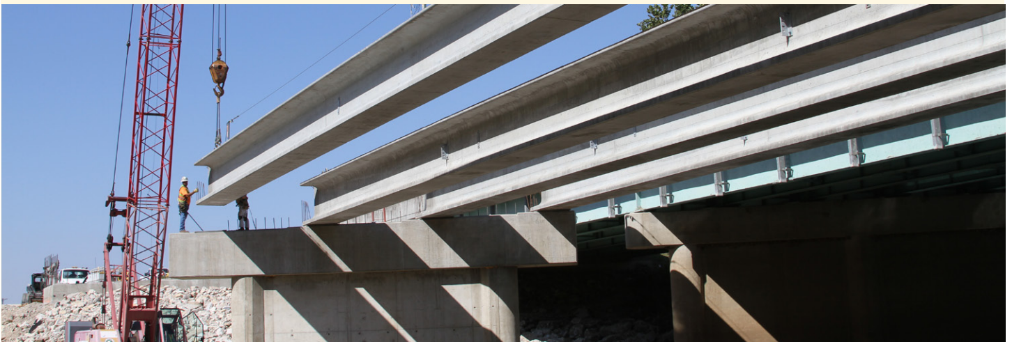
Missouri Bridge A7957 on Highway 50 near Jefferson City, Missouri during construction showing a high-strength self-consolidating concrete (HS-SCC) NU girder being erected with Data Acquisition System (DAS) attached. Photo courtesy of Dr. John J. Myers, Missouri S&T.
