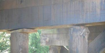
Figure 5. Insufficient Support for Bridge Components
