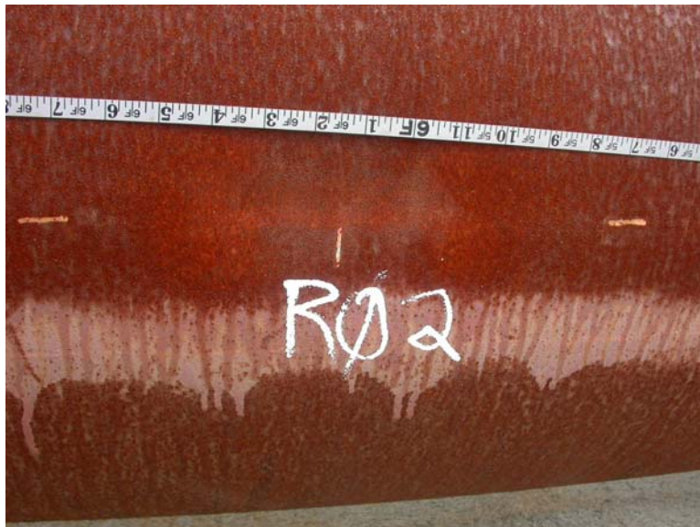
Figure 20. Example Mechanical Damage Defect from Pipe Sample 2
