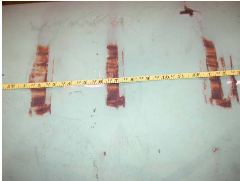
Figure 19. Example Mechanical Damage Defect from Pipe Sample 1
