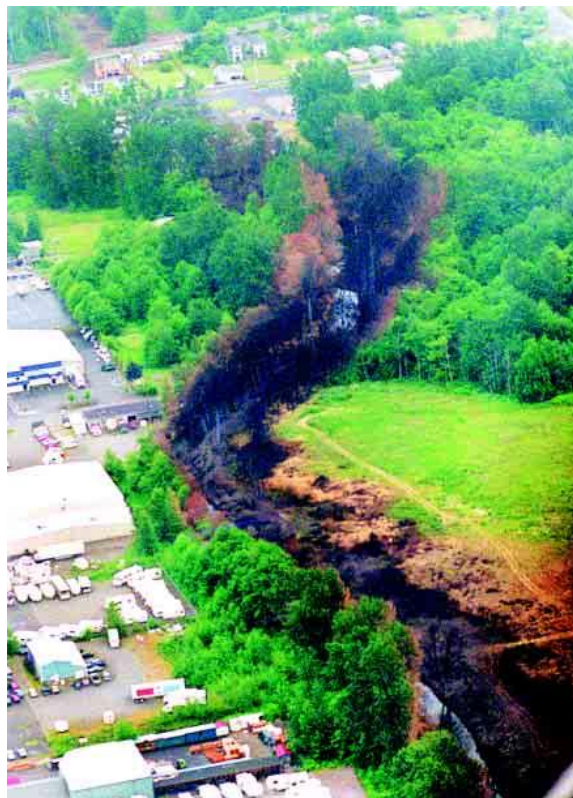
Fig. 1.3. Fire damage resulting from hazardous liquid pipeline release in Bellingham, Washington (NTSB, 2002).
