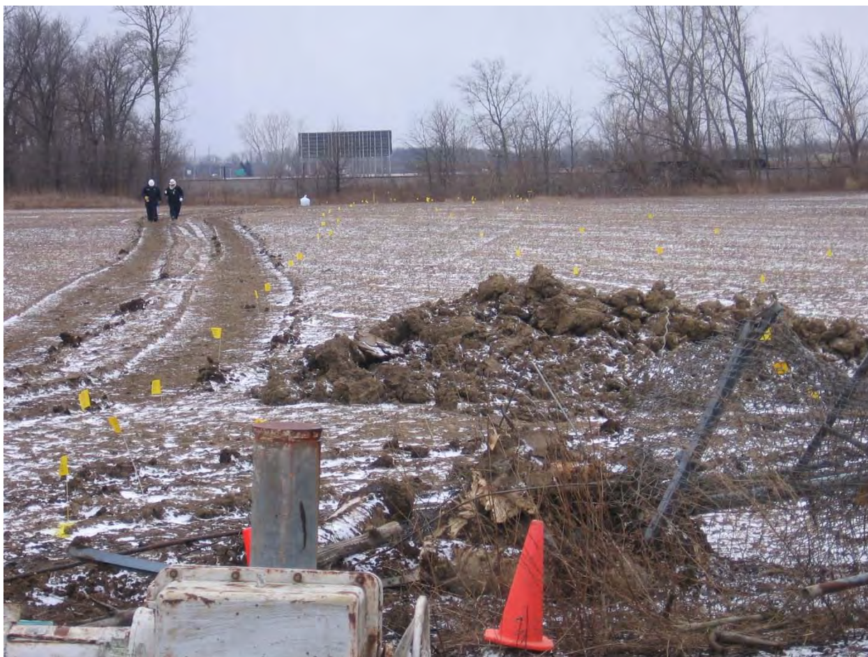
Photo 3 - The photo shows the view south of the branch connection. The tree line indicates Rocky Ford Creek. Field tile drain to the south into the Rocky Ford Creek and crude oil did reach the creek through the tile.
