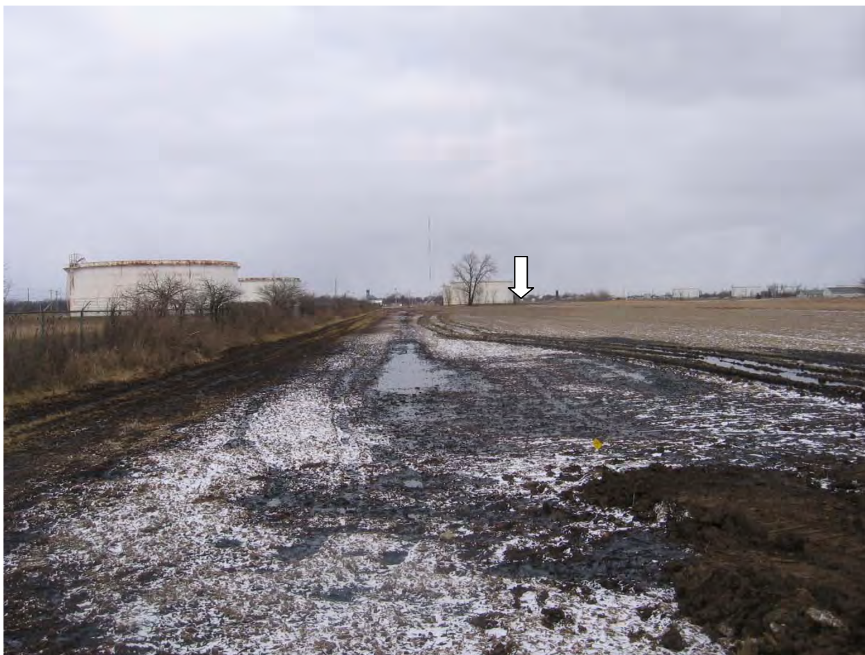
Photo 1 – View looking north from leak site. Tanks visible in the photo are no longer in service. The arrow points to Tank Farm Road.
