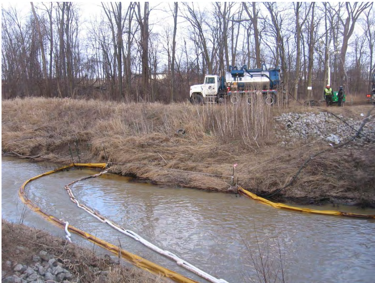
Photo 9 - The photo show booms in the Rocky Ford Creek just downstream of the Tank Farm Road.
