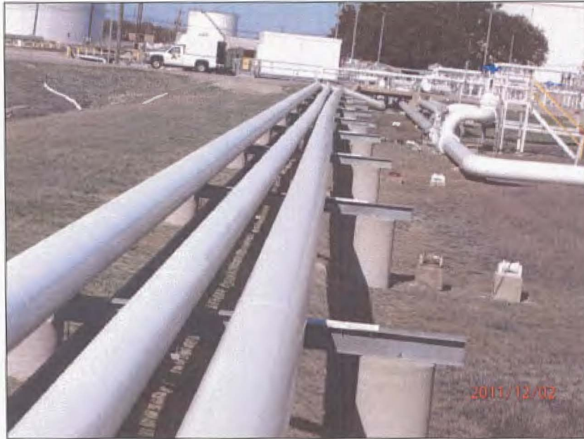
Picture 3 - Tank Line 3012 moved to the left – looking away from Tank 3012
