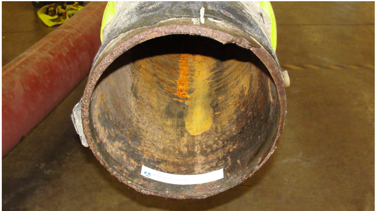
Figure 13. Fractured end of Pipe 014
