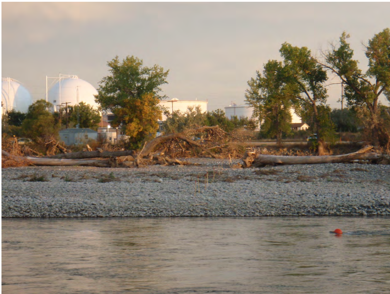
Looking north along original pipeline right-of-way alignment from the south bank taken Thursday, September 29, 2011, 2:55:19 PM. One can see the pipeline marked with lath and ribbon across the island and the first buoy to the south from the island that marks the pipe location being deflected downstream.
