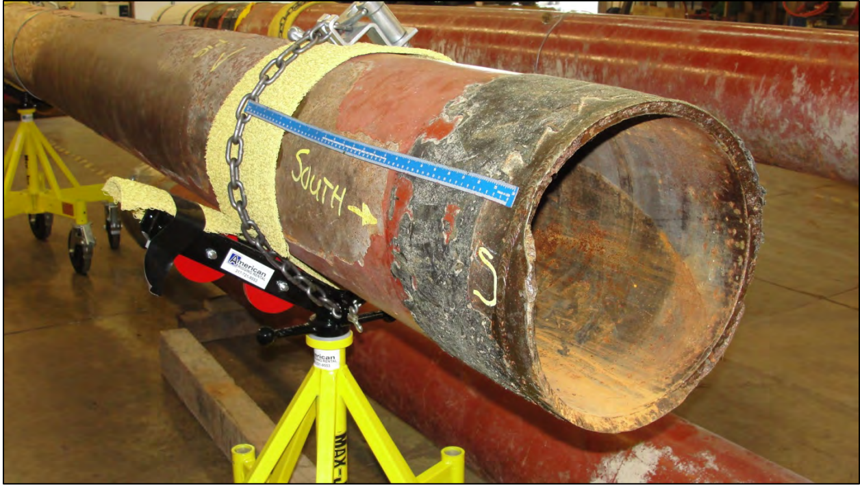
Figure 12. Fractured end of Pipe 024
