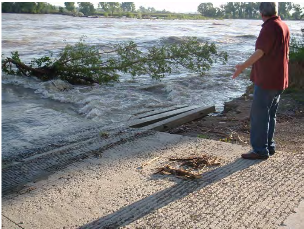
Looking NE from south bank of the Yellowstone River at the boat ramp just upstream of the EMCO crossing. Picture was taken Thursday, July 07, 2011, 9:24:08 AM 6 days after line rupture. The man is showing the location of the water on the south bank the day before. Notice the island is not visible. Also notice the debris pile in the river.
