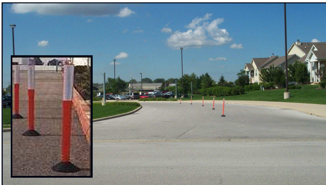
Figure 4. Flexible Delineators Channel Traffic into Lanes to Ensure Accurate In/Out Counts. 7
