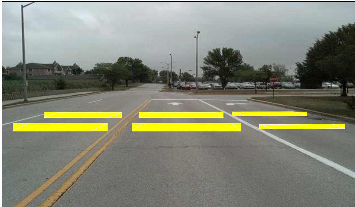
Figure 3. Example of Loop Detector Placement. 6
