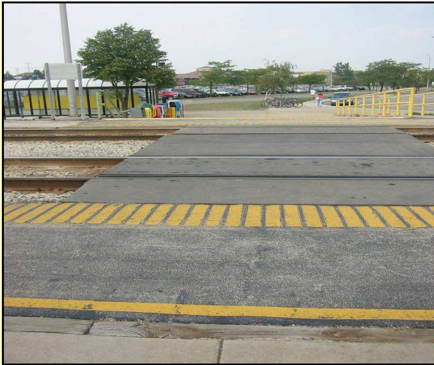
Figure 7. Both Stations have an At-Grade Pedestrian Crossing.
