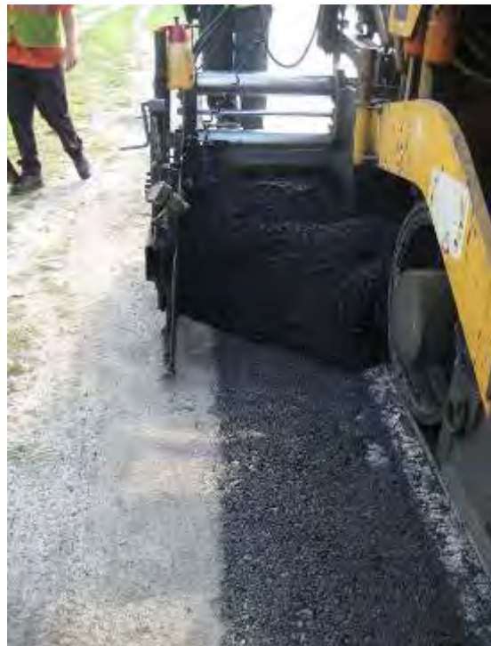
Figure 15. Equipment used to place the WMA overlay.
