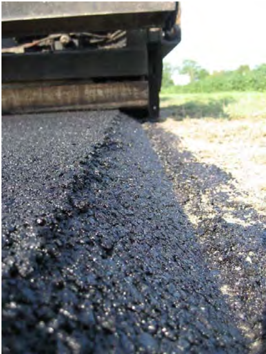
Figure 15. Equipment used to place the WMA overlay.
