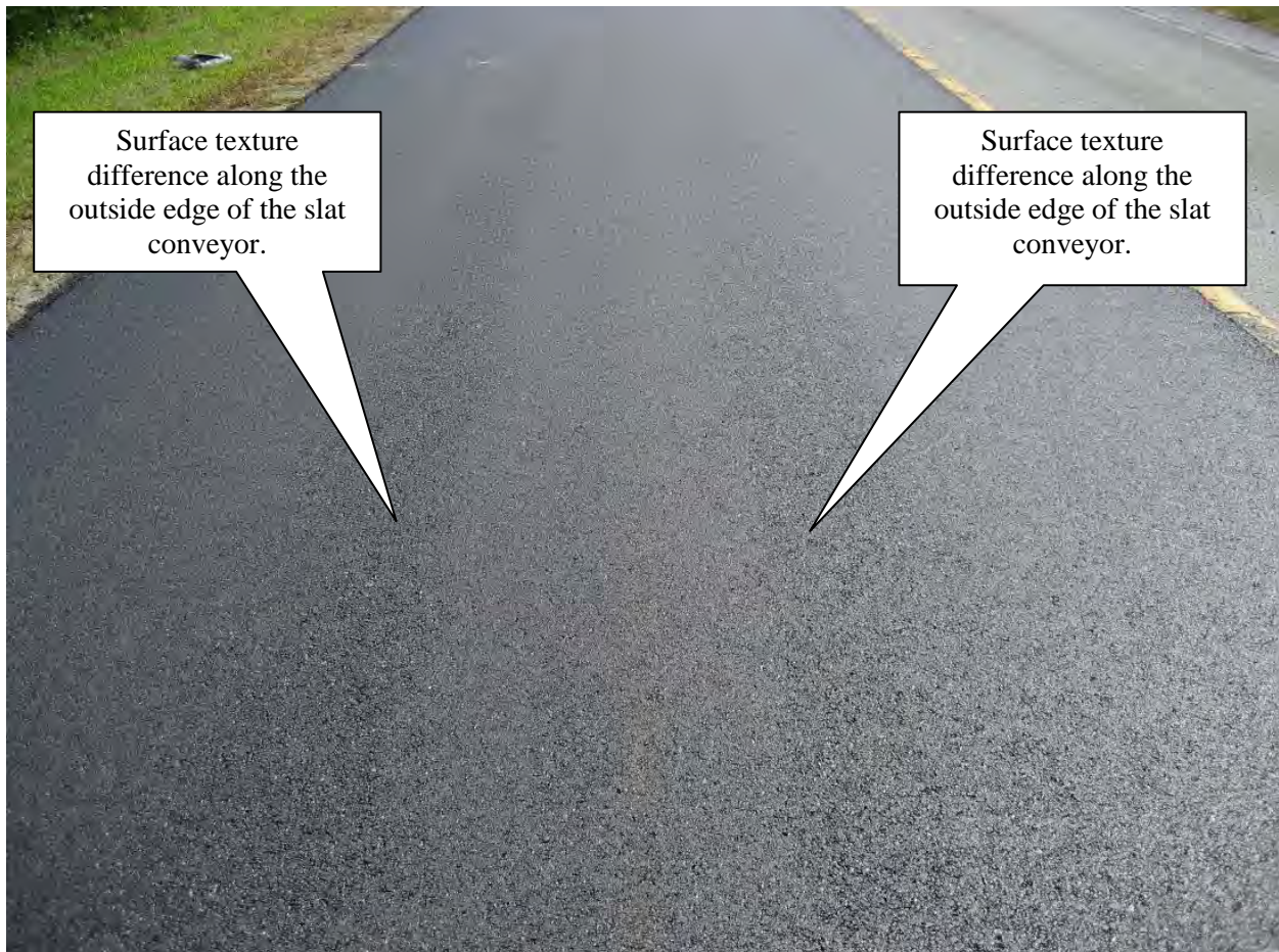
Figure 23. Longitudinal segregation or surface texture differences along the edge of both slat conveyors.
