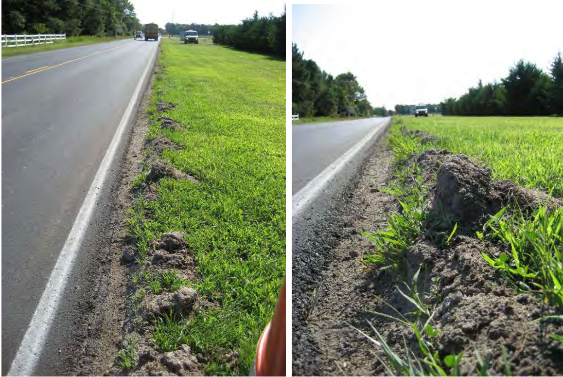
Figure 4. Edge of pavement graded in some areas to remove grass and debris.
