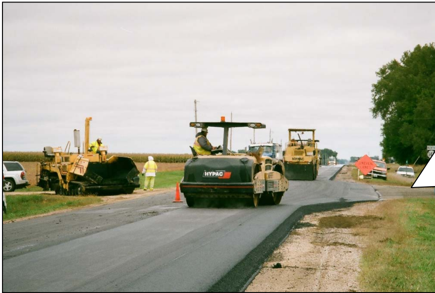
Figure 3. Placing an AC overlay at an intersection of a Safety Edge SM project.
