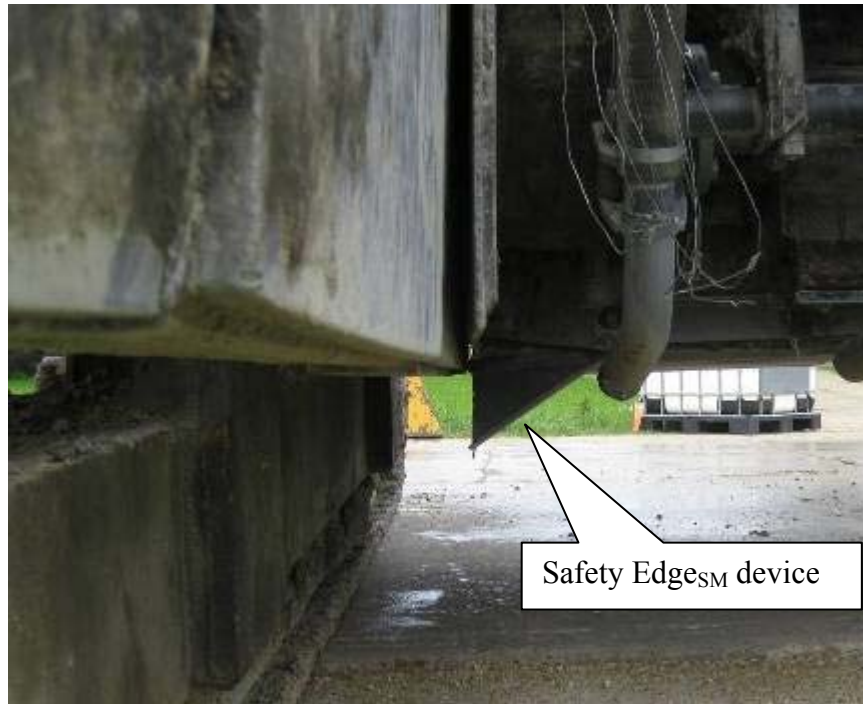
Figure 15. View of the Safety Edge SM device from front of paver.
