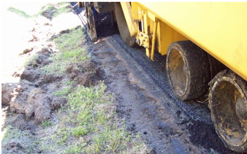
Figure 9. Paver positioned to align the Safety Edge SM break point over the existing pavement.
