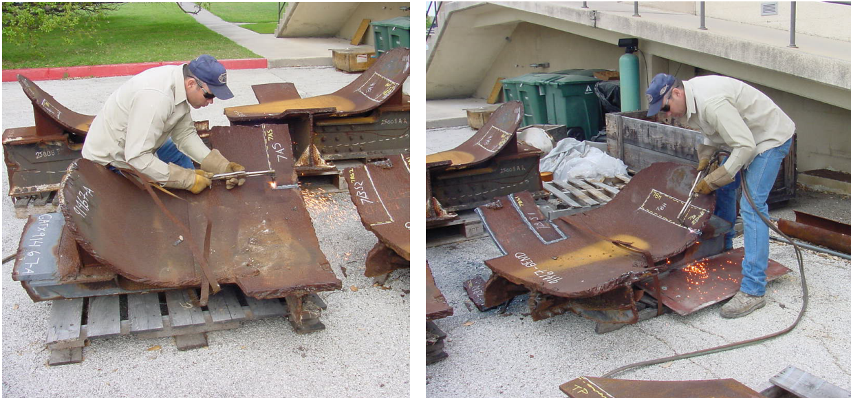
Figure 2-2. Torch-cutting removing segments from the tank cars.
