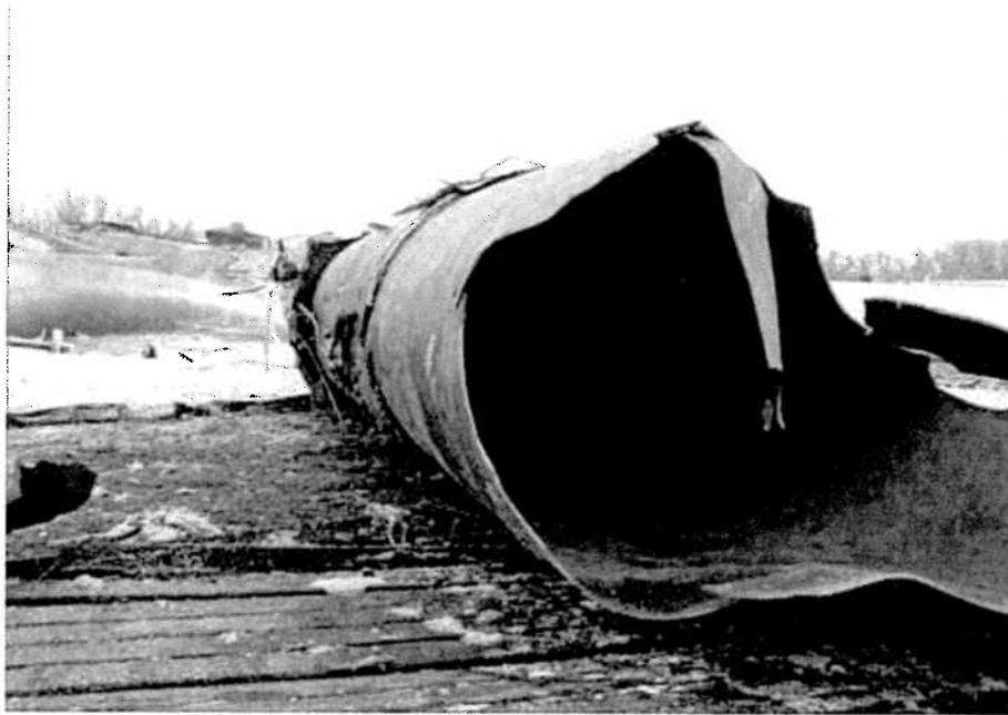
Figure 13. Photograph of B-end View of Tank Car PLMX 4504 at Minot Accident Site
