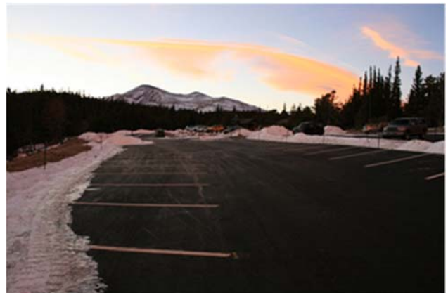
Figure 1-2. BLRA Entrance Portal parking lot (winter).
