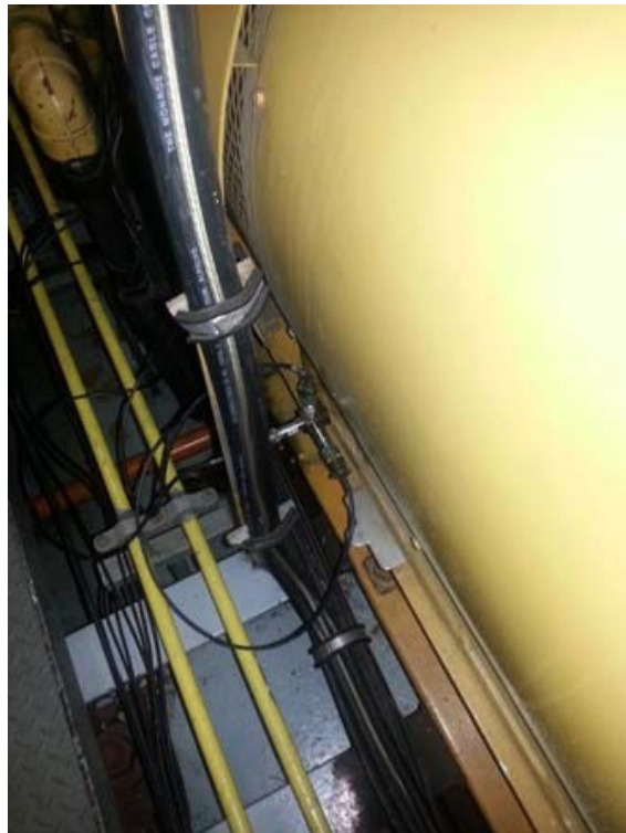
Figure 15. Generator Forward Accelerometers
