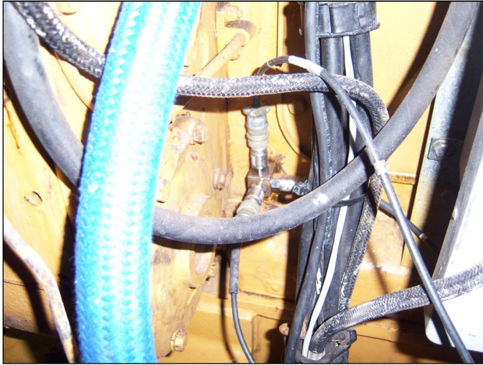
Main Diesel FWD BEARING
