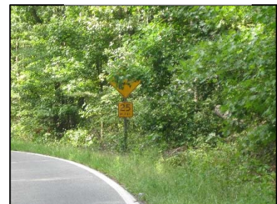
Figure 39. Photo. Curve warning sign covered by foliage.
