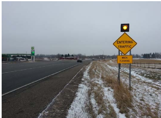
Figure 65. Photo. A dynamic warning sign alerts drivers in real time of other users in the roadway.
