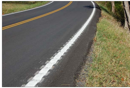
Figure 48. Photo. Milled Edge Line Rumble Stripes. Source: KYTC.
