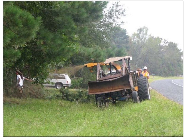
Figure 50. Photo. Removing brush as part of clear zone maintenance. Source: Texas DOT.
