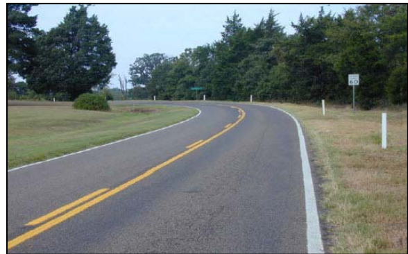
Figure 12. Photo. The color of delineators must match the color of the adjacent edge line. Source: Texas Transportation Institute.
