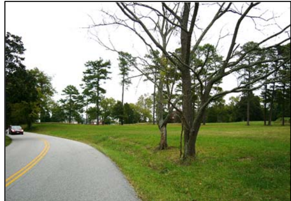
Figure 49. Photo. Fixed objects (trees) located within clear zone.
