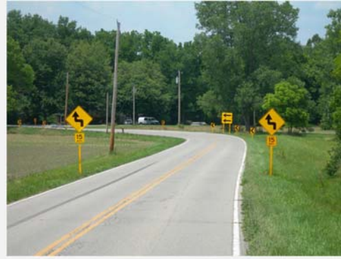
Figure 28. Photo. After signage updates.
