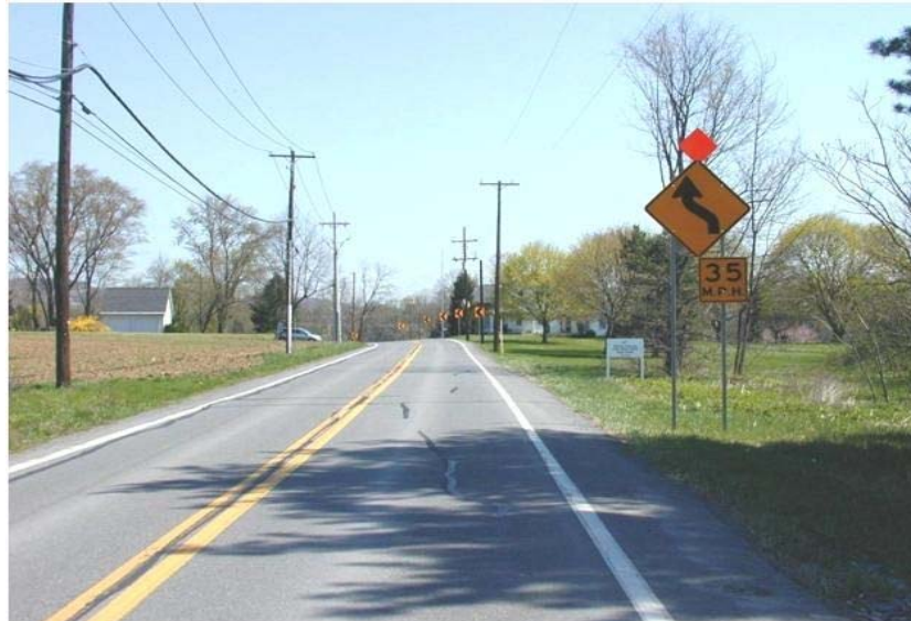
Figure A-1. Photo. An orange flag supplementing the reverse curve warning sign and speed advisory plaque. Chevrons were also used to delineate the curve.
