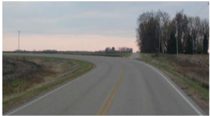
Figure B-1. Photo. Example of a visual trap; one of MnDOT's five risk factors for horizontal curves.
