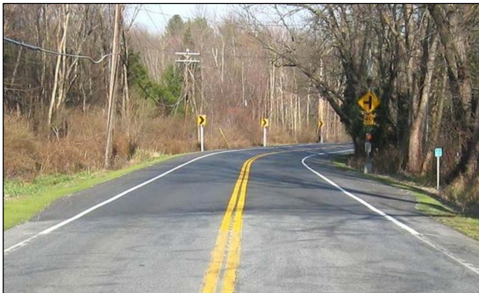
Figure 43. Photo. Widening on the inside and outside of the curve.
