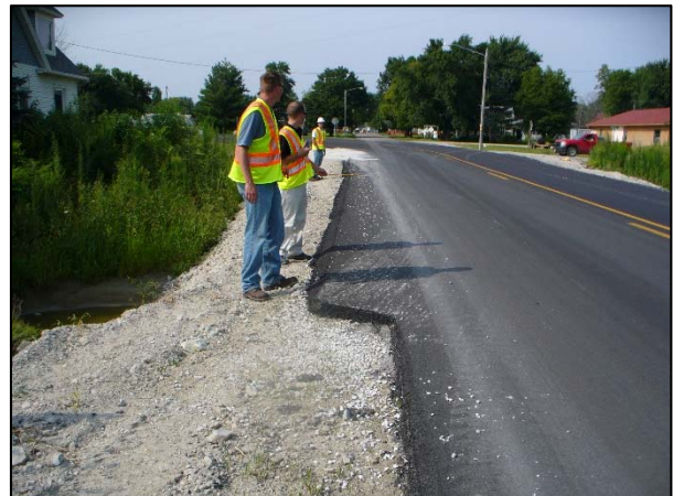
Figure 44. Photo. Shoulder paving operation.
