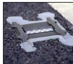
Figure 17. Photo. Snowplowable Retroreflective raised pavement marker.
