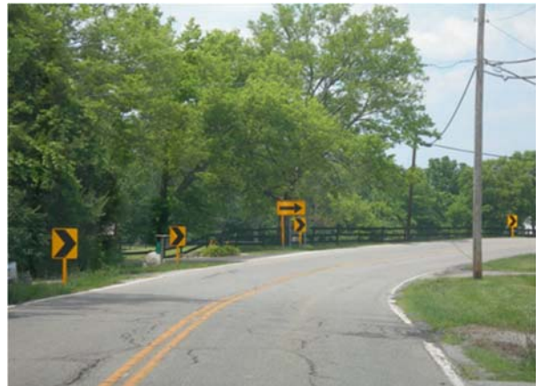
Figure D-4. Photo. A curve on a rural, two-lane road after signage updates through the Horizontal Curve Program.
