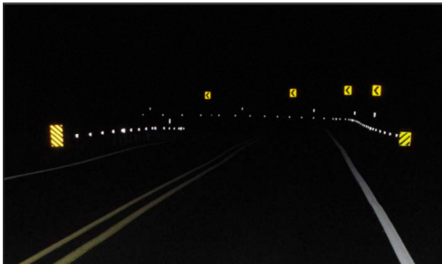
Figure 56. Photo. Delineators installed on post, nighttime view. Source: Michigan DOT.
