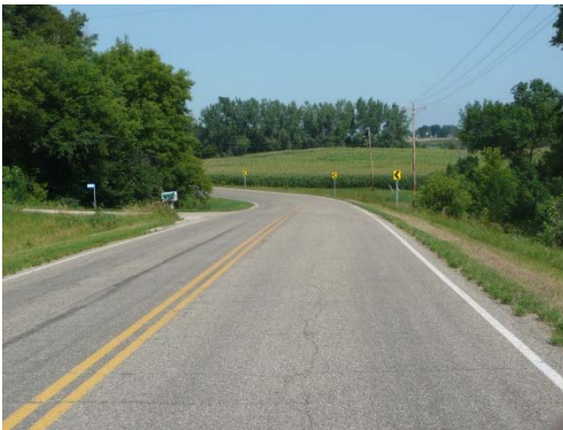
Figure 4. Photo. Delineation with chevrons. Source: MnDOT.
