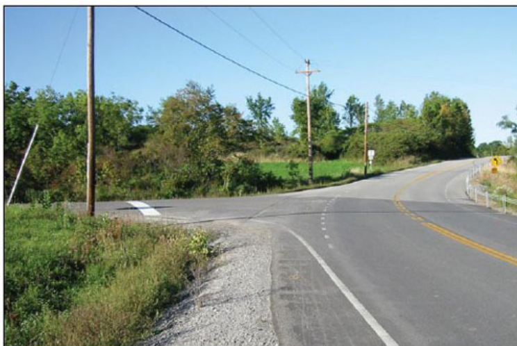
Figure 59. Photo. Dotted edge line extensions at an intersection within a curve.
