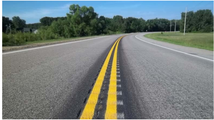
Figure 5. Photo. Centerline rumble strips.
