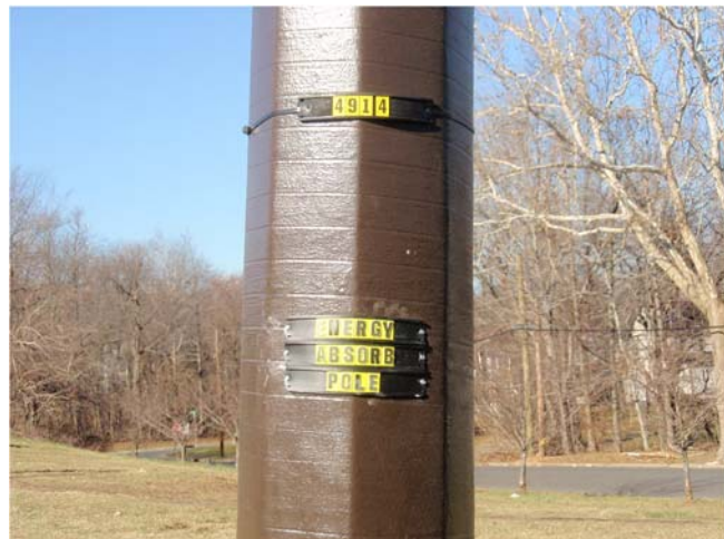
Figure H-1. Photo. A close-up of the energy absorbing utility poles used as a part of NJDOT's pilot project.
