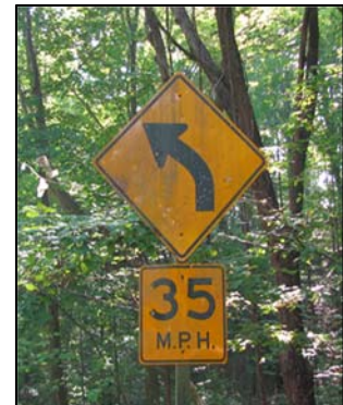
Figure 38. Photo. Low Retroreflectivity sign example.
