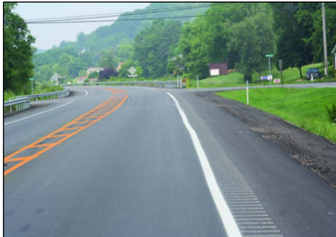
Figure 60. Photo. Pavement markings narrow the travel lane as the driver approaches the intersection.
