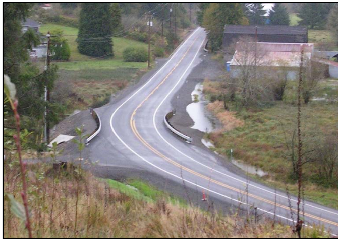
Figure 67. Photo. Intersection with paved approach.
