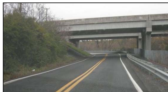
Figure 9. Photo. Edge lines.
