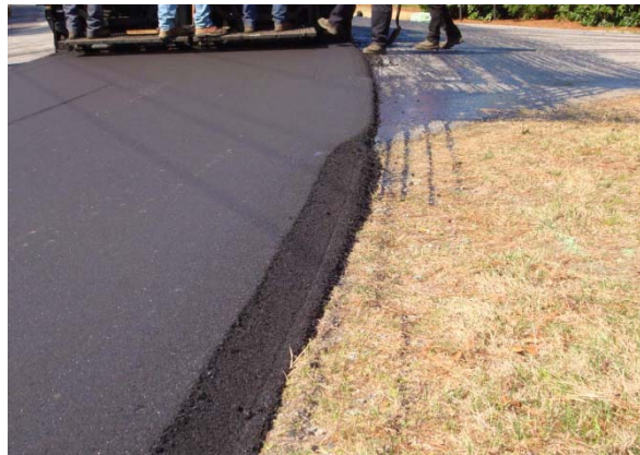
Figure 45. Photo. Pavement with and without the Safety Edge SM .
