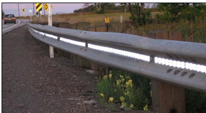
Figure 54. Photo. Retroreflective panels in the web of a W-beam. Source: Michigan DOT.
