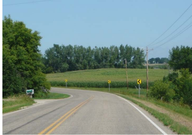
Figure B-2. Photo. MnDOT installed chevrons as part of their Systemic Safety Improvements Program.
