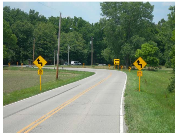
Figure D-2. Photo. A curve on a rural, two-lane road after signage updates through the Horizontal Curve Program.
