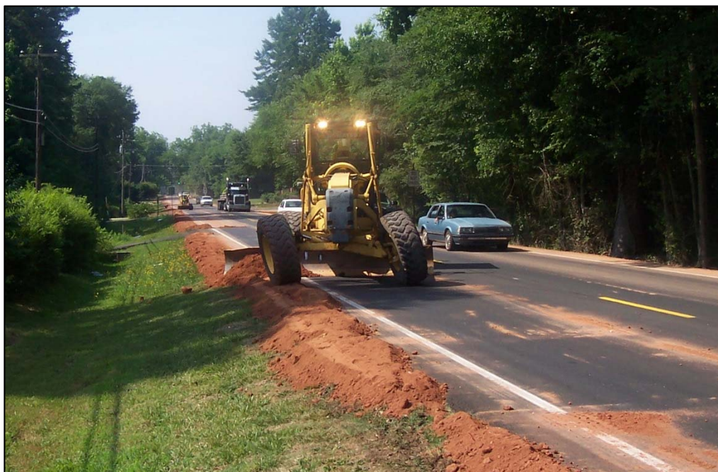
Figure 46. Photo. Backfilling against newly installed Safety Edge SM .
