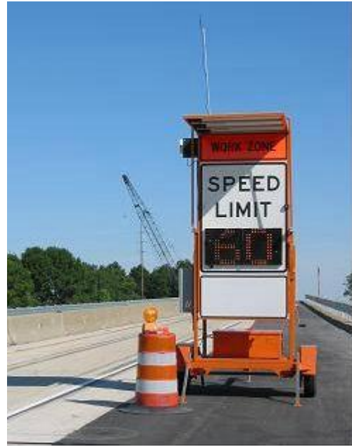
Figure 1. Variable speed limit system deployed in Michigan varied the speed limit based on nature of road work activity and traffic conditions.
