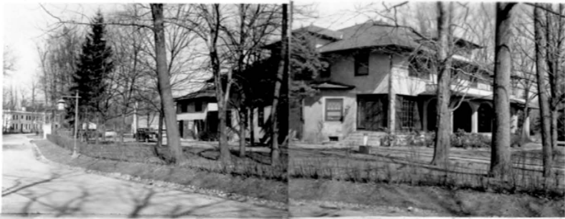
Figure 21. Panoramic View of the Marchant house and garage (both demolished), 1942 (NARA RG 178).
