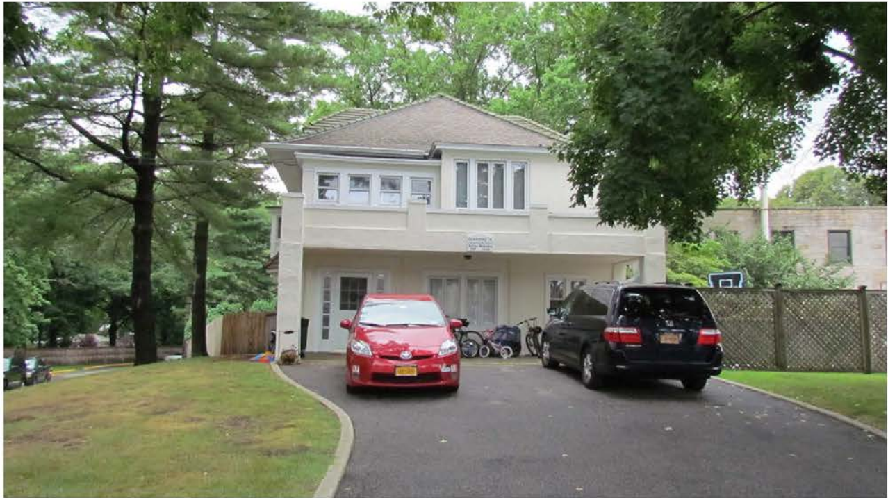
Photo 23. View to the south of Quarters K (Meighan House Garage).
