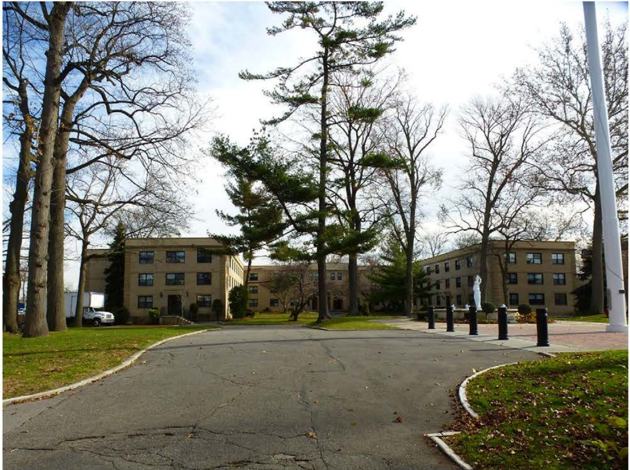
Photo 2. Looking east to Jones Hall (left), Truxton Arcade (center), and Barry Hall (right).
