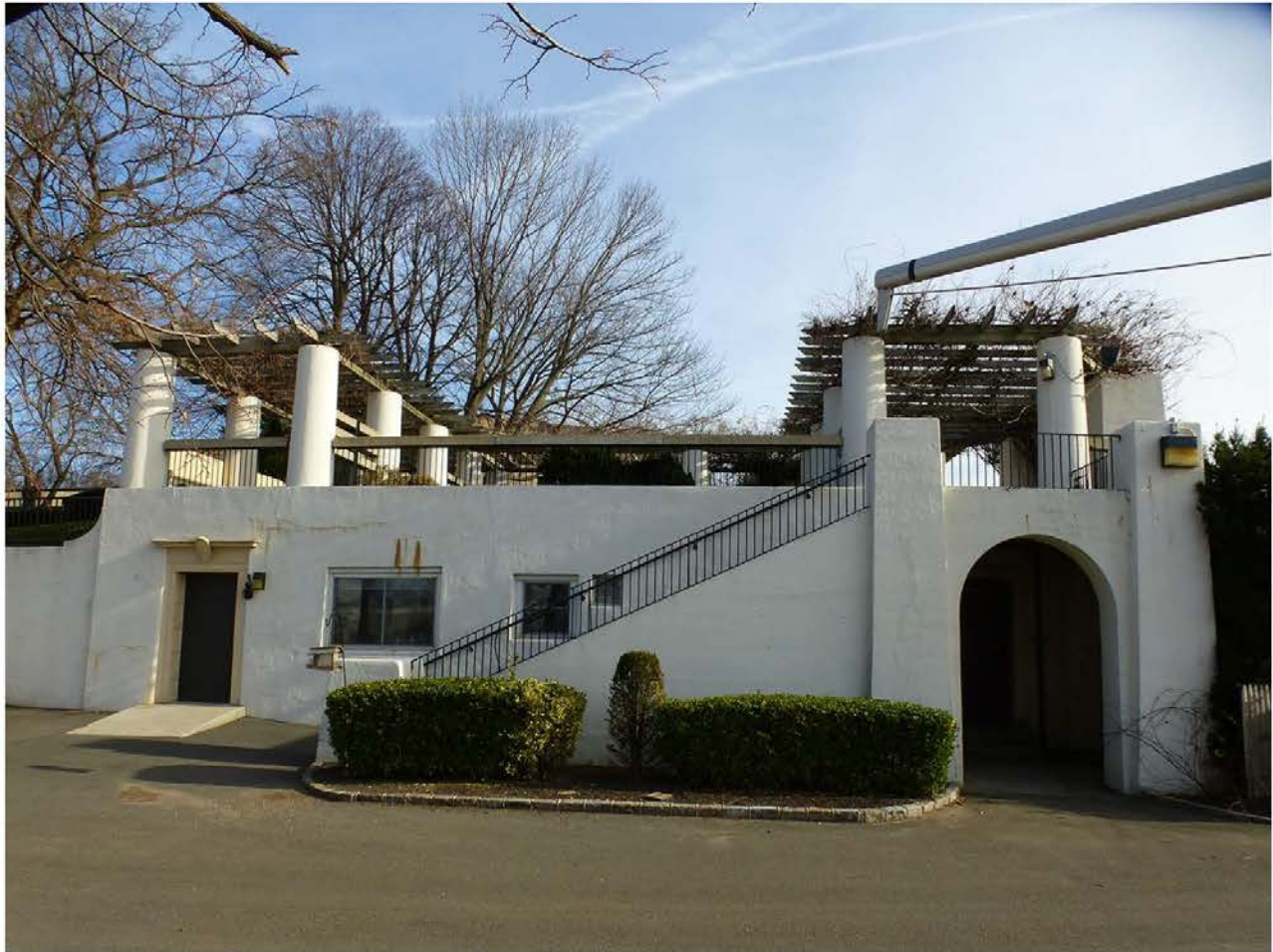
Photo 17. View to the east of the mechanical room for the Eldridge Pool.
