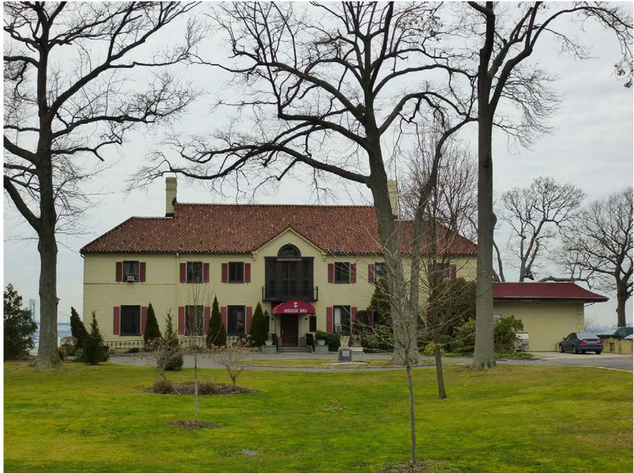
Photo 22. View to the west of Melville Hall (Meighan House).
