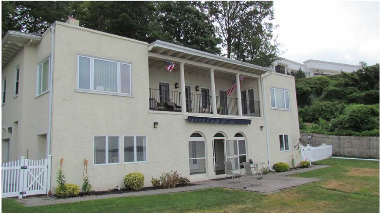
Photo 19. View to the east of Quarters D (Grenwolde Casino).
