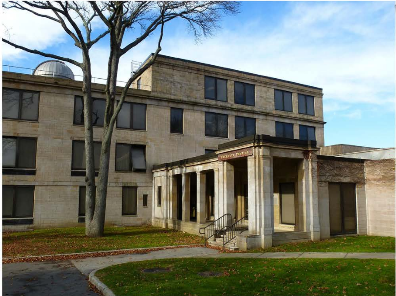
Photo 34. View to the northwest of Fulton Hall (a typical classroom building).
