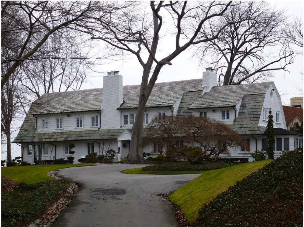
Photo 20. View to the northwest of Quarters A (Neiley House).
