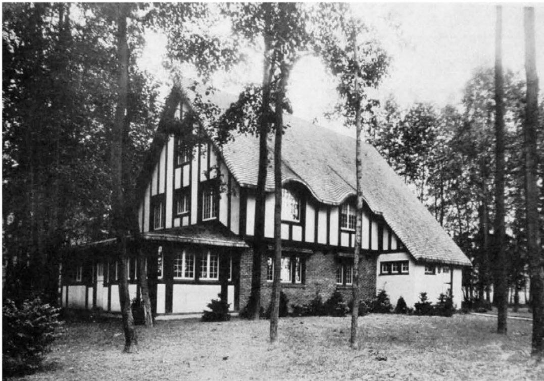
Figure 22. Vreeland (Friedman) house (Quarters C) in 1914 ( Architectural Record ).
