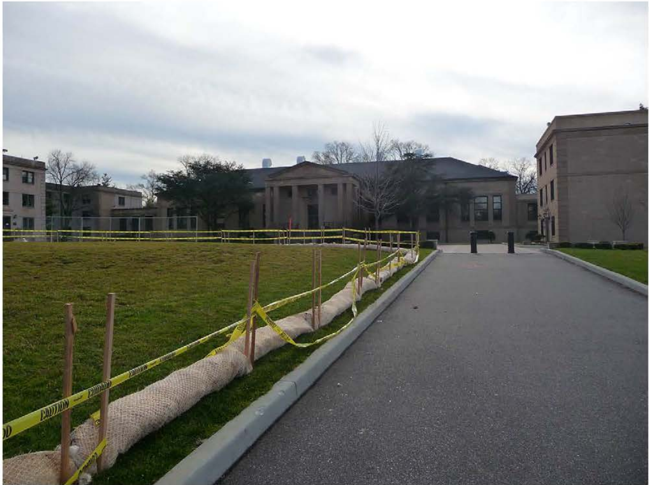
Photo 4. View to the south towards Delano Hall.
