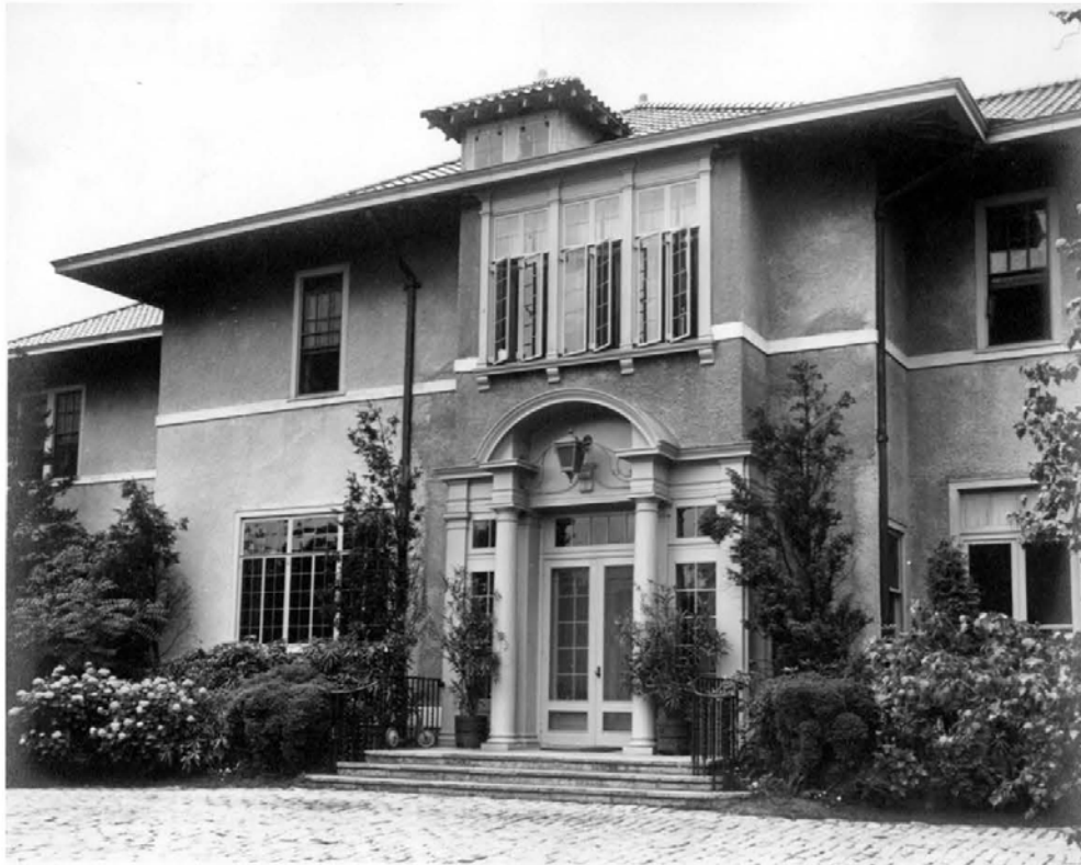
Figure 11. Schenck house (Land Hall), north façade, 1942 (NARA RG 178).
