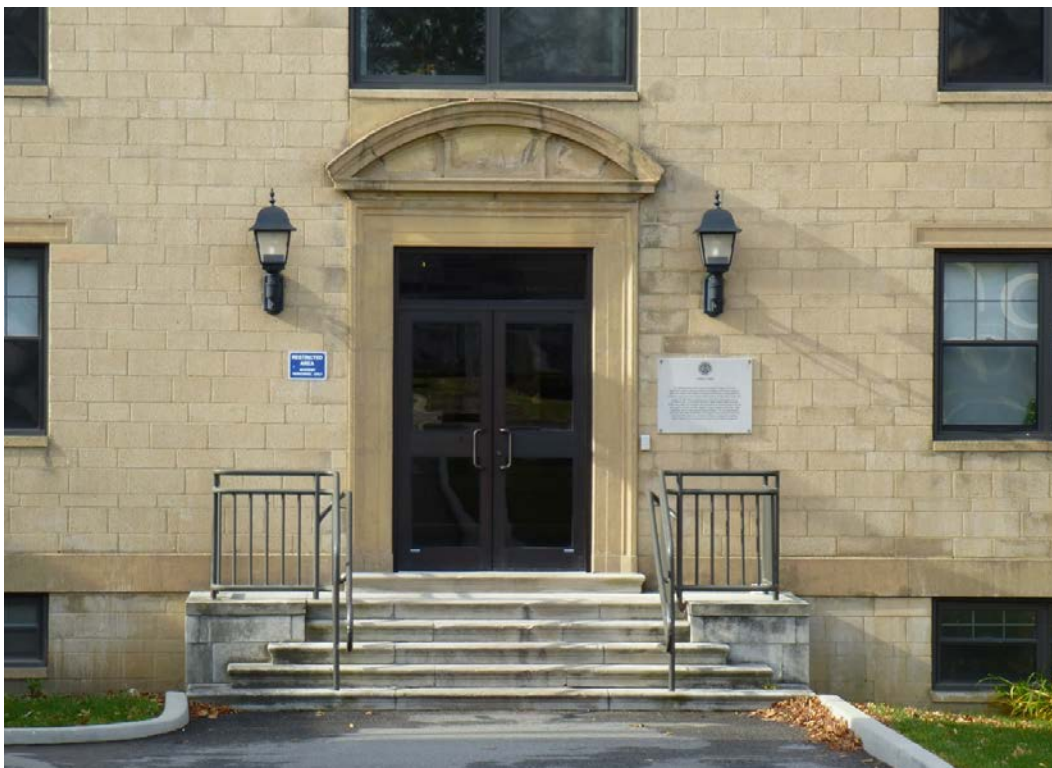
Figure 88. West entrance to Palmer Hall (ERDC-CERL, 2013).
