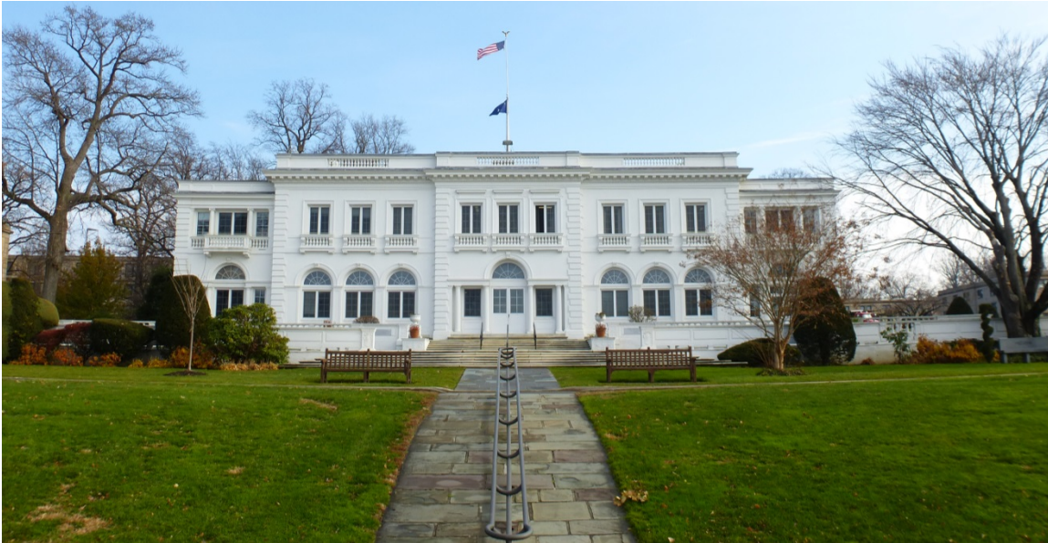
Figure 70. West façade of Wiley Hall (ERDC-CERL, 2013).
