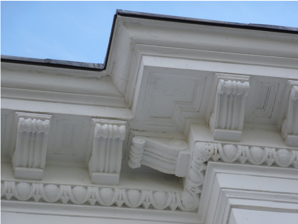
Figure 75. Corbels and egg-and-dart detail on the soffit on the west façade of Wiley Hall (ERDC-CERL, 2013).
