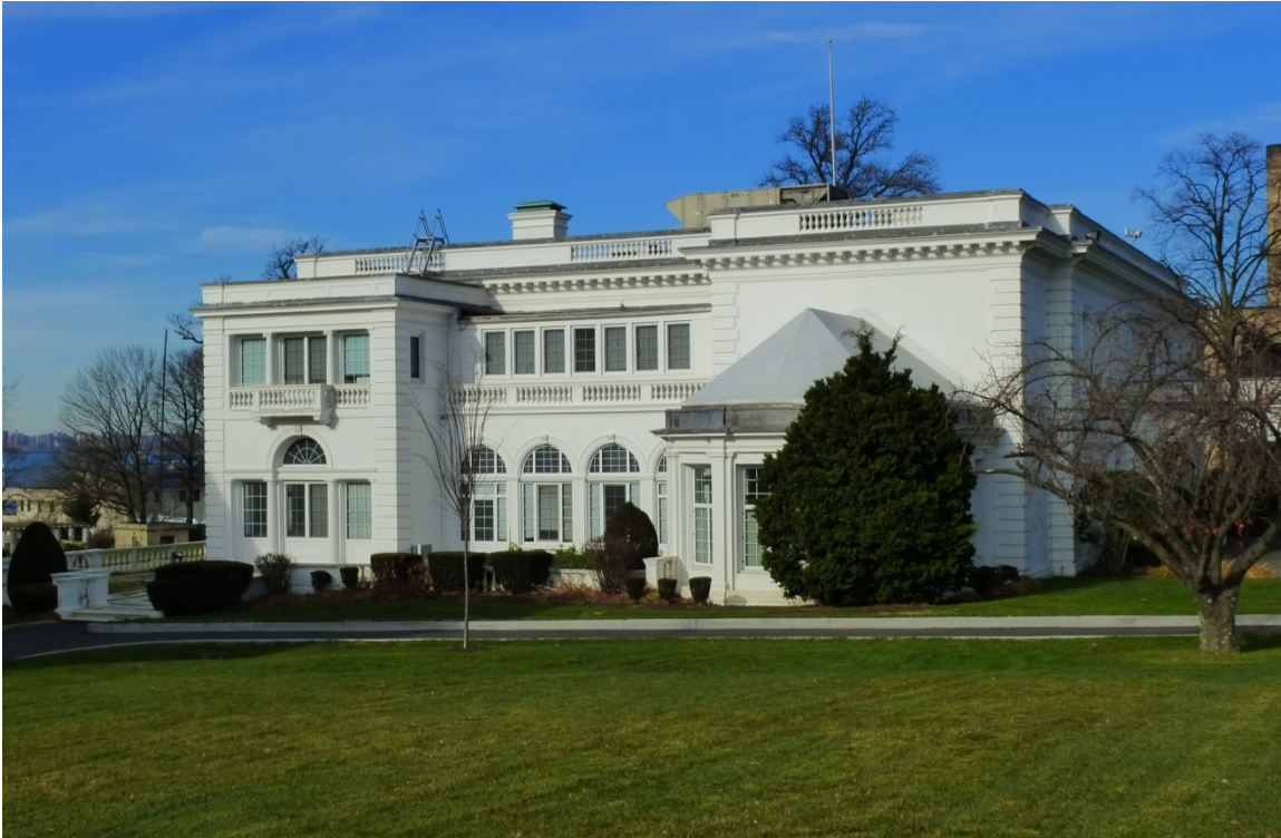
Figure 68. South façade of Wiley Hall (ERDC-CERL, 2013).
