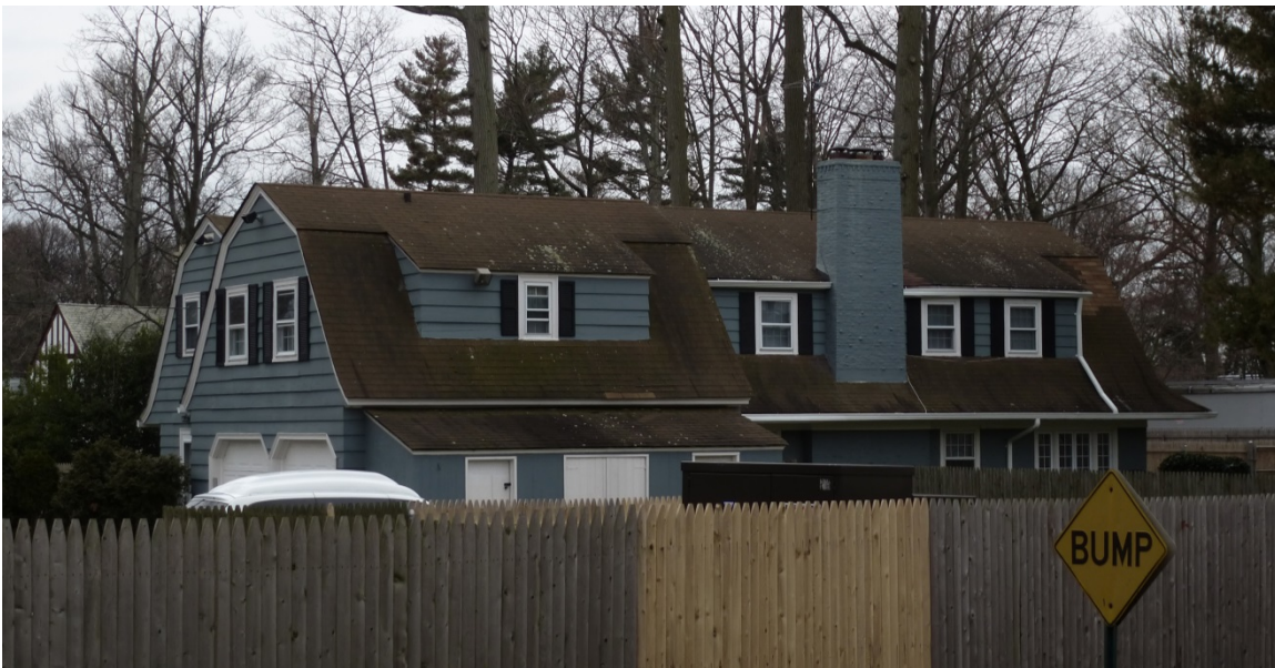
Figure 62. North façade of Quarters B (ERDC-CERL, 2013).
