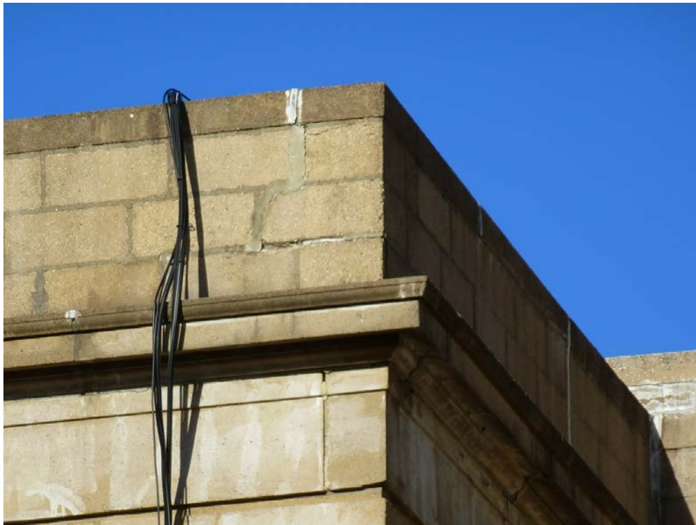
Figure 93. Detail of cornice and parapet on Cleveland Hall (ERDC-CERL, 2013).
