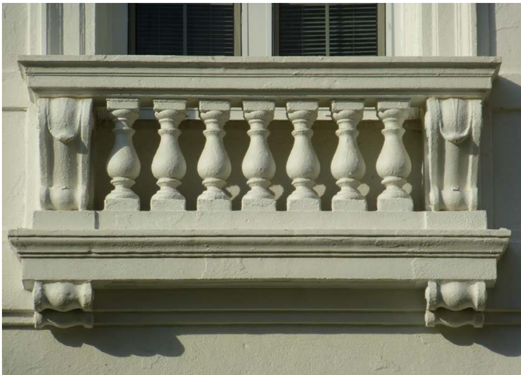
Figure 72. Balustrade beneath window on the east façade of Wiley Hall (ERDC-CERL, 2013).
