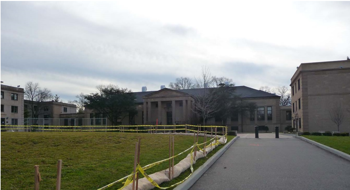
Figure 141. North façade of Delano Hall with Blarney Square in the foreground (ERDC-CERL, 2013).
