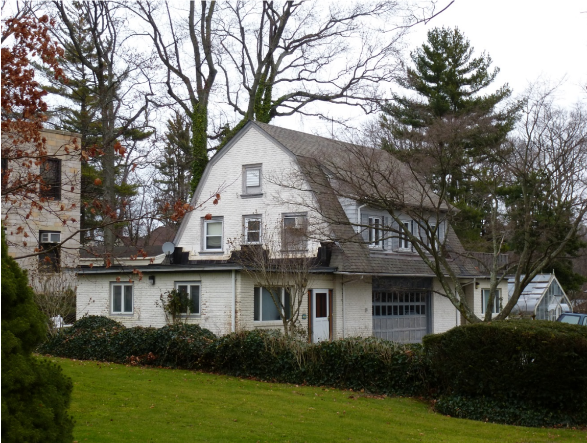
Figure 52. Southwest oblique of Quarters J (Neiley garage) (ERDC-CERL, 2013).
