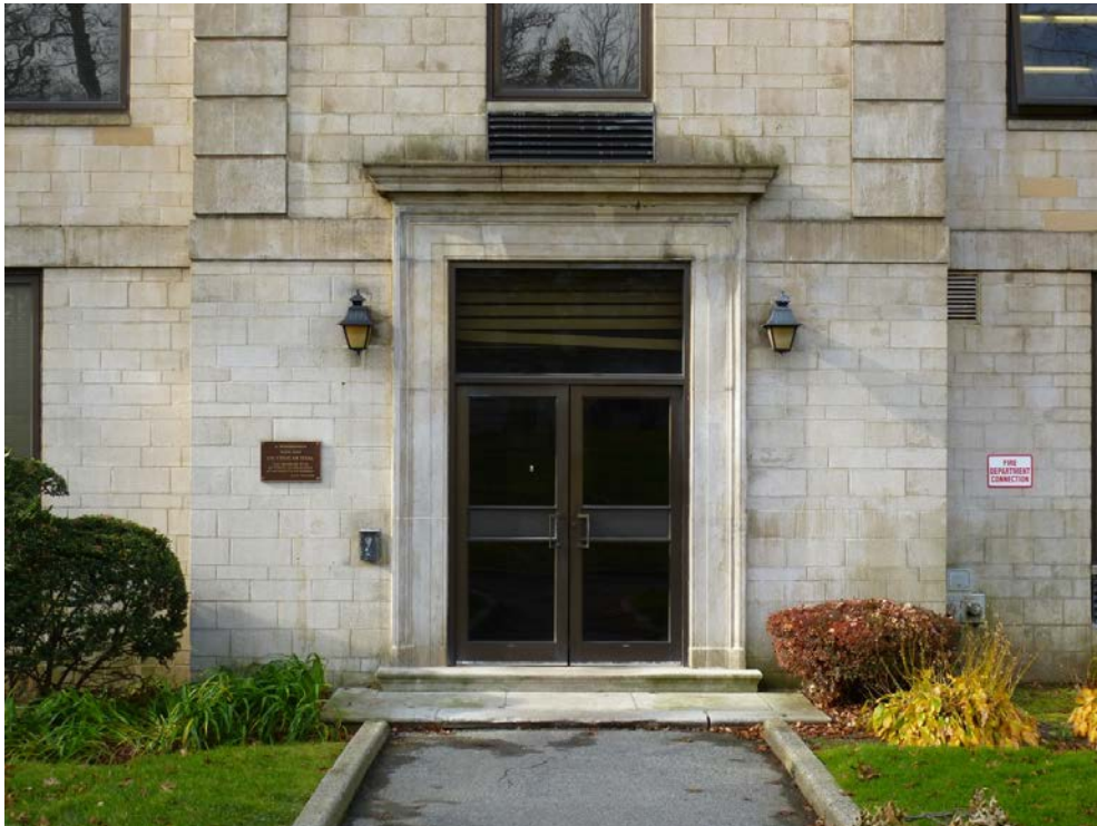
Figure 122. East entrance to Fulton Hall (ERDC-CERL, 2013).
