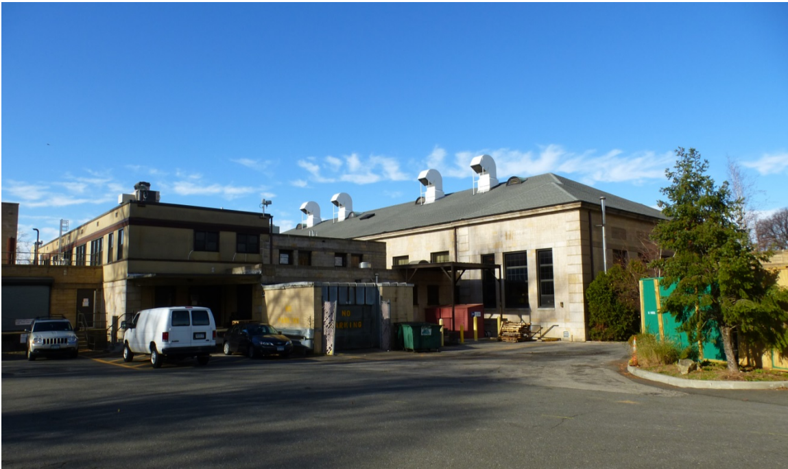
Figure 143. Southeast oblique of Delano Hall, showing the kitchen wing on the left and the dining hall on the right (ERDC-CERL, 2013).
