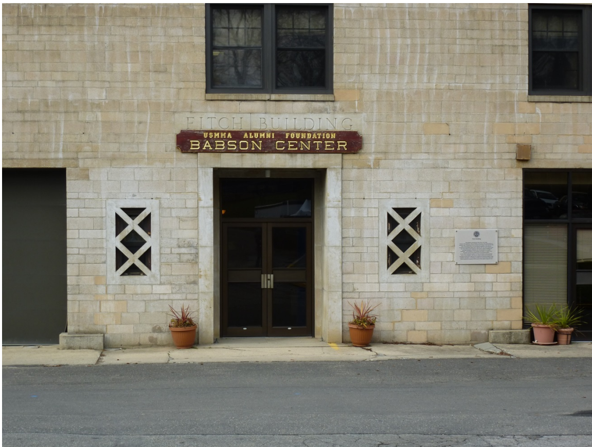
Figure 135. Entrance to the Fitch Building on the east façade (ERDC-CERL, 2013).
