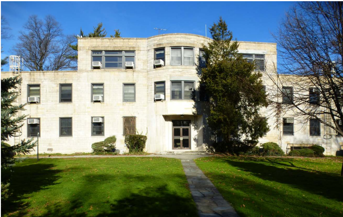
Figure 180. South façade of Patten Clinic (ERDC-CERL, 2013).
