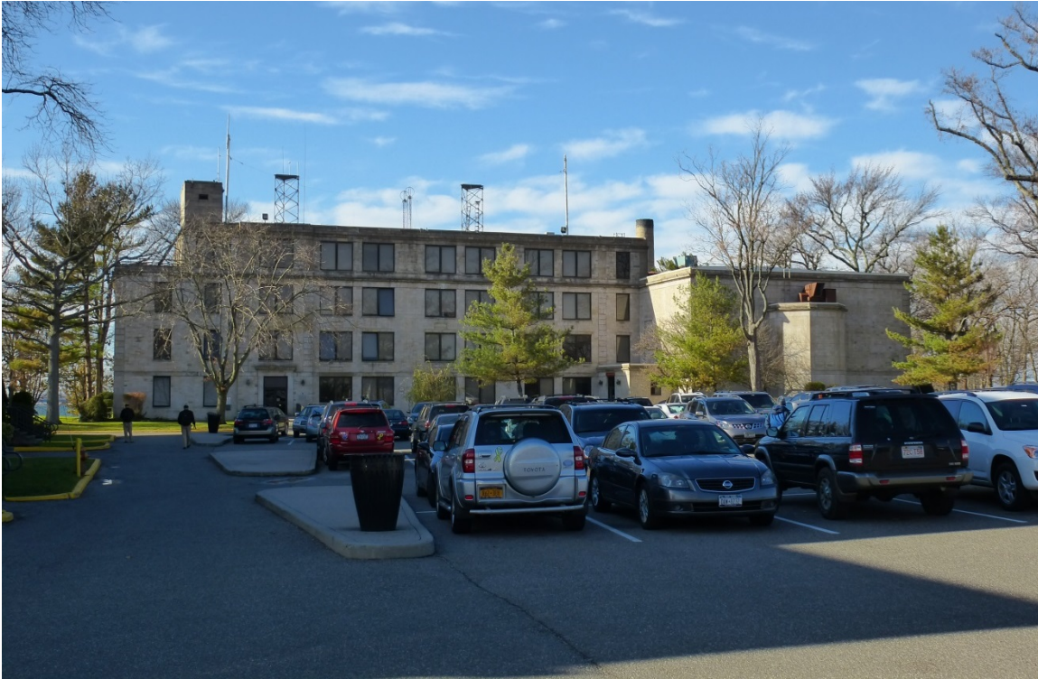
Figure 118. East façade of Bowditch Hall (ERDC-CERL, 2013).
