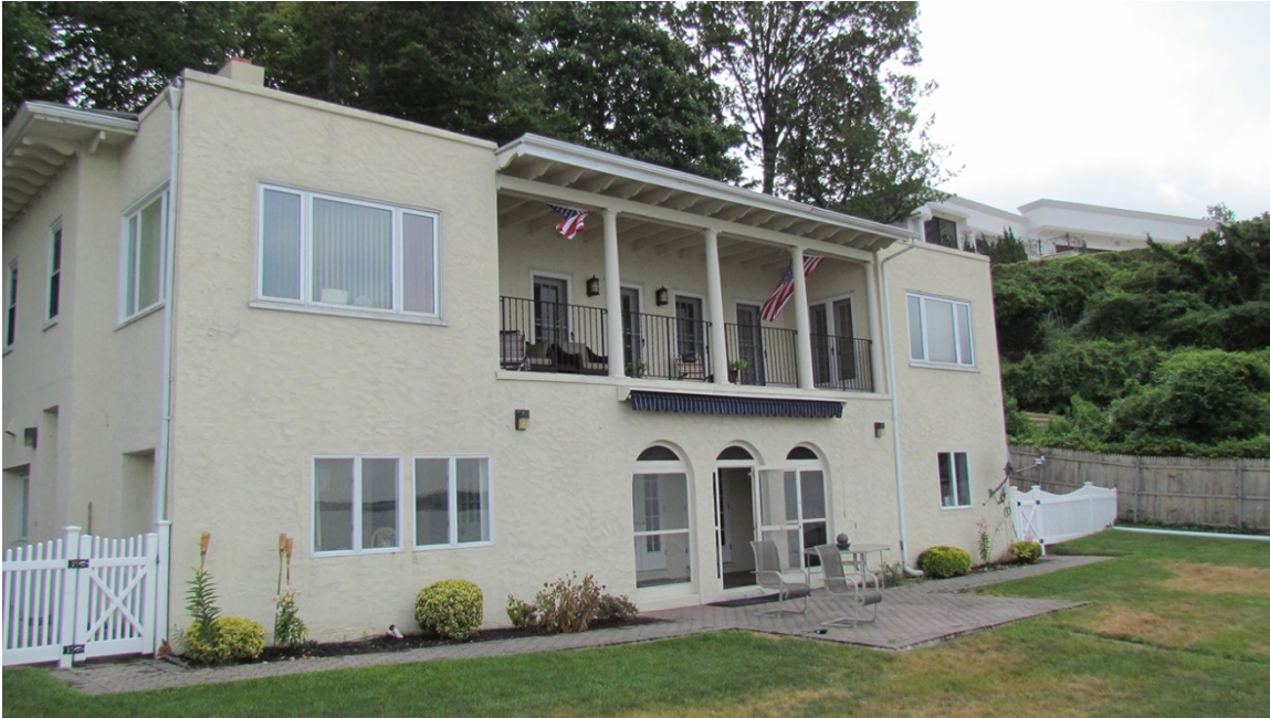
Figure 46. West façade of Quarters D (Grenwolde Casino) (USMMA, 2013).
