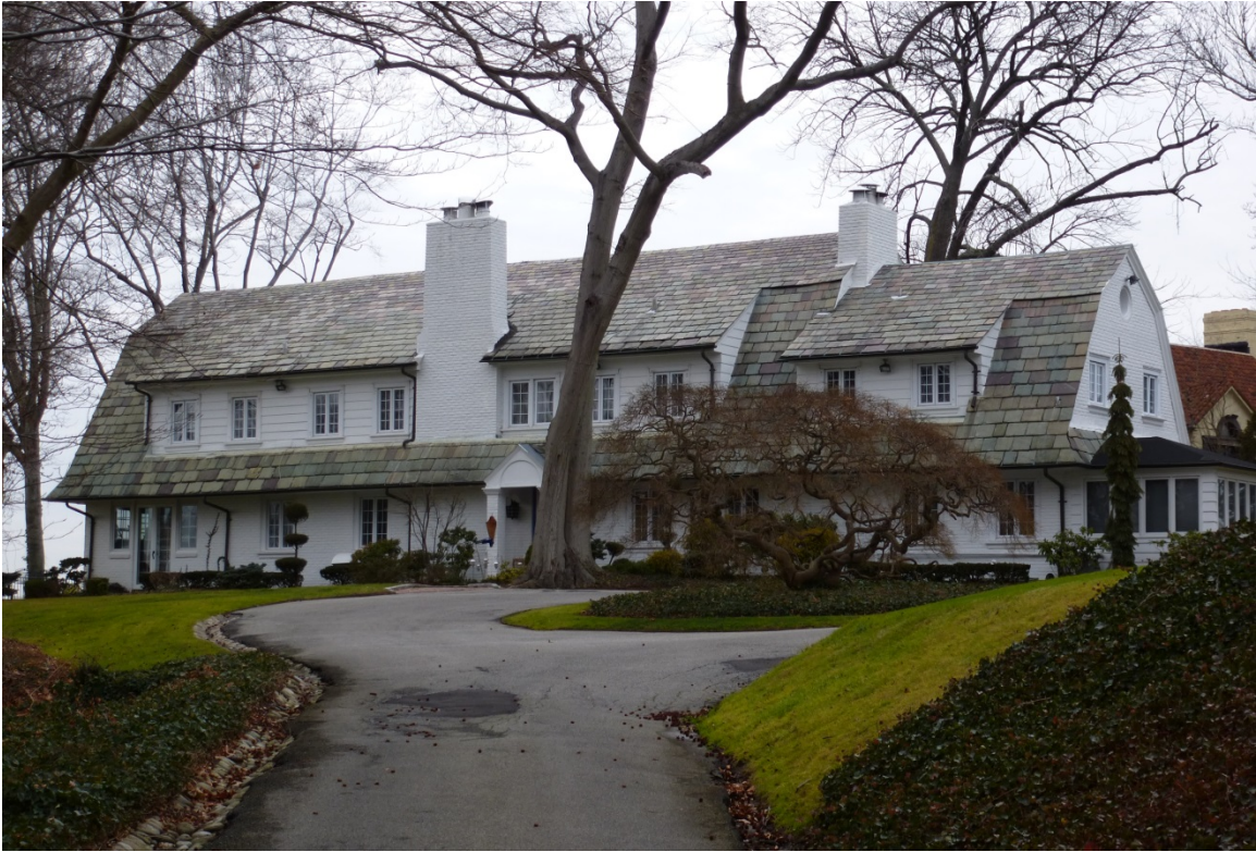
Figure 48. South façade of Quarters A (Neiley house) (ERDC-CERL, 2013).
