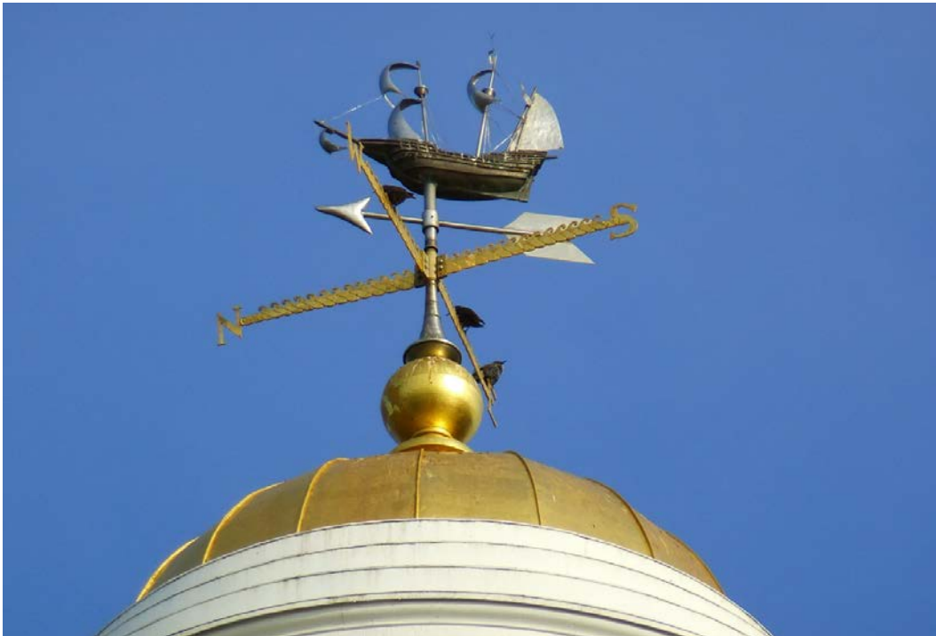
Figure 189. Weathervane detail of the Memorial Chapel steeple (ERDC-CERL, 2013).
