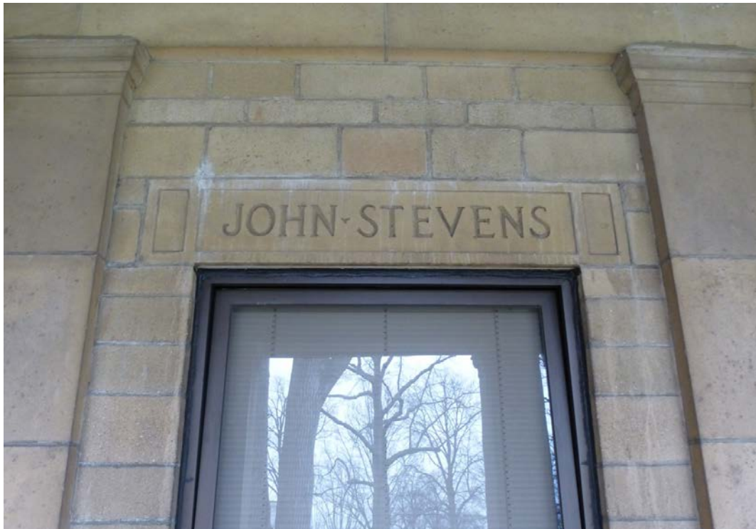
Figure 124. Inscription on cast-stone lintel at portico entrance to Fulton Hall (ERDC-CERL, 2013).
