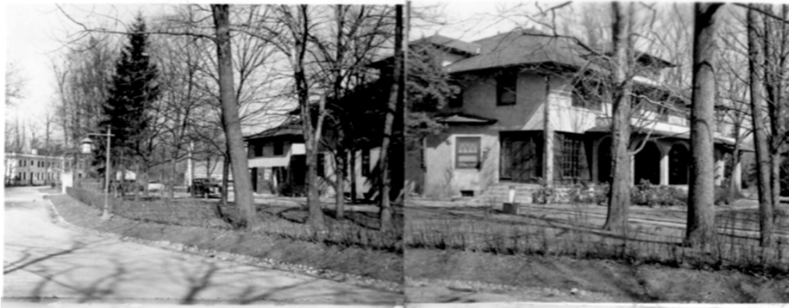
Figure 23. Panoramic View of the Marchant house and garage (both demolished), 1942 (NARA RG 178).
