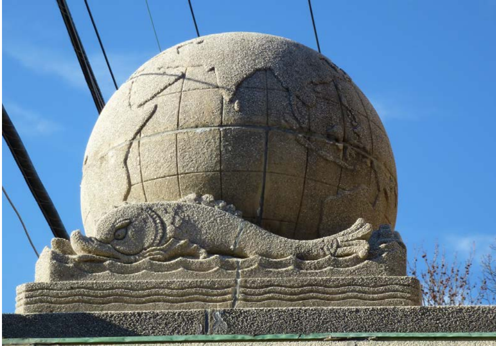
Figure 205. Globe and dolphin detail on top of Vickery Gate guardroom on the north side of Steamboat Road; the same detail is also on top of the south side guard room. (ERDC-CERL, 2013).
