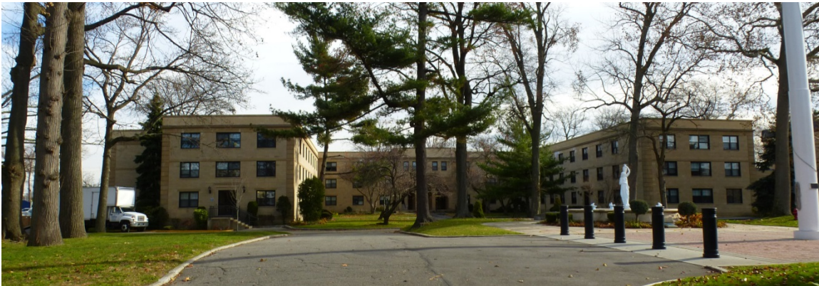
Figure 97. West façades of Jones Hall [left], Truxton Arcade [center], and Barry Hall [right] (ERDC-CERL, 2013).
