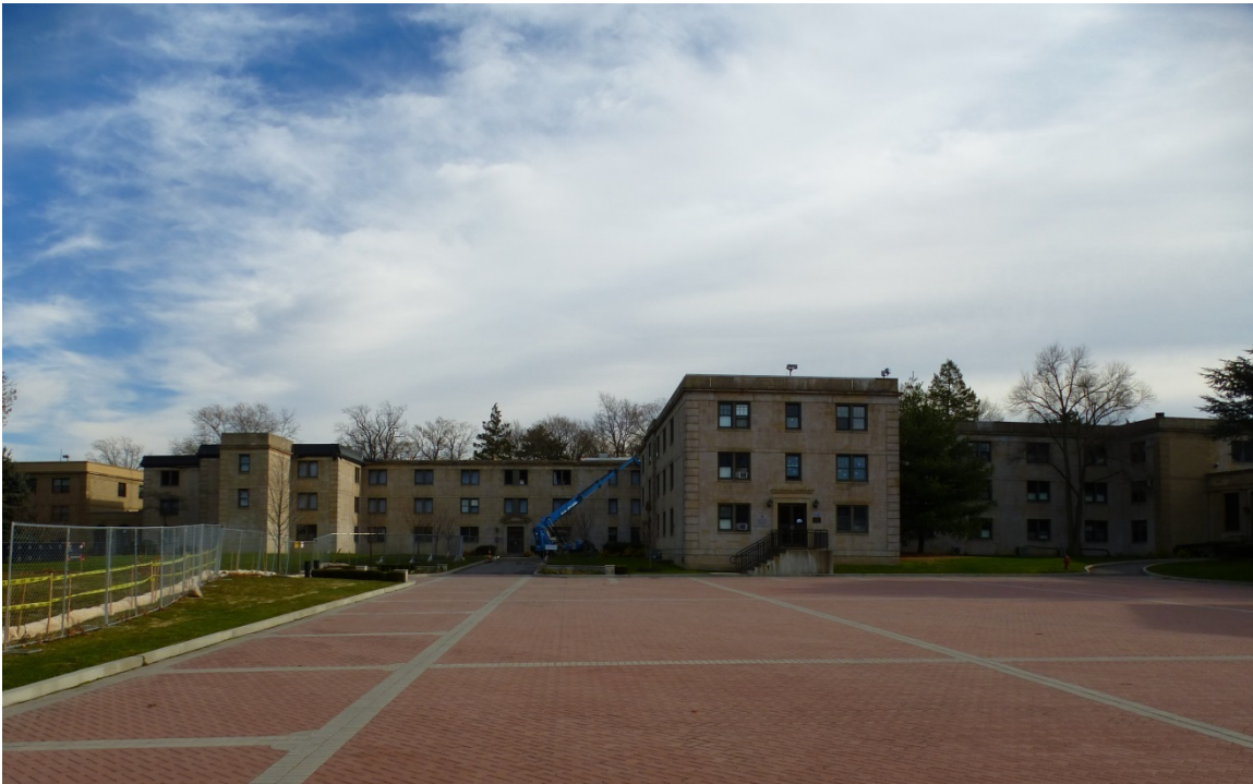
Figure 85. West façades of Rogers Hall [left] and Cleveland Hall [right] (ERDC-CERL, 2013).
