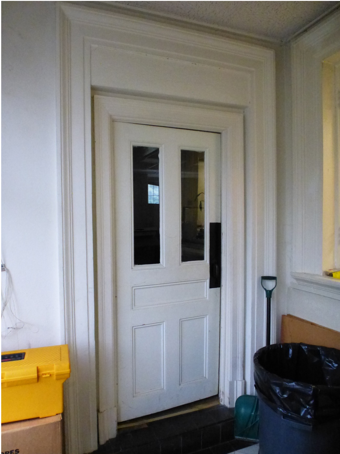
Figure 82. Door and door surround in Wiley Hall (ERDC-CERL, 2013).
