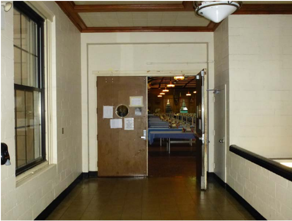
Figure 156. Replacement interior doors in Delano Hall (ERDC-CERL, 2013).
