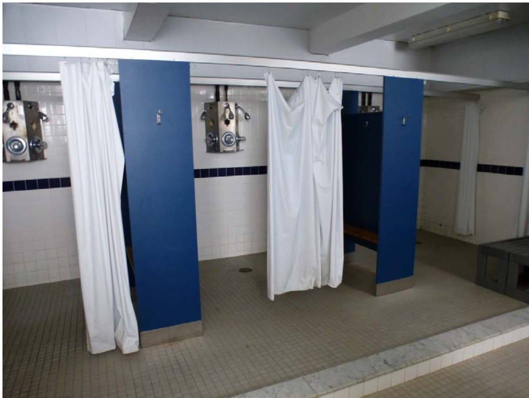
Figure 195. Noncontributing shower interior (ERDC-CERL, 2013).
