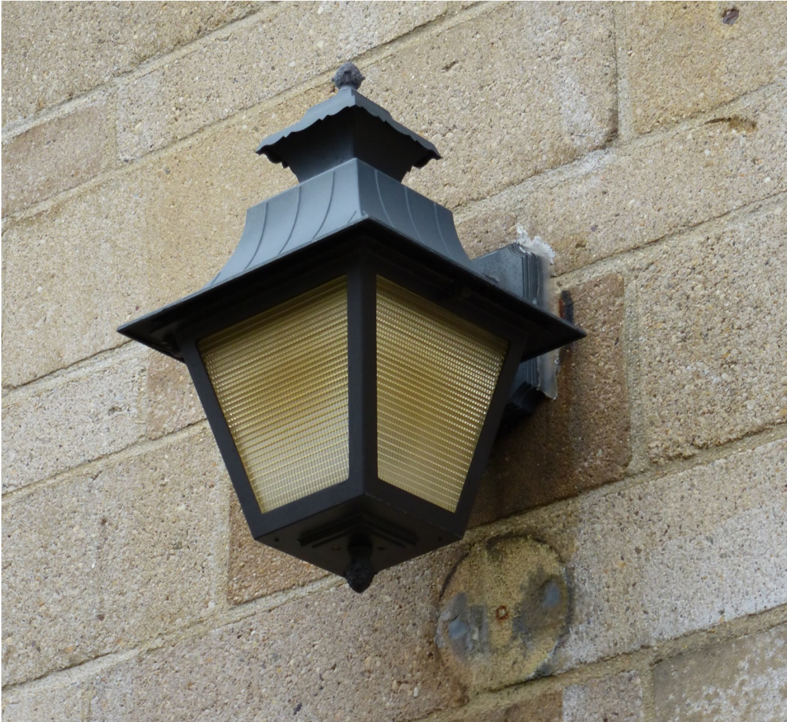
Figure 112. Replacement light fixture at entrance (ERDC-CERL, 2013).
