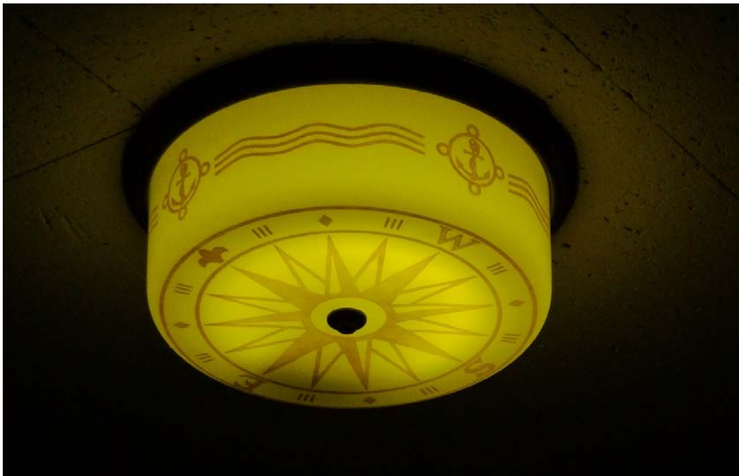
Figure 131. Original light fixture in lobby of auditorium in Bowditch Hall (ERDC-CERL, 2013).
