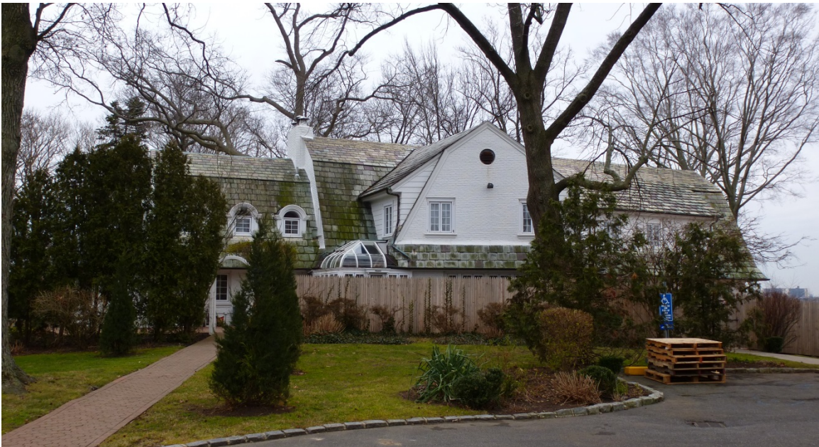
Figure 49. North façade of Quarters A (Neiley house) (ERDC-CERL, 2013).
