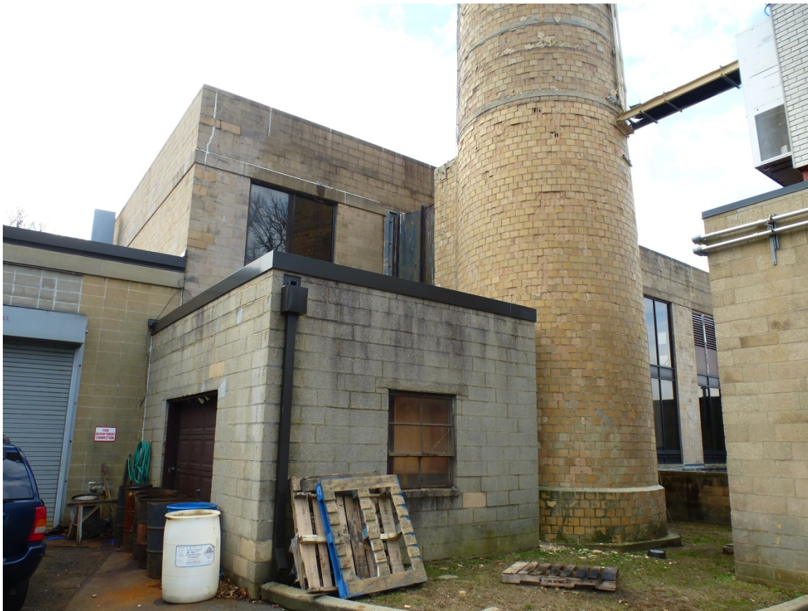
Figure 116. Mechanical room and base of chimney at the northeast corner of Fulton Hall (ERDC-CERL, 2013).
