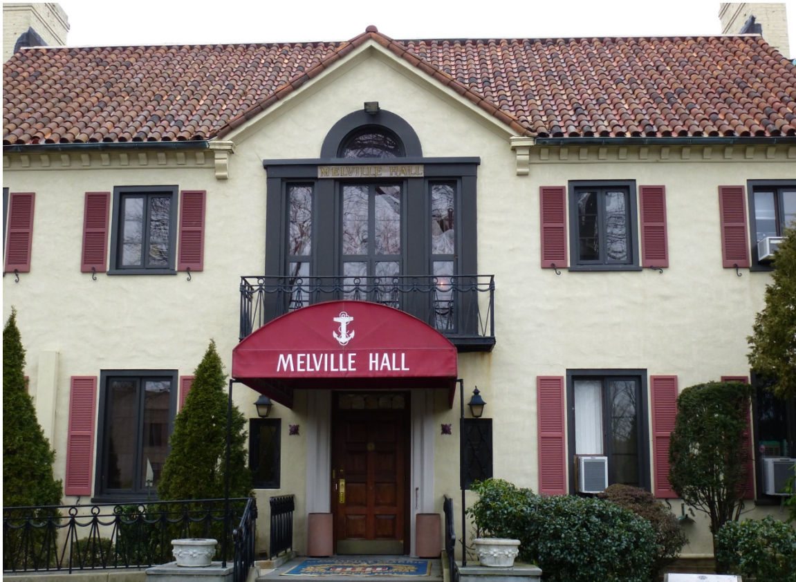
Figure 55. Detail of the east entrance to Melville Hall (ERDC-CERL, 2013).
