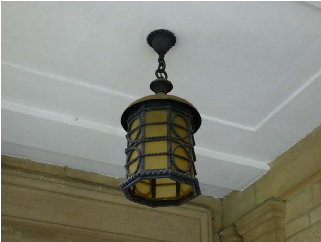
Figure 126. Original light fixture at portico entrance to Fulton Hall (ERDC-CERL, 2013).
