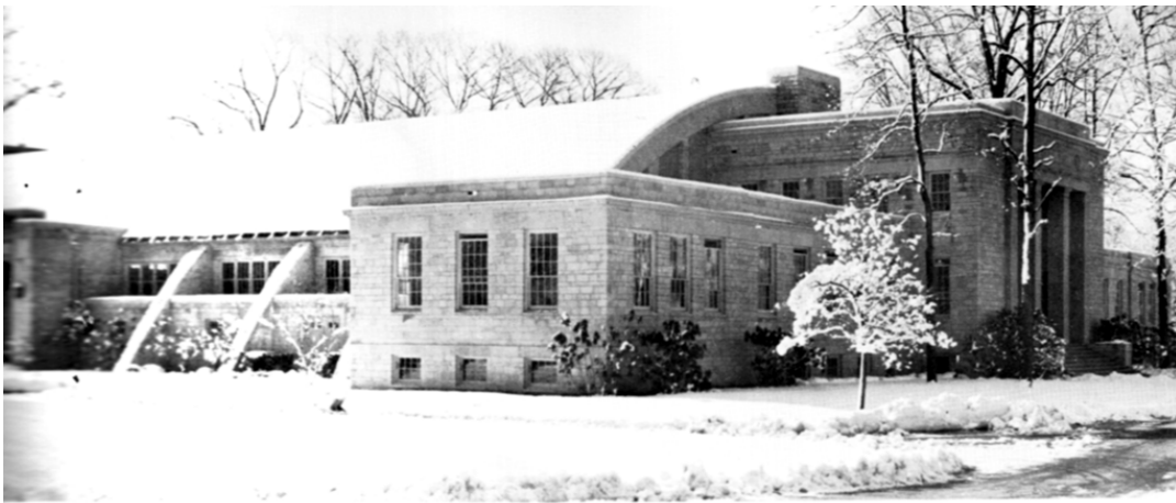
Figure 159. Northwest oblique of O'Hara Hall (drill hall/gymnasium), 1944 (Bland Library, USMMA).
