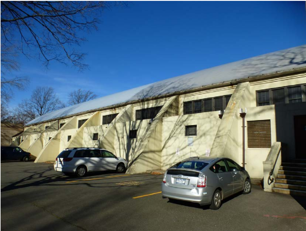
Figure 164. South side of O'Hara Hall, showing buttresses (ERDC-CERL, 2013).
