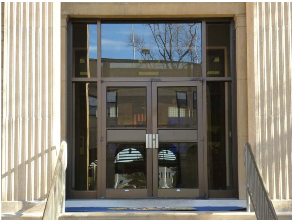
Figure 166. Replacement doors on the west façade entrance of O'Hara Hall (ERDC-CERL, 2013).
