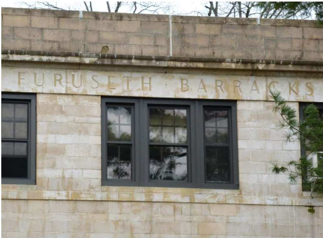
Figure 108. Beltcourse, replacement windows, cornice, inscription, and parapet on Furusetth Hall (ERDC-CERL, 2013).
