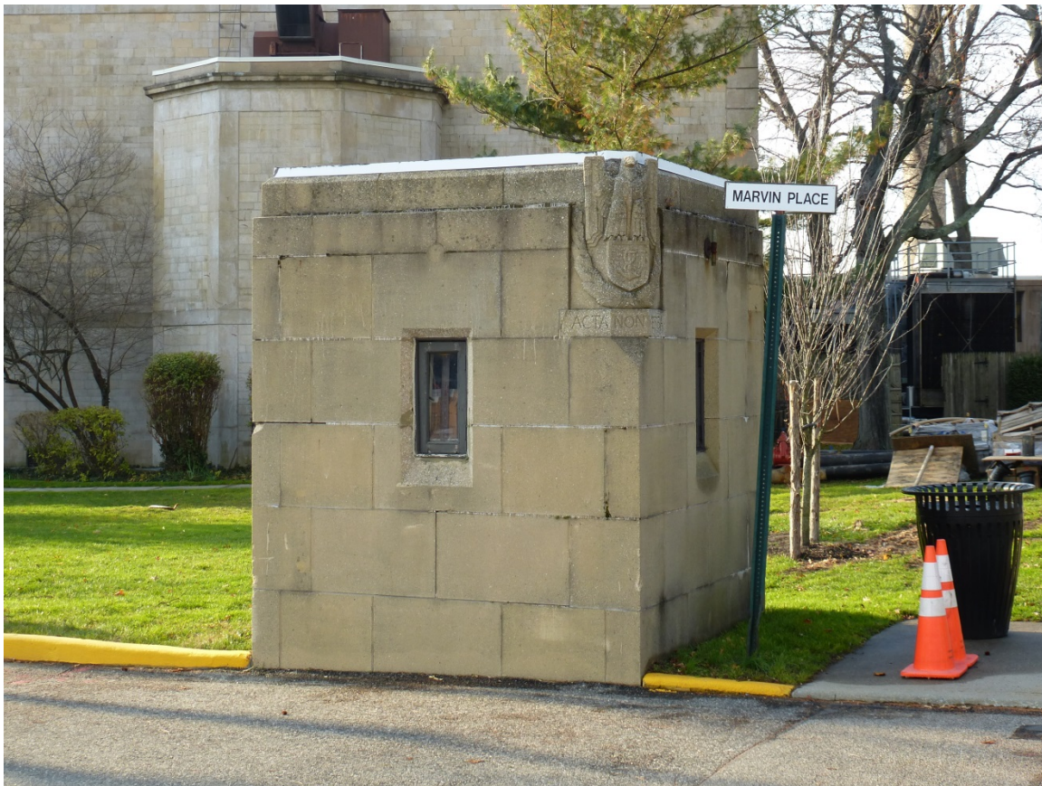
Figure 206. Northeast oblique of the Marvin Place Gate guard house on the south side of Steamboat Road (ERDC-CERL, 2013).
