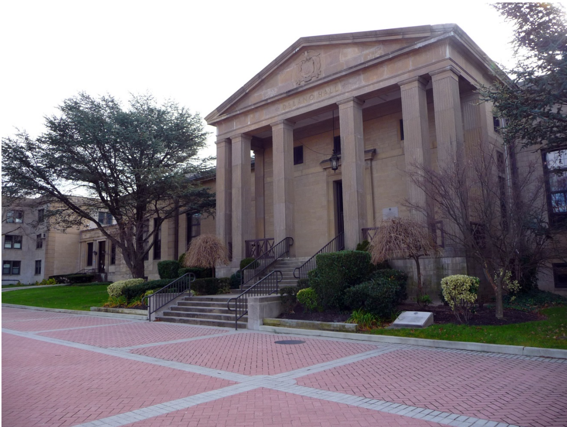
Figure 142. North façade of the Delano Hall entrance portico (ERDC-CERL, 2013).
