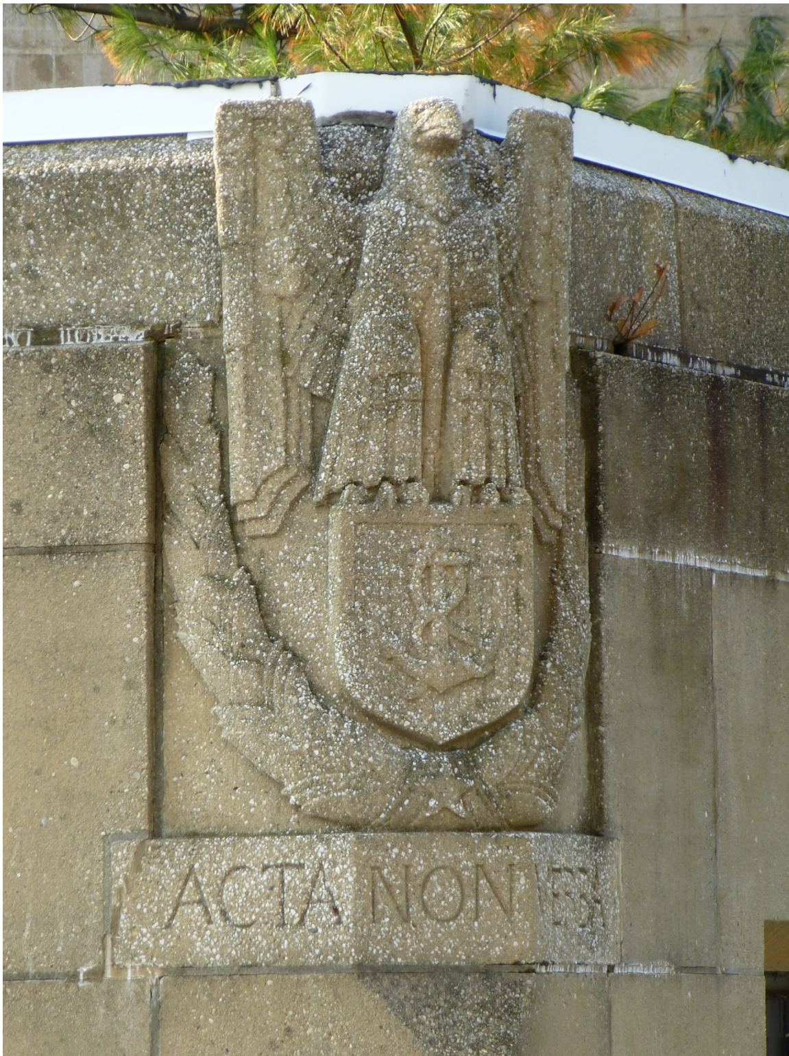
Figure 208. Cast-stone eagle on the northeast corner of the Marvin Place Gate guard house on the south side of Steamboat Road (ERDC-CERL, 2013).
