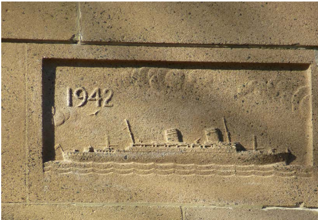
Figure 103. Detail of a cast-stone bas-relief on the east façade of the Truxton Arcade (ERDC-CERL, 2013).
