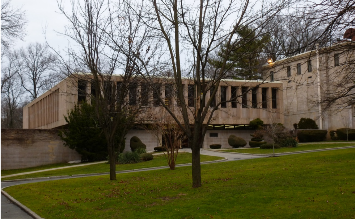
Figure 199. South façade (front) of Bland Library (ERDC-CERL, 2013).
