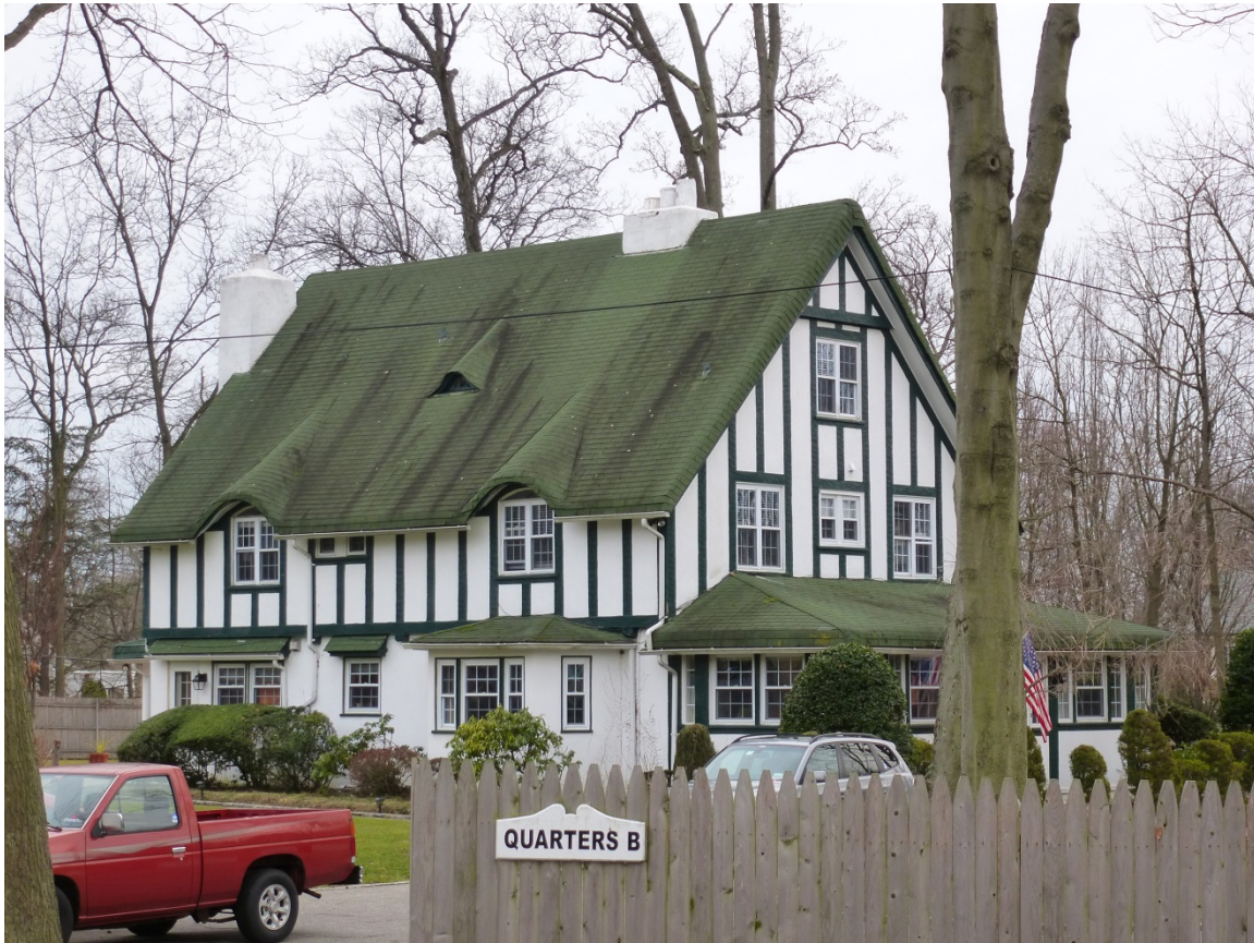
Figure 65. Northwest oblique of Quarters C (Vreeland house) (ERDC-CERL, 2013).
