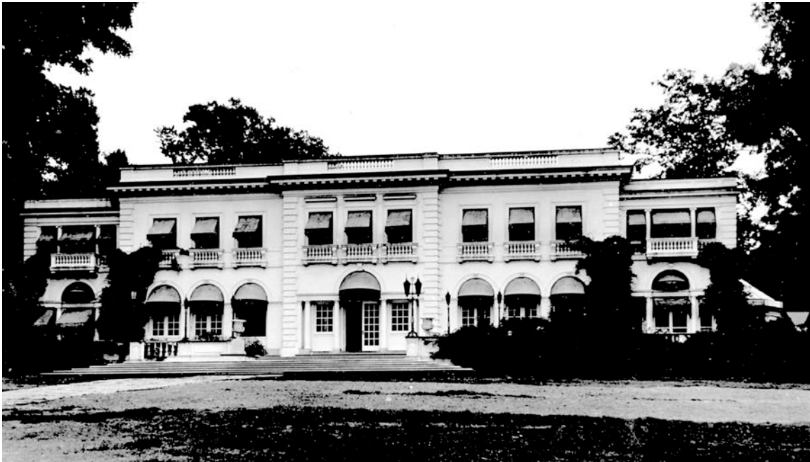
Figure 29. Former west-side loggia, newly enclosed on Wiley Hall, 1942 (Bland Library, USMMA).
