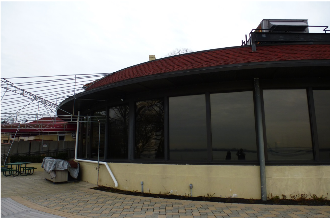
Figure 56. Southwest portions of the ballroom addition to Melville Hall (ERDC-CERL, 2013).
