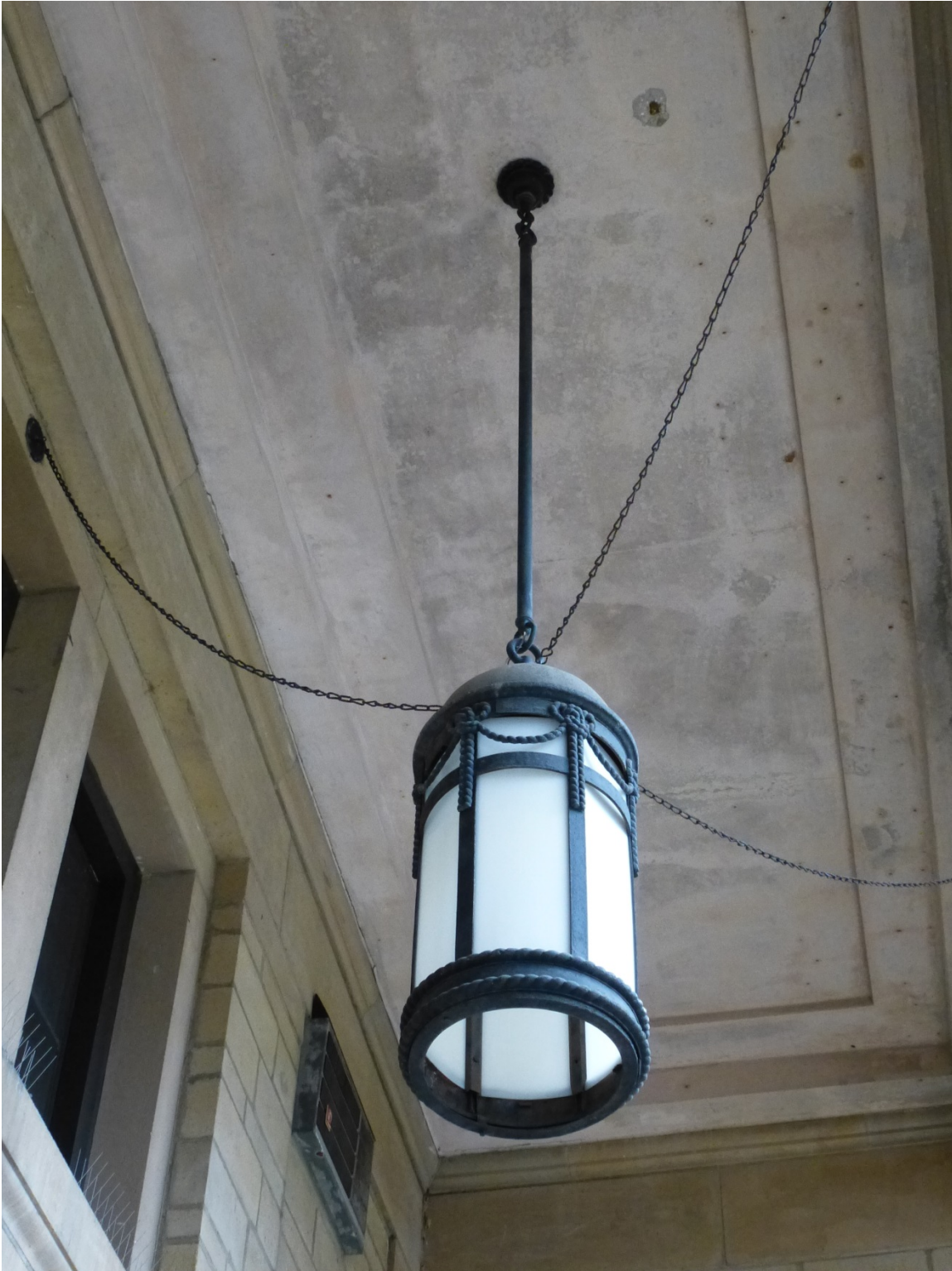
Figure 171. Original ceiling fixture on portico of O'Hara Hall (ERDC-CERL, 2013).
