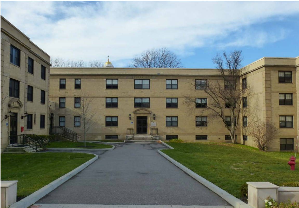
Figure 87. Close-up of the entry (center) on east façade of Palmer Hall, with entrance to Murphy Hall shown on the left (ERDC-CERL, 2013).
