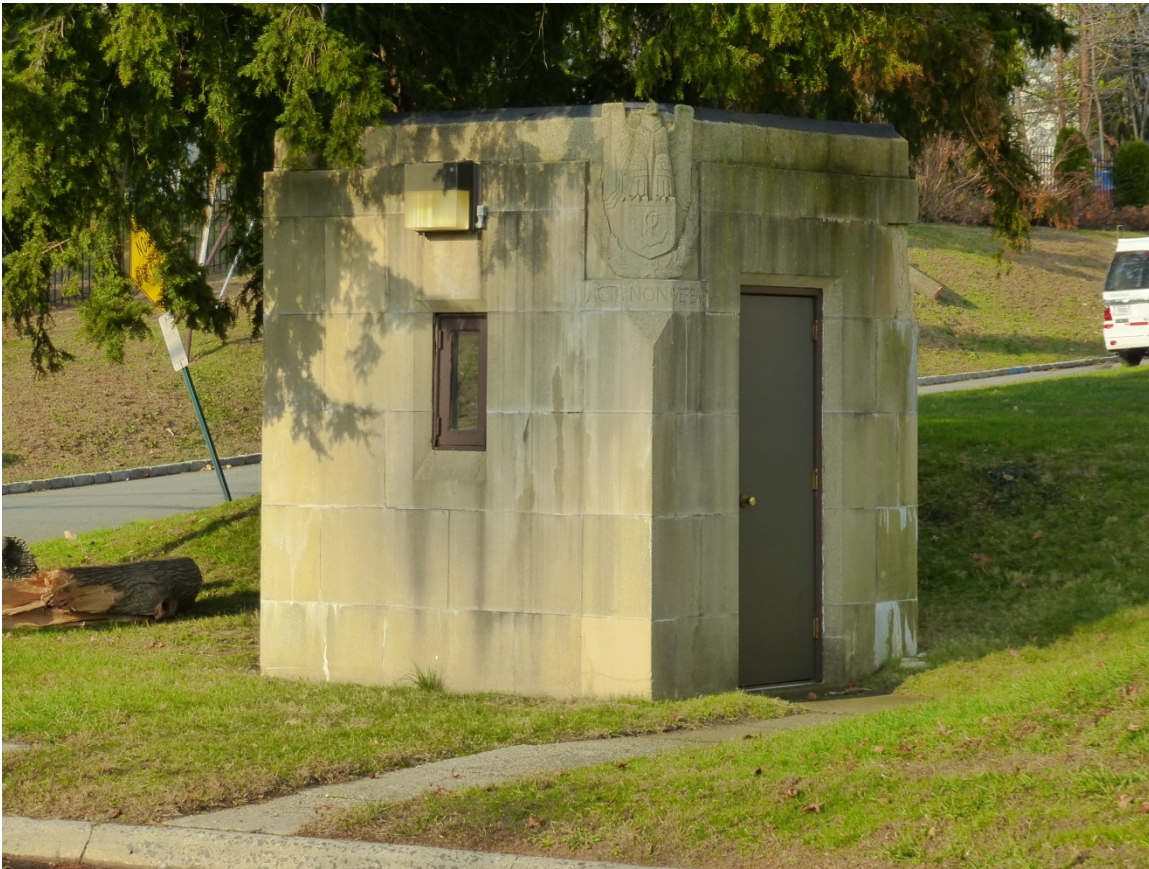
Figure 207. Southeast oblique of the Marvin Place Gate guard house on the north side of Steamboat Road (ERDC-CERL, 2013).
