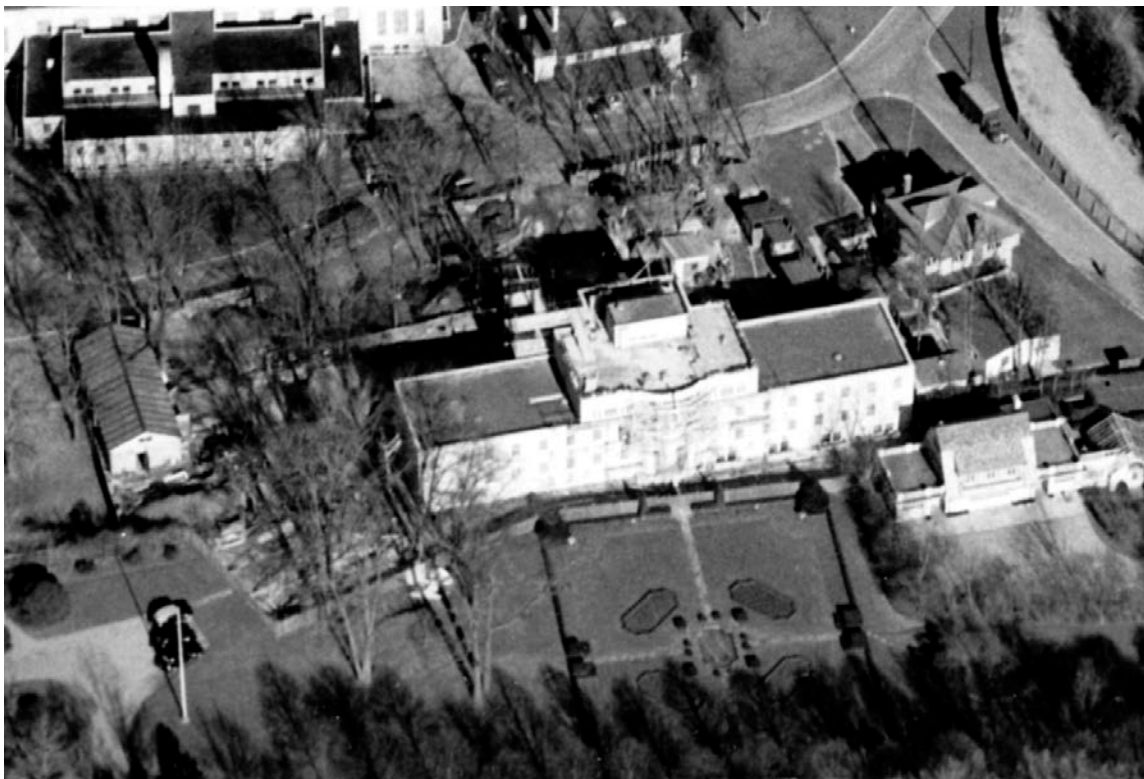
Figure 21. 1943 aerial showing the new Patten Hospital with the Neiley garden in the lower center, the expanded Neiley garage (Quarters J) in the lower right, and the Meighan garage (Quarters K) in the upper right (Bland Library, USMMA).
