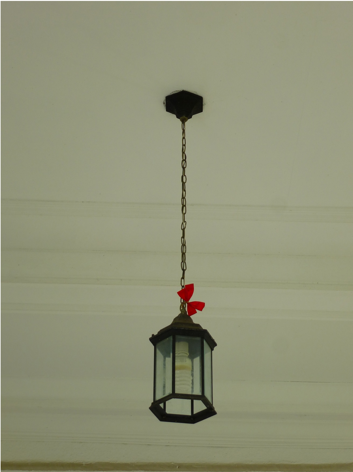
Figure 74. Light fixture underneath porte cochere on the east façade of Wiley Hall (ERDC-CERL, 2013).
