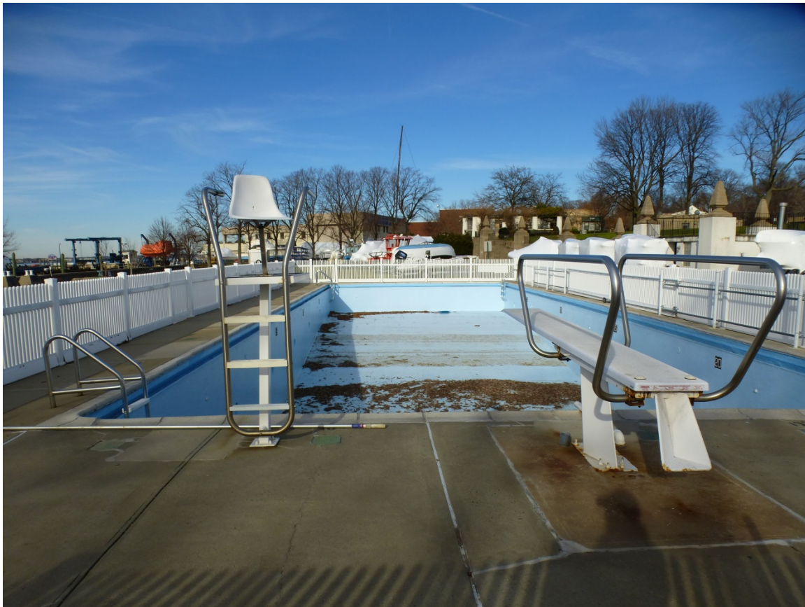
Figure 211. Looking to the north over Eldridge Pool (ERDC-CERL, 2013).
