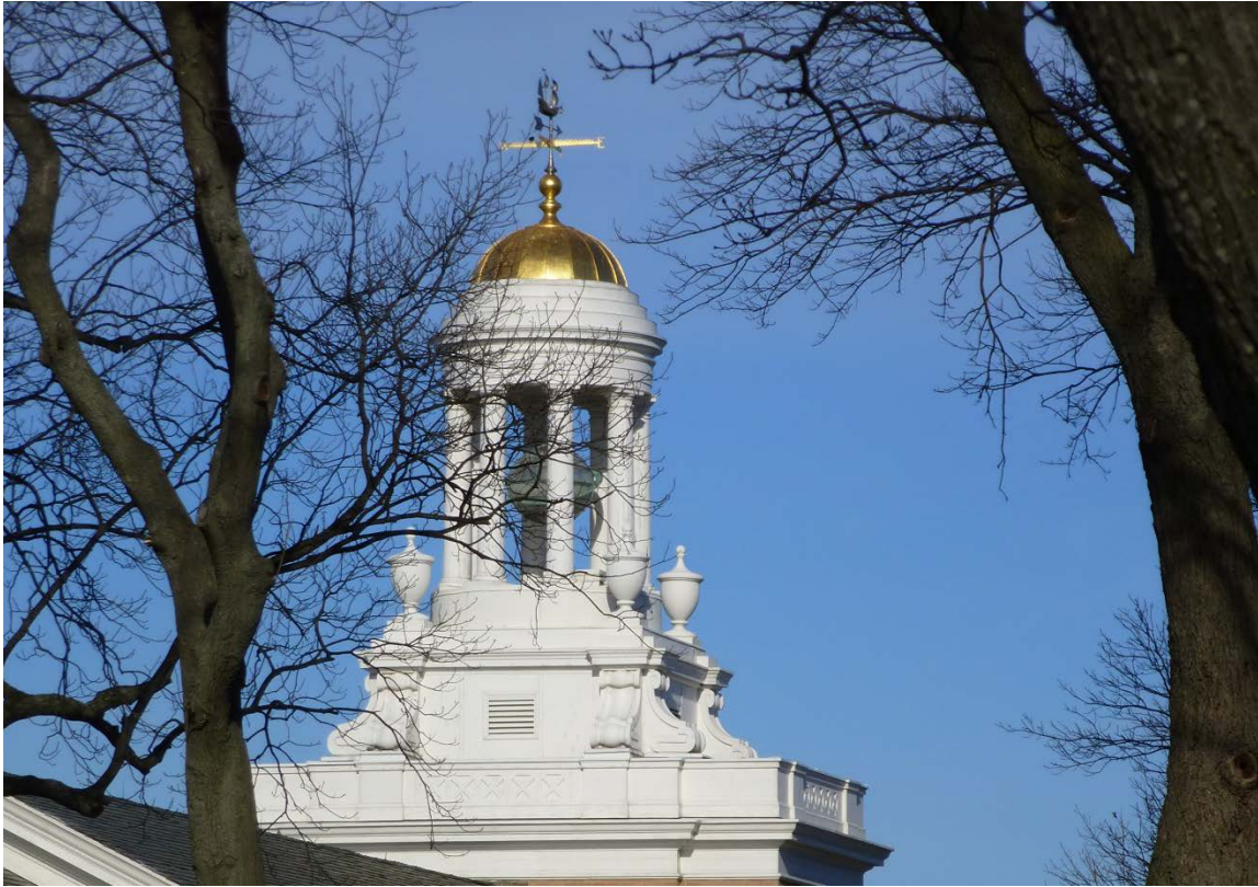
Figure 188. South side of the Memorial Chapel steeple (ERDC-CERL, 2013).
