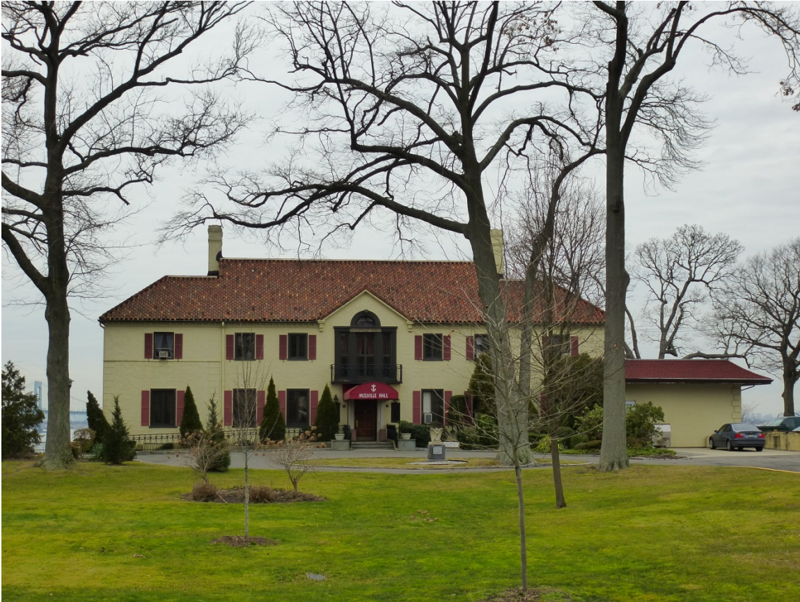
Figure 54. East façade of Melville Hall (ERDC-CERL, 2013).
