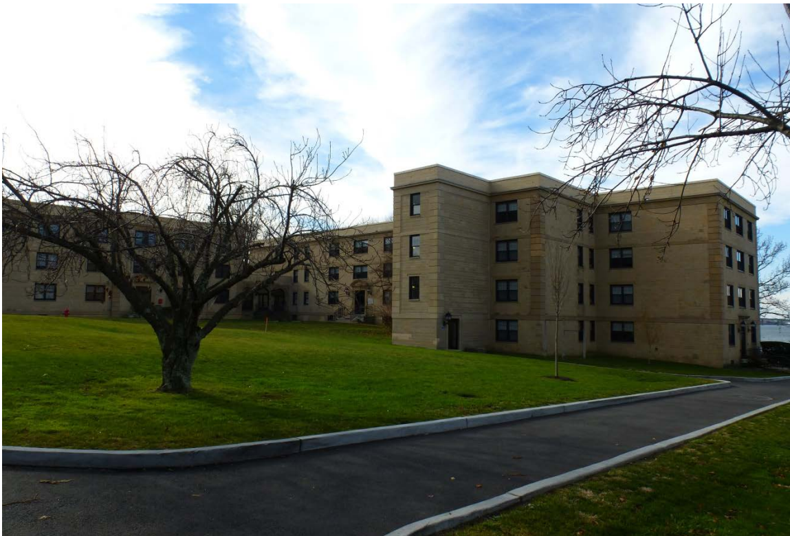
Figure 86. North façade of Murphy Hall [left] and east façade of Palmer Hall [right] (ERDC-CERL, 2013).
