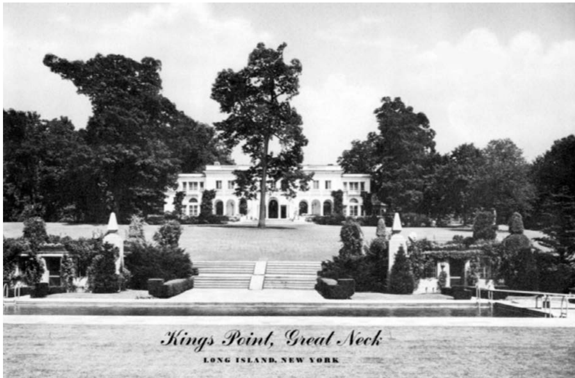
Figure 5. Bendel/Chrysler mansion (Wiley Hall) and grounds, west façade, 1941 (Previews Incorporated).
