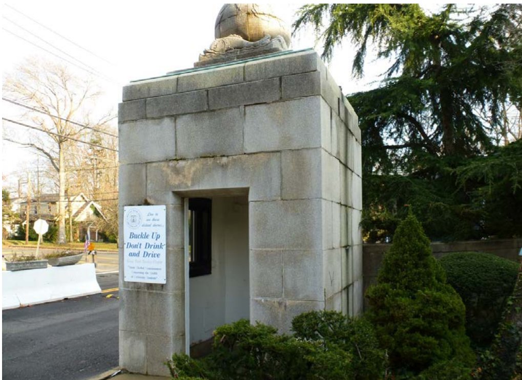
Figure 204. West façade of the Vickery Gate guard room on the south side of Steamboat Road (ERDC-CERL, 2013). (Note that this gate's wall does not have the upper layer of stone.)
