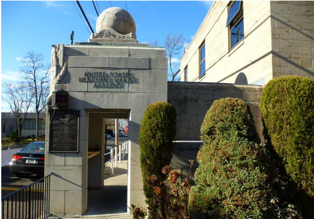
Figure 203. East façade of the Vickery Gate guard room on the north side of Steamboat Road (ERDC-CERL, 2013). Note the added top layer of wall extending from guard room that is not part of original plans.
