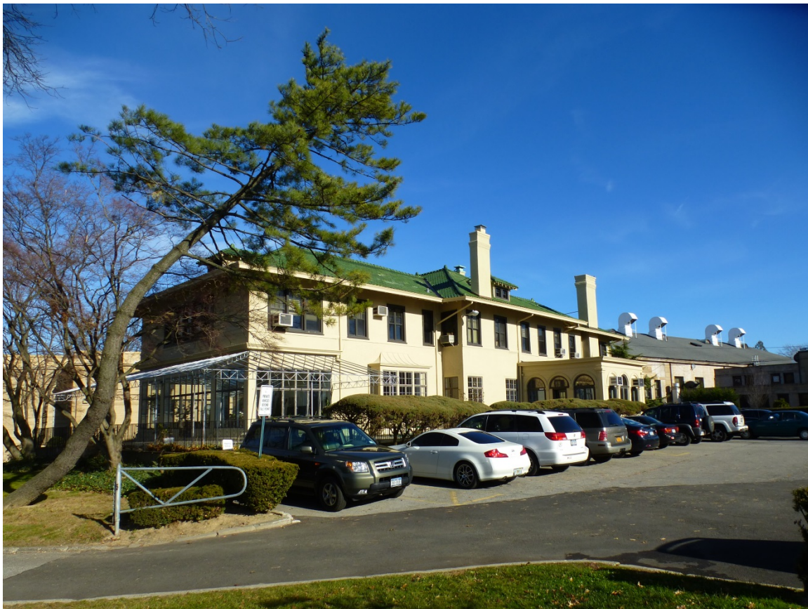
Figure 60. Southwest oblique of Land Hall (Schenck house) (ERDC-CERL, 2013).
