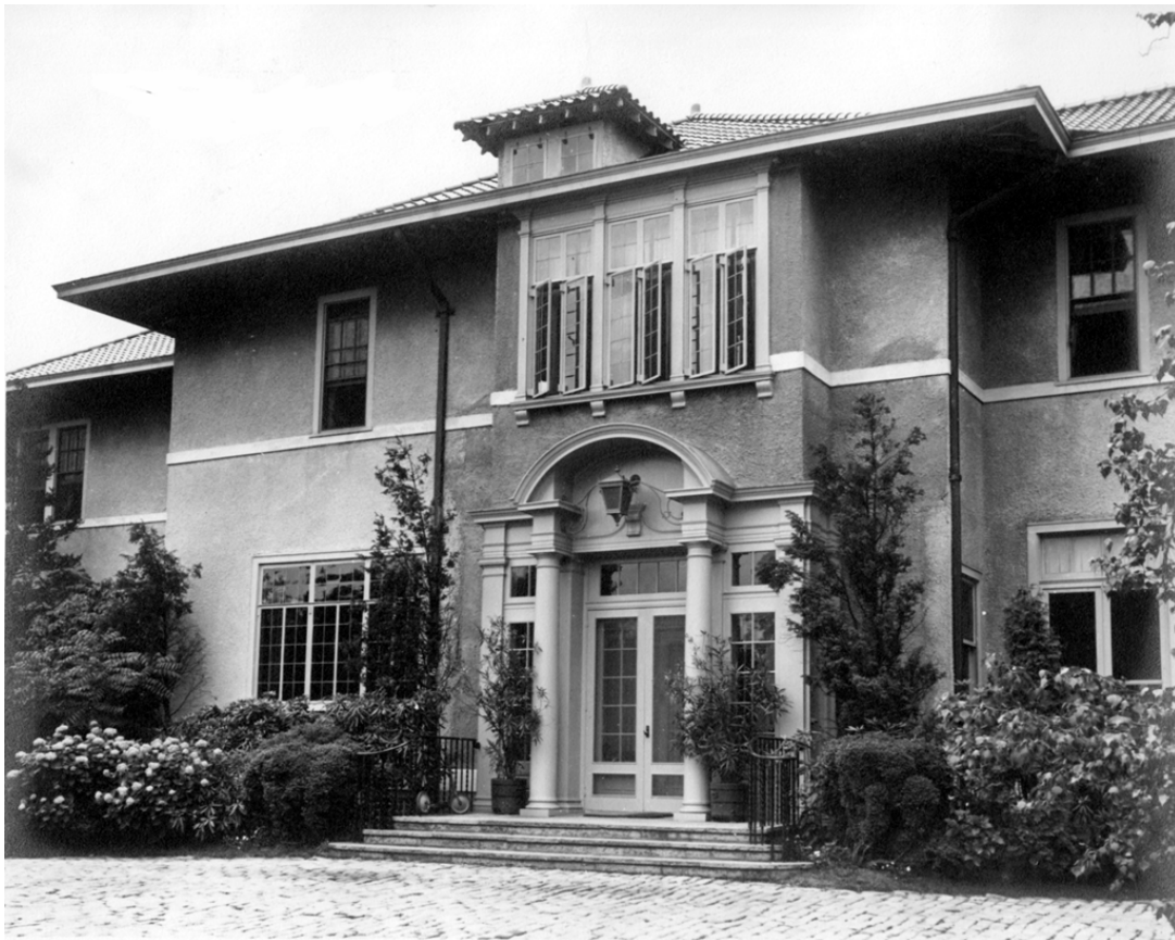
Figure 58. North façade of Land Hall (Schenck house), 1942 (NARA RG 178).
