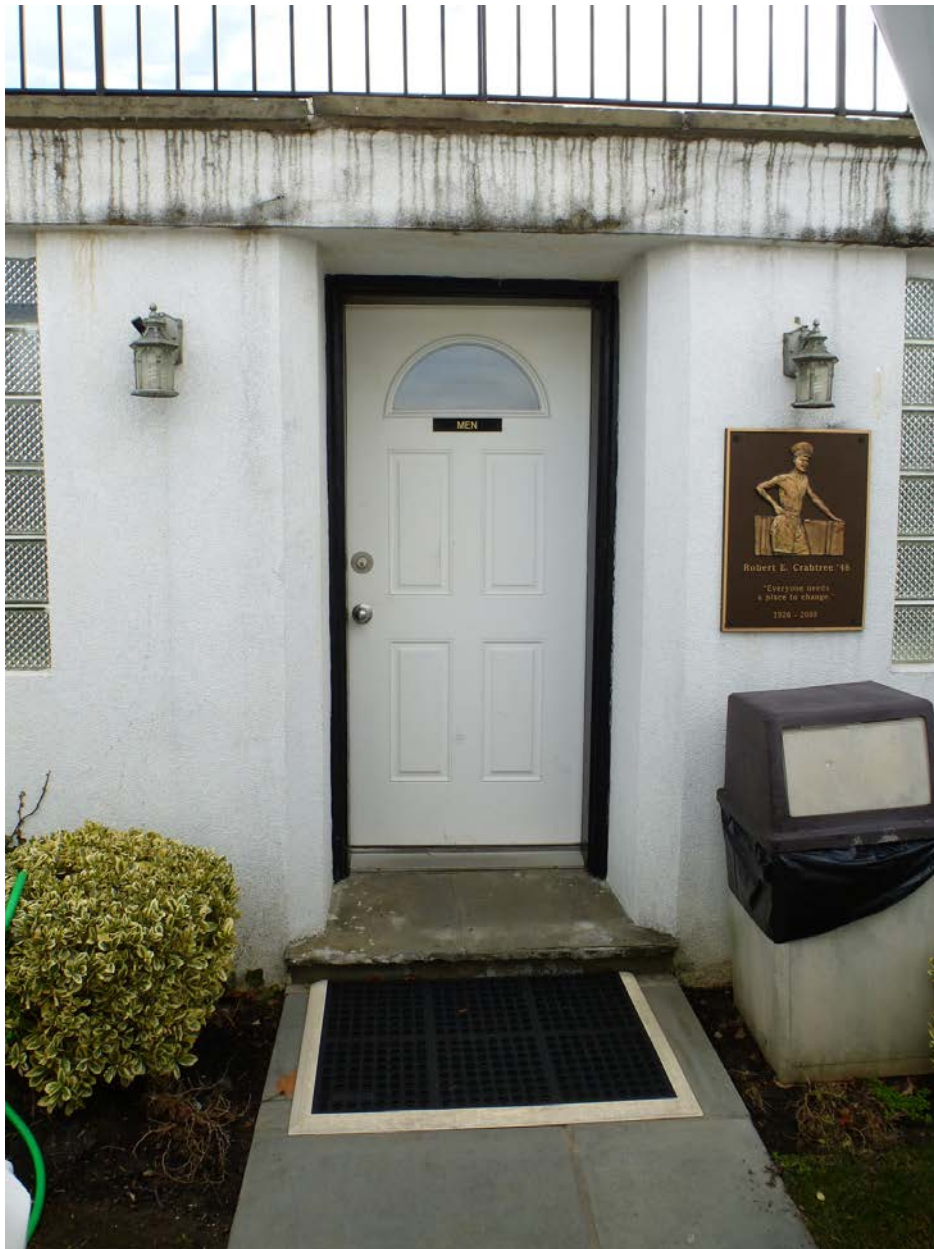
Figure 193. The replacement door into the men's shower at Crowninshield Pier and Boat House (ERDC-CERL, 2013).
