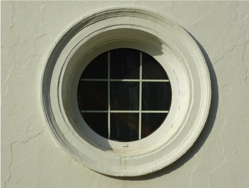
Figure 73. Round window on the east façade of Wiley Hall (ERDC-CERL, 2013).
