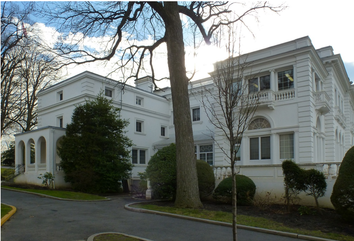
Figure 69. North façade of Wiley Hall (ERDC-CERL, 2013).
