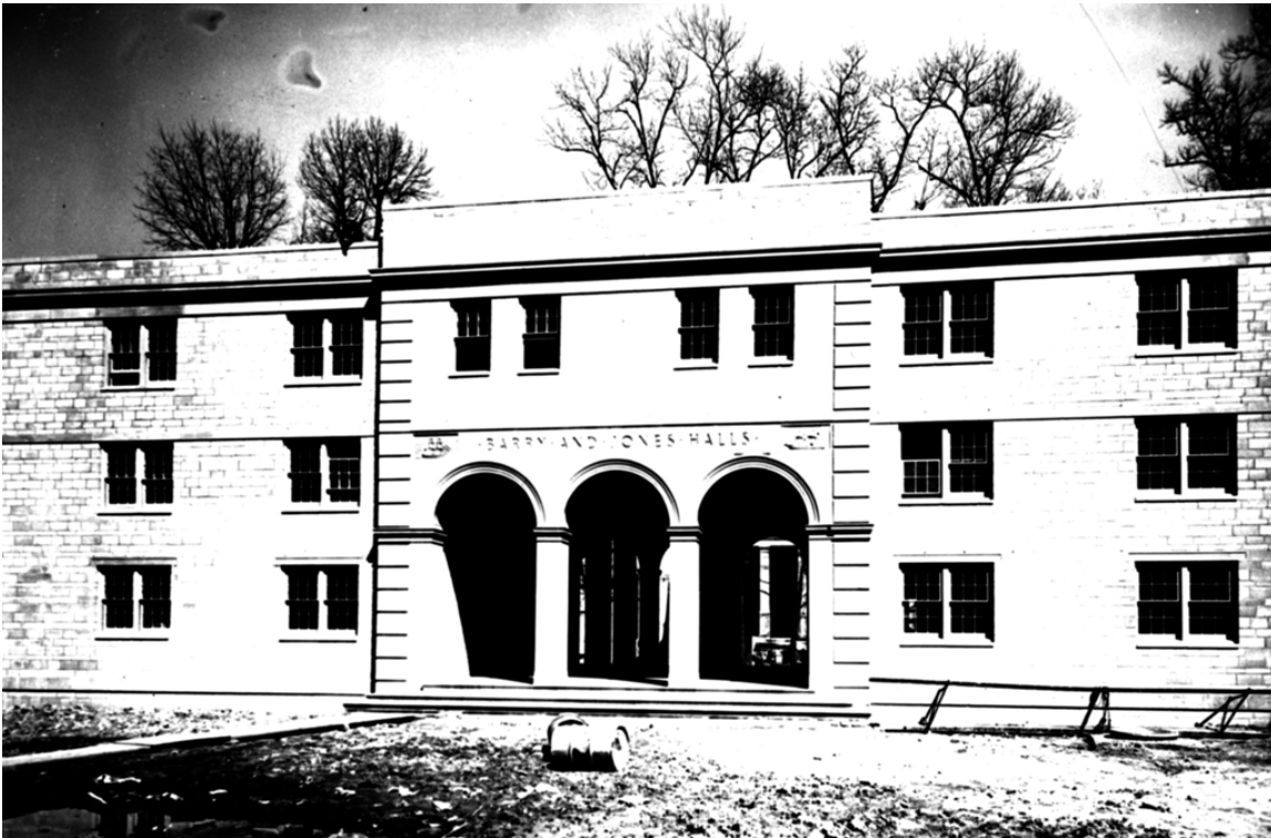
Figure 96. West façade of the Truxton Arcade that connects Barry and Jones Halls (barracks), April 1943 (Bland Library, USMMA).
