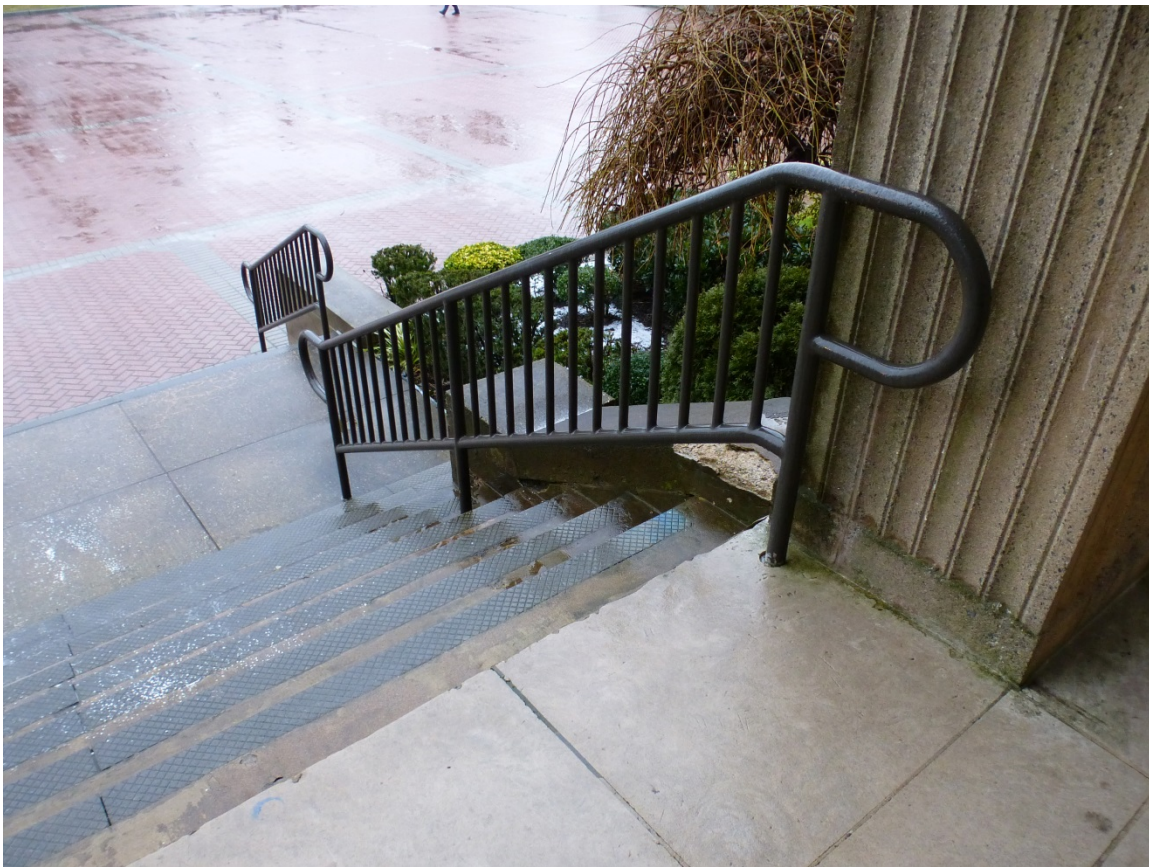
Figure 158. Non-character-defining stair railing on the portico steps (ERDC-CERL, 2013).
