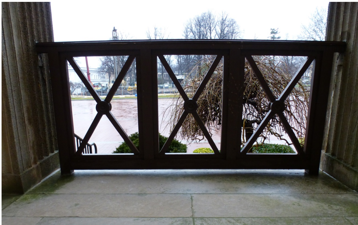
Figure 144.. Original railing on the portico on Delano Hall (ERDC-CERL, 2013).
