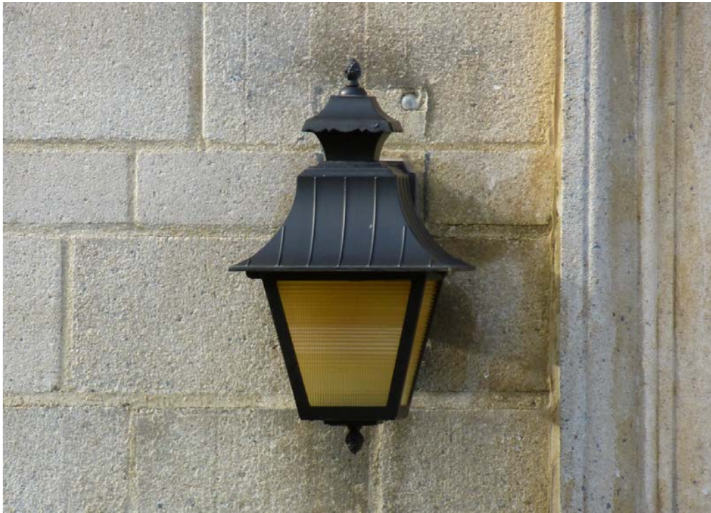
Figure 123. Replacement light fixture at east entrance to Fulton Hall (ERDC-CERL, 2013).
