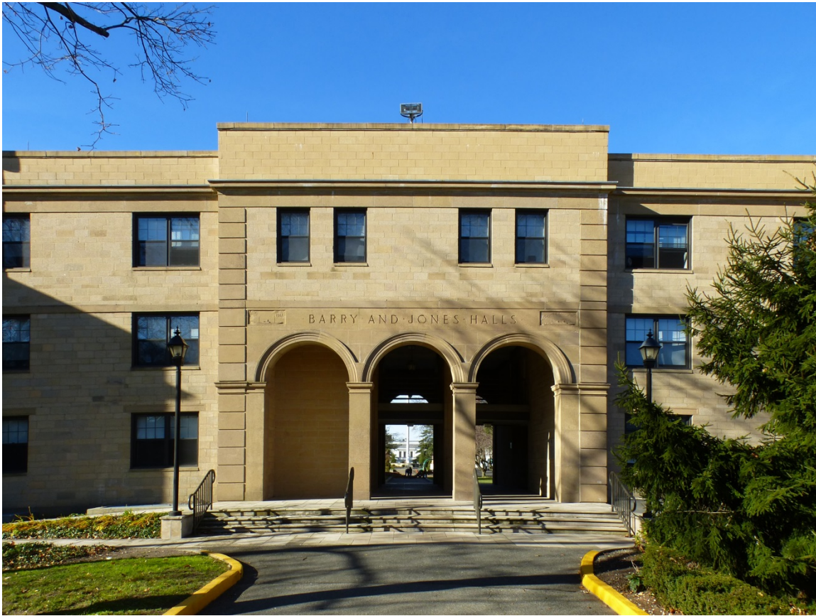
Figure 98. East façade of the Truxton Arcade (ERDC-CERL, 2013).
