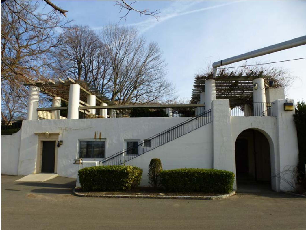
Figure 196. The paint locker north of Eldridge Pool (ERDC-CERL, 2013).
