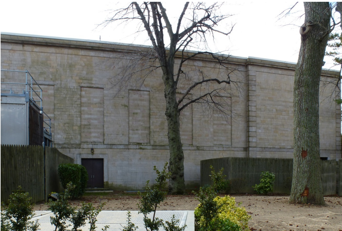
Figure 119. North façade of Bowditch Hall (ERDC-CERL, 2013).
