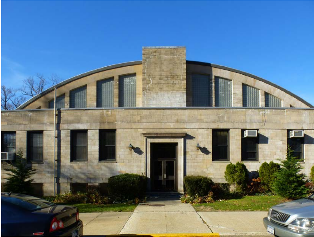
Figure 163. East façade of O'Hara Hall (ERDC-CERL, 2013).
