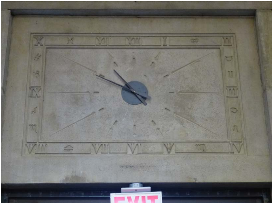
Figure 151. Cast-stone clock above doorway from dining hall to the vestibule (ERDC-CERL, 2013).
