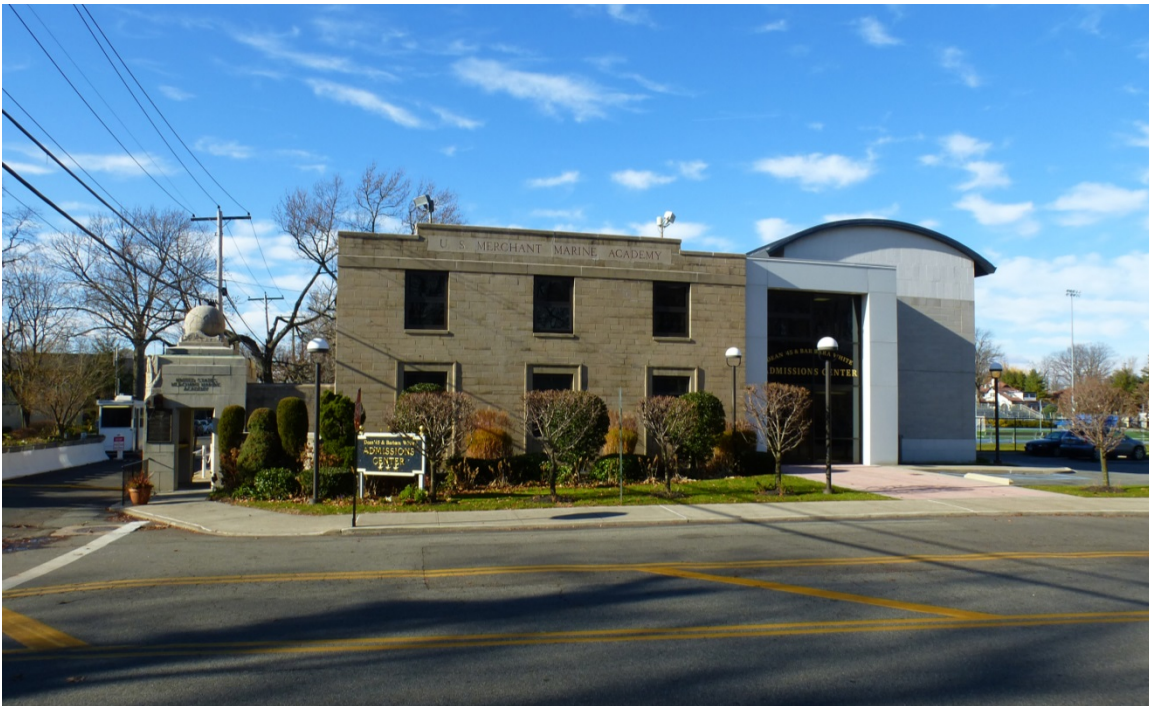
Figure 174. The east façade of the Admissions Center with addition to the right (ERDC-CERL, 2013).
