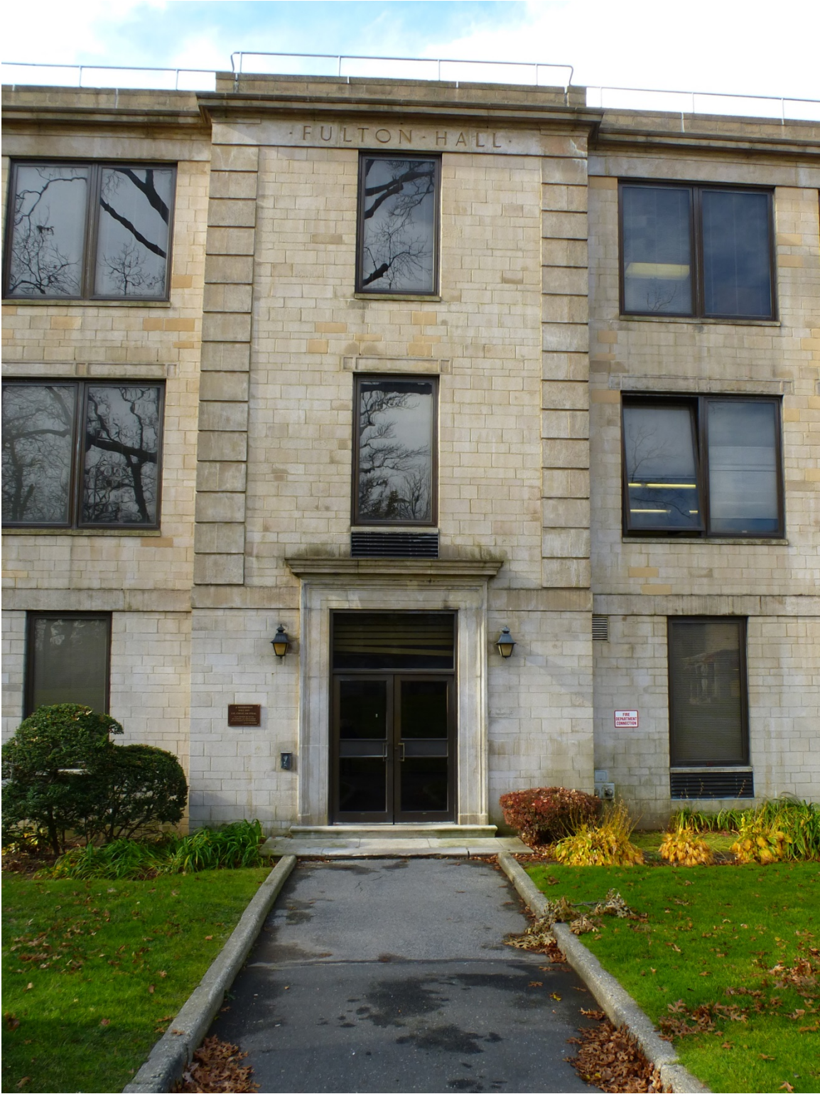
Figure 115. East entrance to Fulton Hall (ERDC-CERL, 2013).
