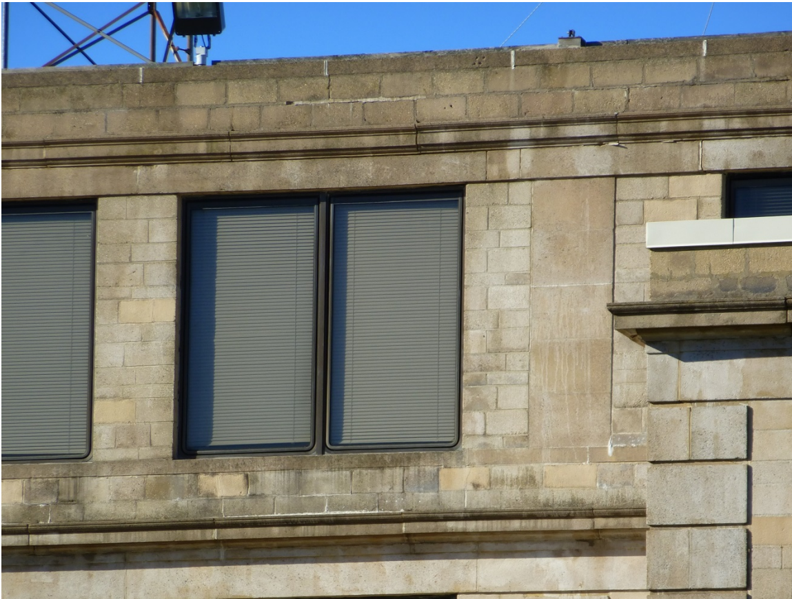
Figure 127. Replacement windows in original openings on Bowditch Hall (ERDC-CERL, 2013).
