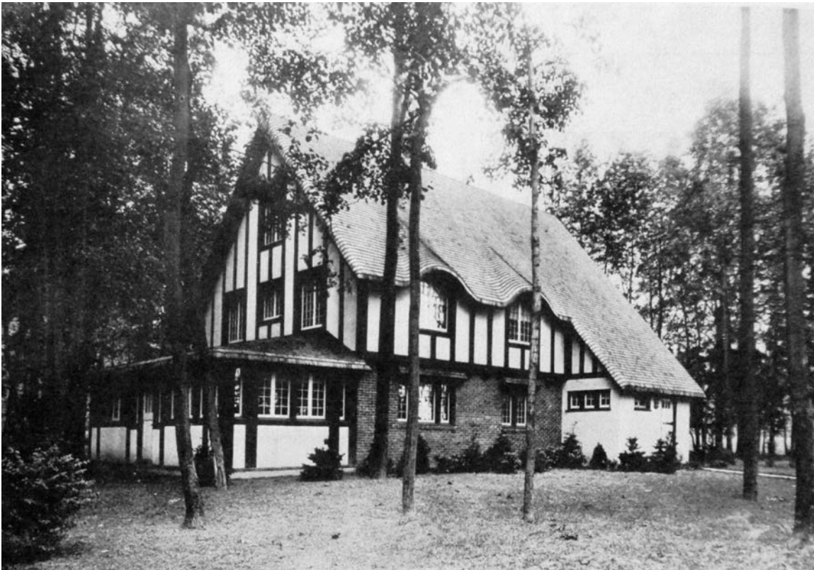
Figure 63. South façade of Quarters C (Vreeland house) in 1914 ( Architectural Record ).
