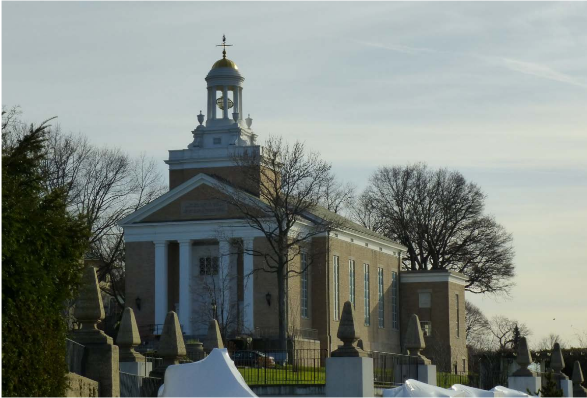
Figure 185. Northwest oblique of the chapel (ERDC-CERL, 2013).
