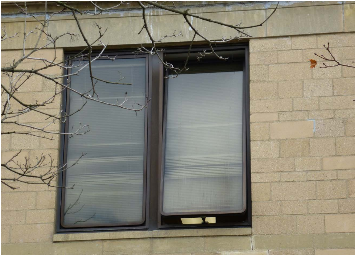
Figure 139. Replacement awning (tilt) window on Samuels Hall (ERDC-CERL, 2013).
