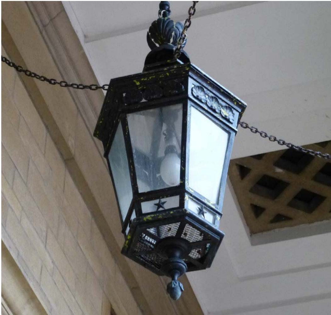
Figure 147. Detail of original light fixture on the portico (ERDC-CERL, 2013).
