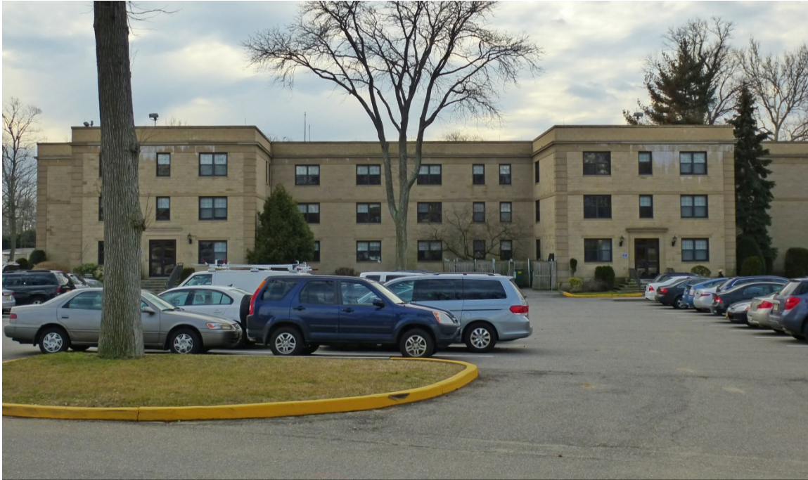
Figure 100. North façade of Jones Hall (ERDC-CERL, 2013).
