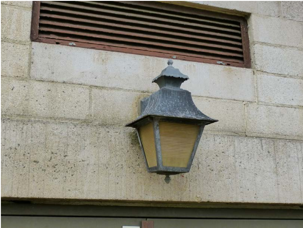
Figure 172. Replacement exterior light fixture on O'Hara Hall (ERDC-CERL, 2013).
