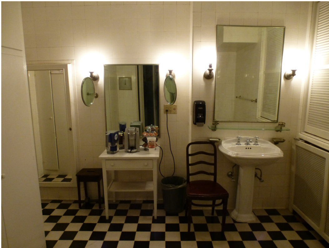
Figure 84. One of the original Bendel/Chrysler bathrooms (with a replacement sink) in Wiley Hall (ERDC-CERL, 2013).
