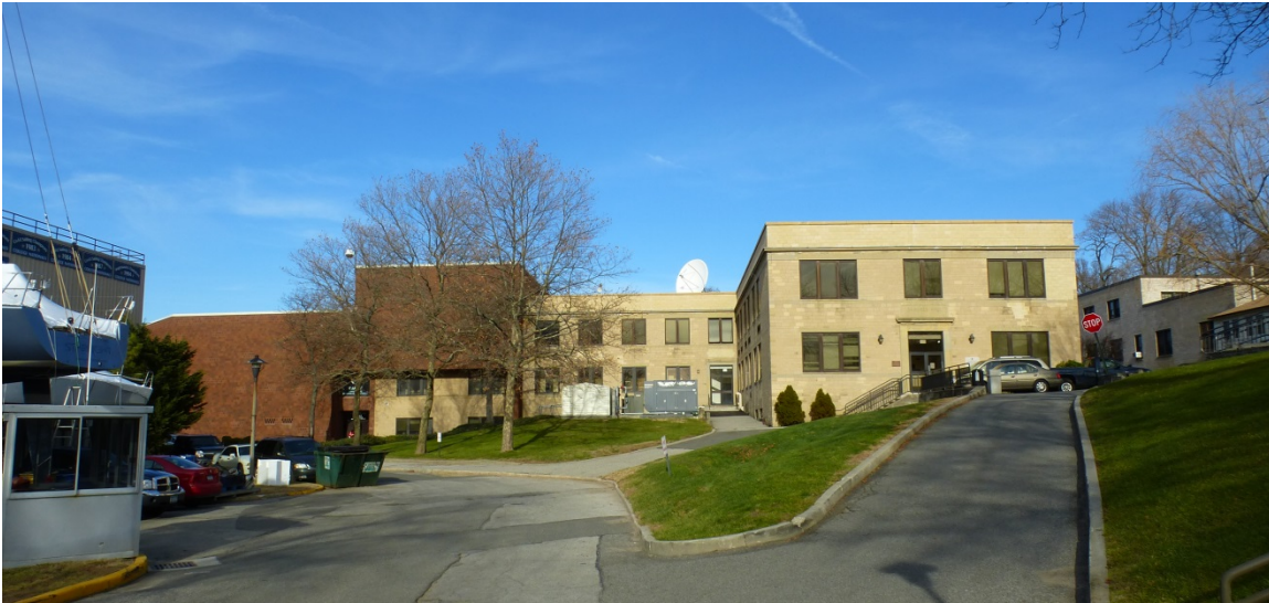
Figure 136. South façade of Samuels Hall, with the 1975 addition on the left (ERDC-CERL, 2013).
