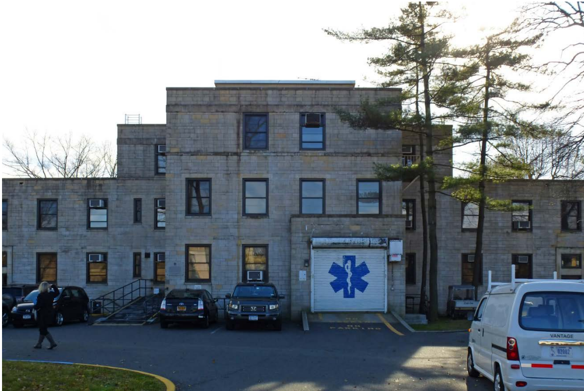
Figure 179. North façade of Patten Clinic (ERDC-CERL, 2013).
