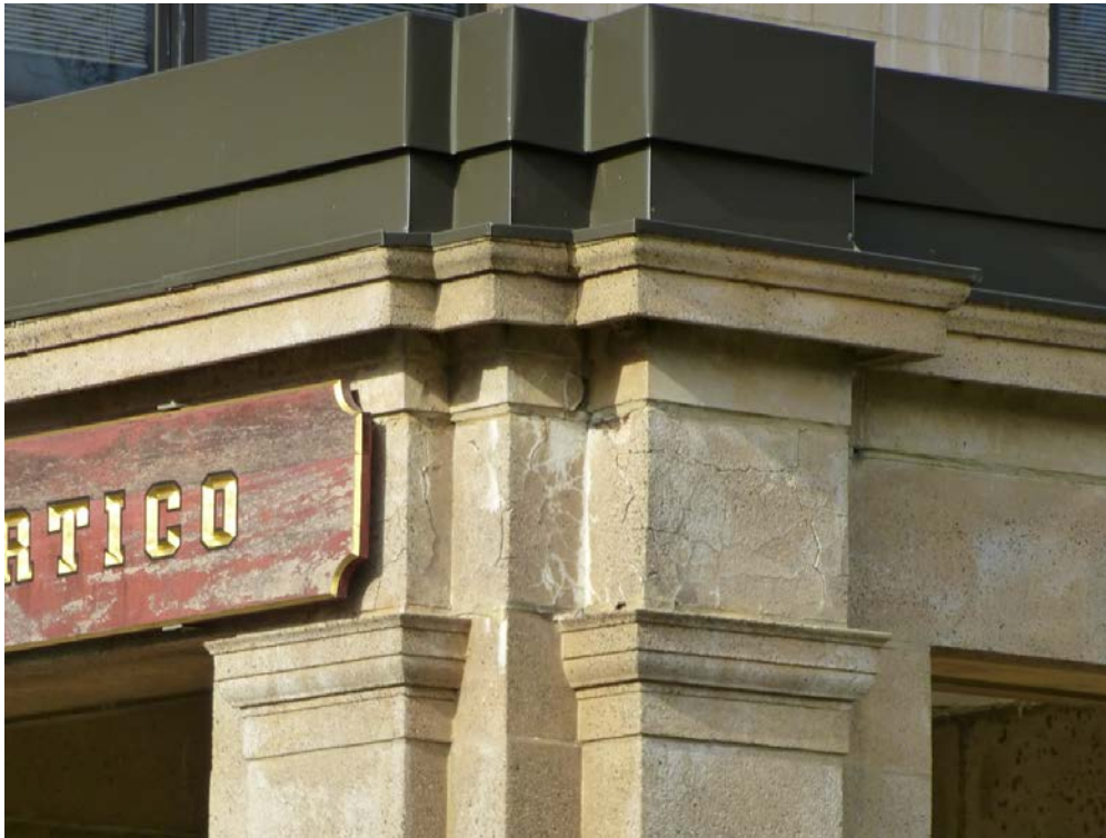
Figure 121. Detail of southwest corner of portico entrance to Fulton Hall showing cast-stone architectural elements (ERDC-CERL, 2013).
