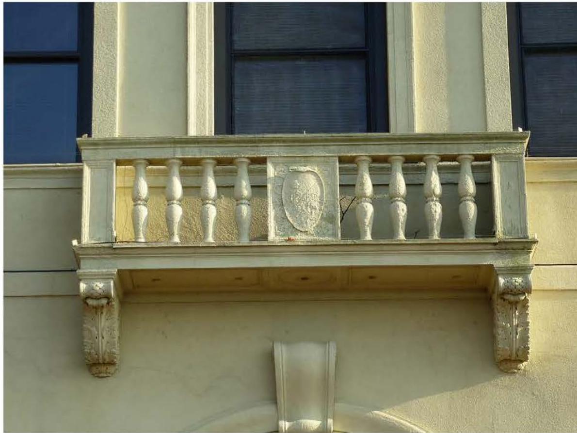
Photo 9. View to the east of the balcony on the second floor.
