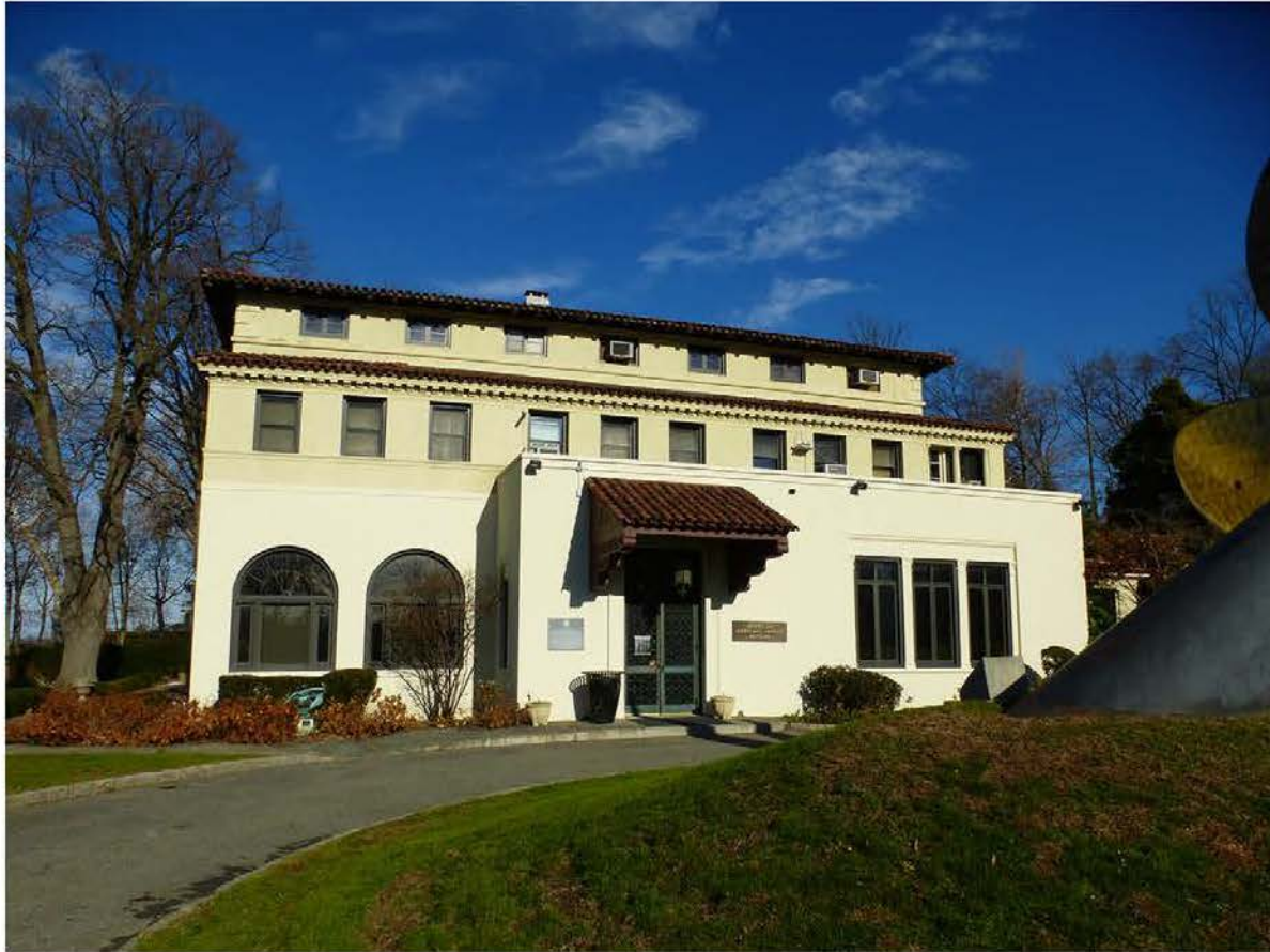
Photo 5. View to north of the front facade.
