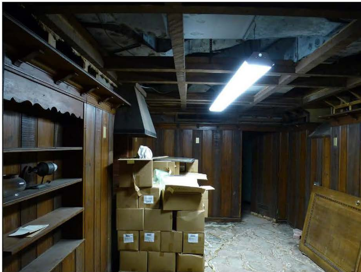
Photo 51. View to the north of the tap room in the basement of the music room addition.
