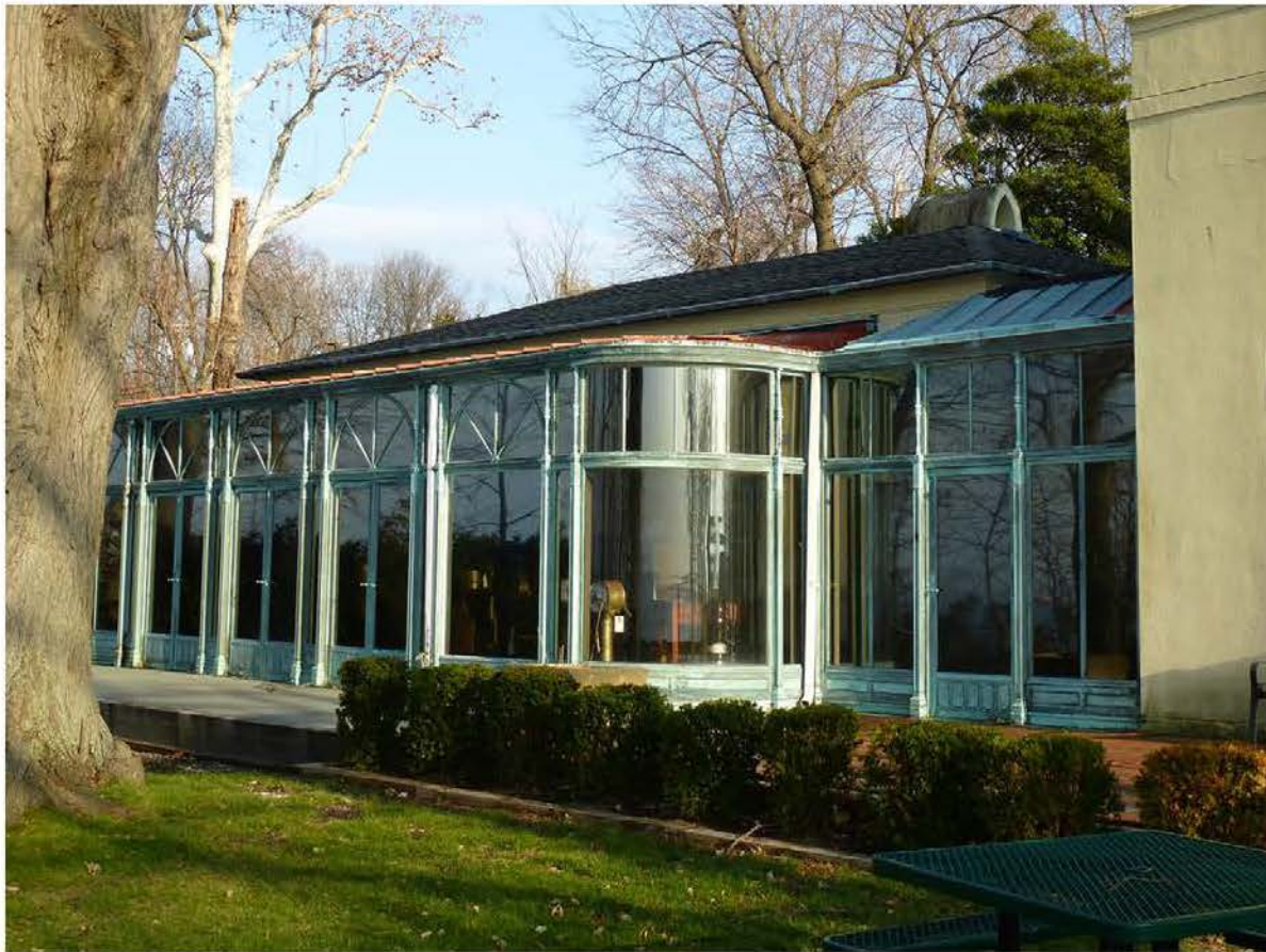
Photo 11. View to the northeast of the solarium on the west facade of the music room addition.
