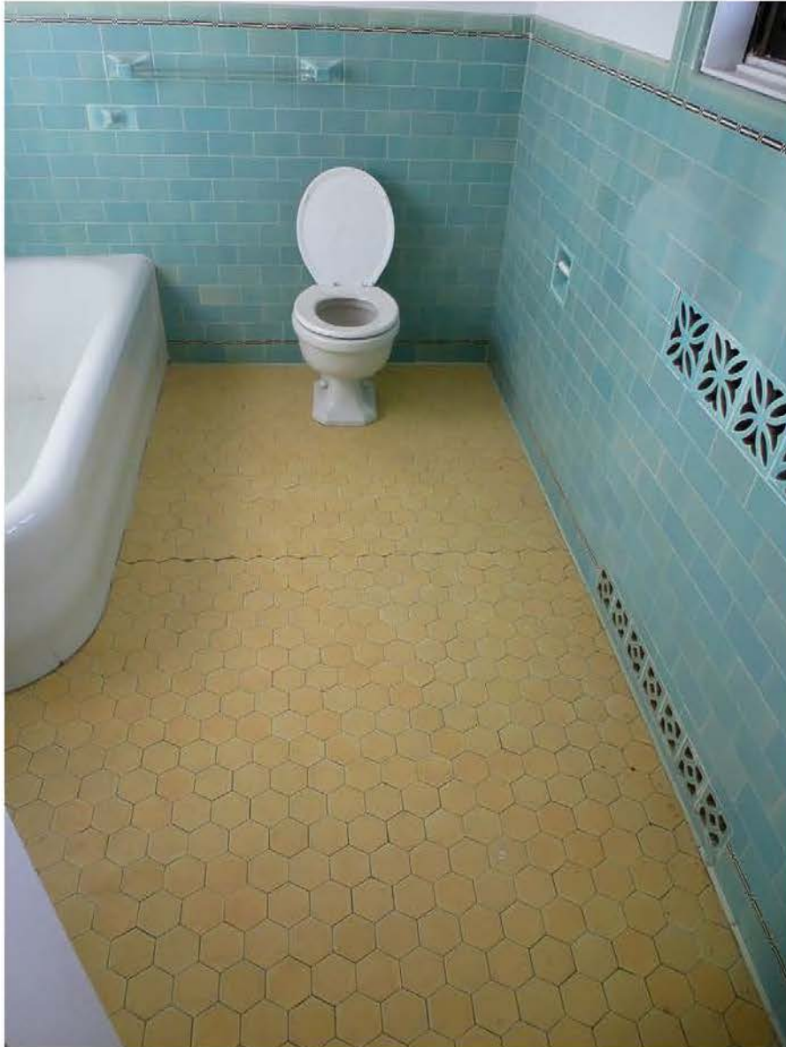
Photo 48. View to the east of the third-floor southwest bathroom.
