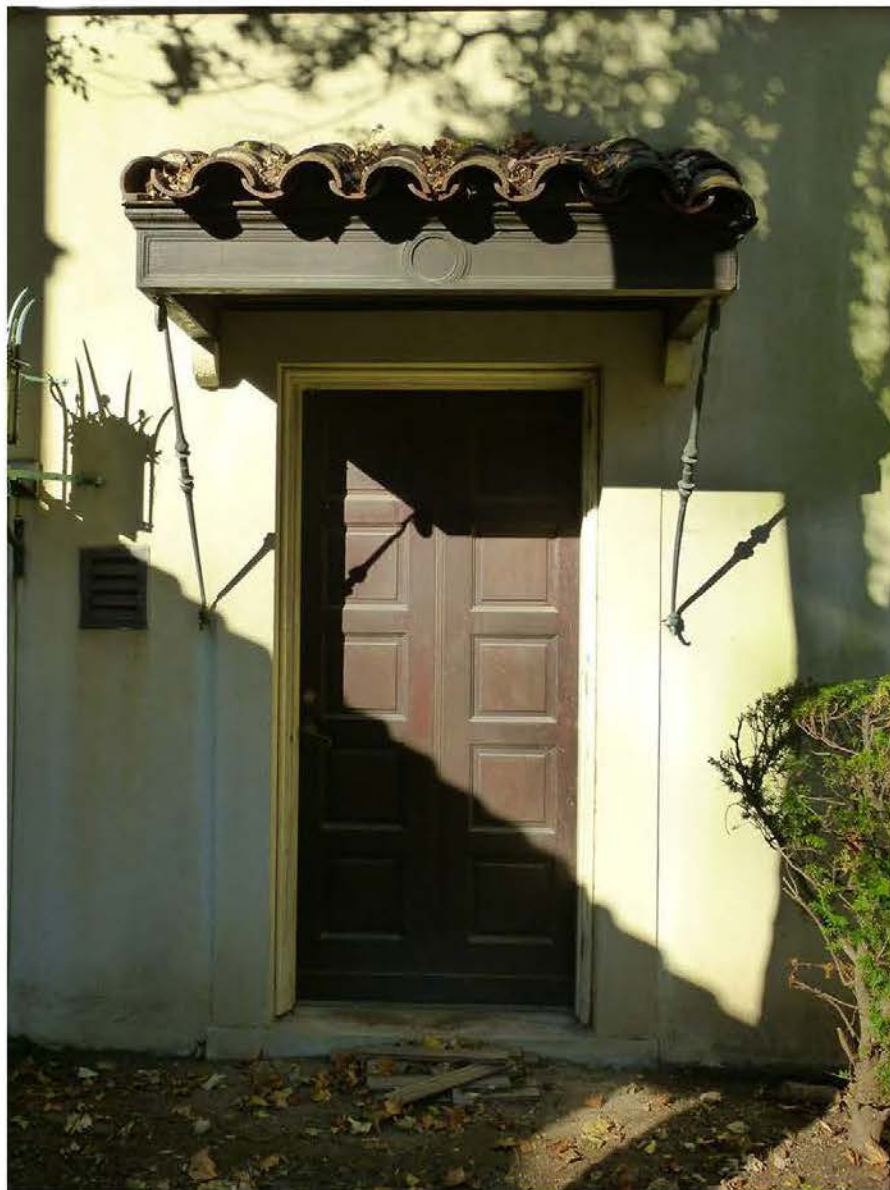
Photo 14. View to the west of the south entrance door into the music room addition.
