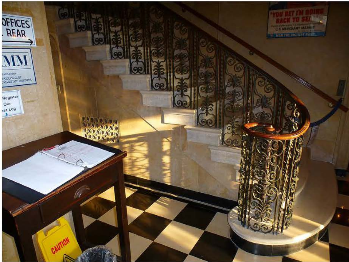
Photo 18. View to the northeast showing the marble staircase in the foyer and the wrought-iron balustrade designed by Greville Rickard in 1929.
