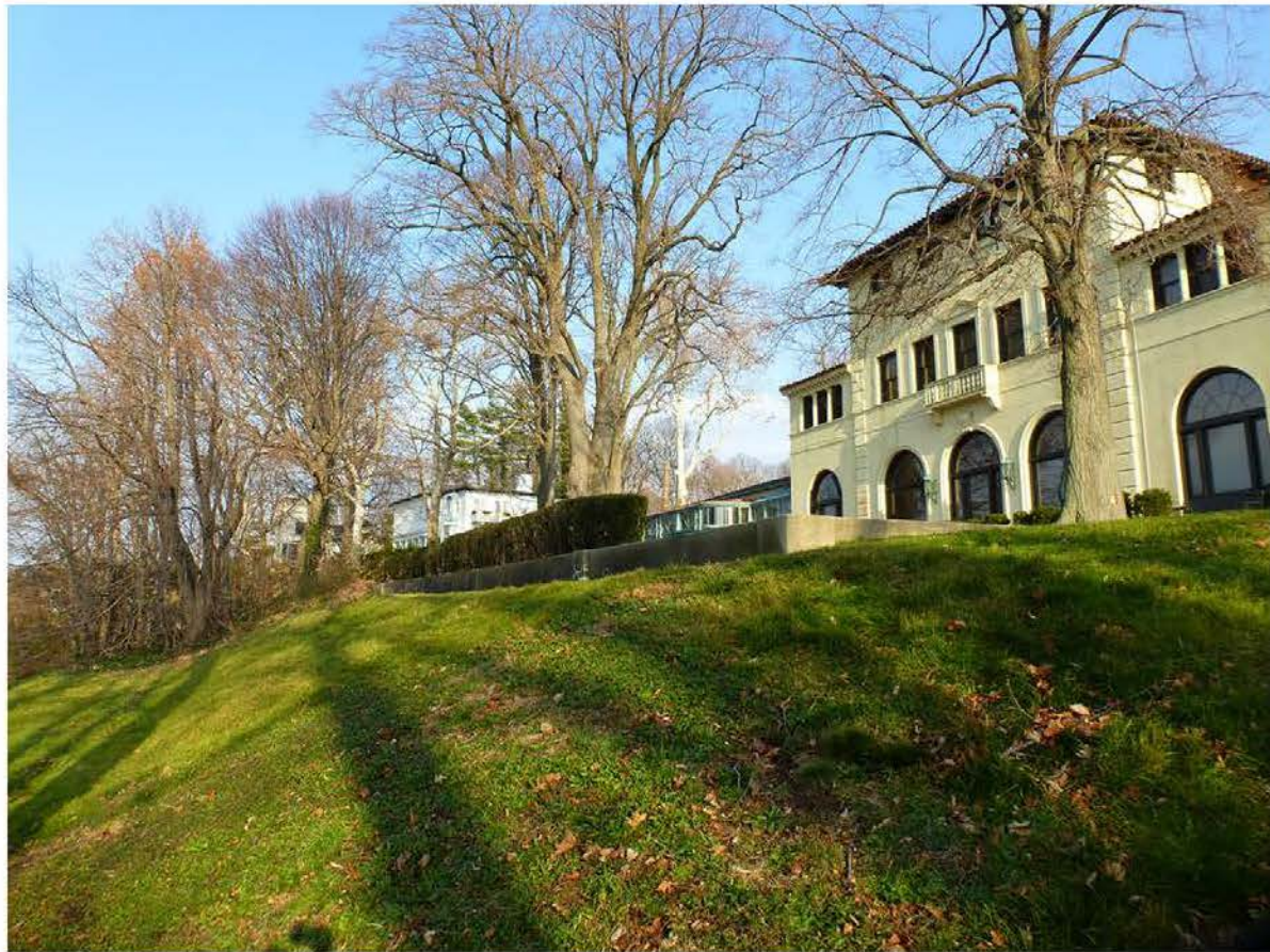
Photo 4. View to north showing the slope from the mansion down to the Long Island shore.
