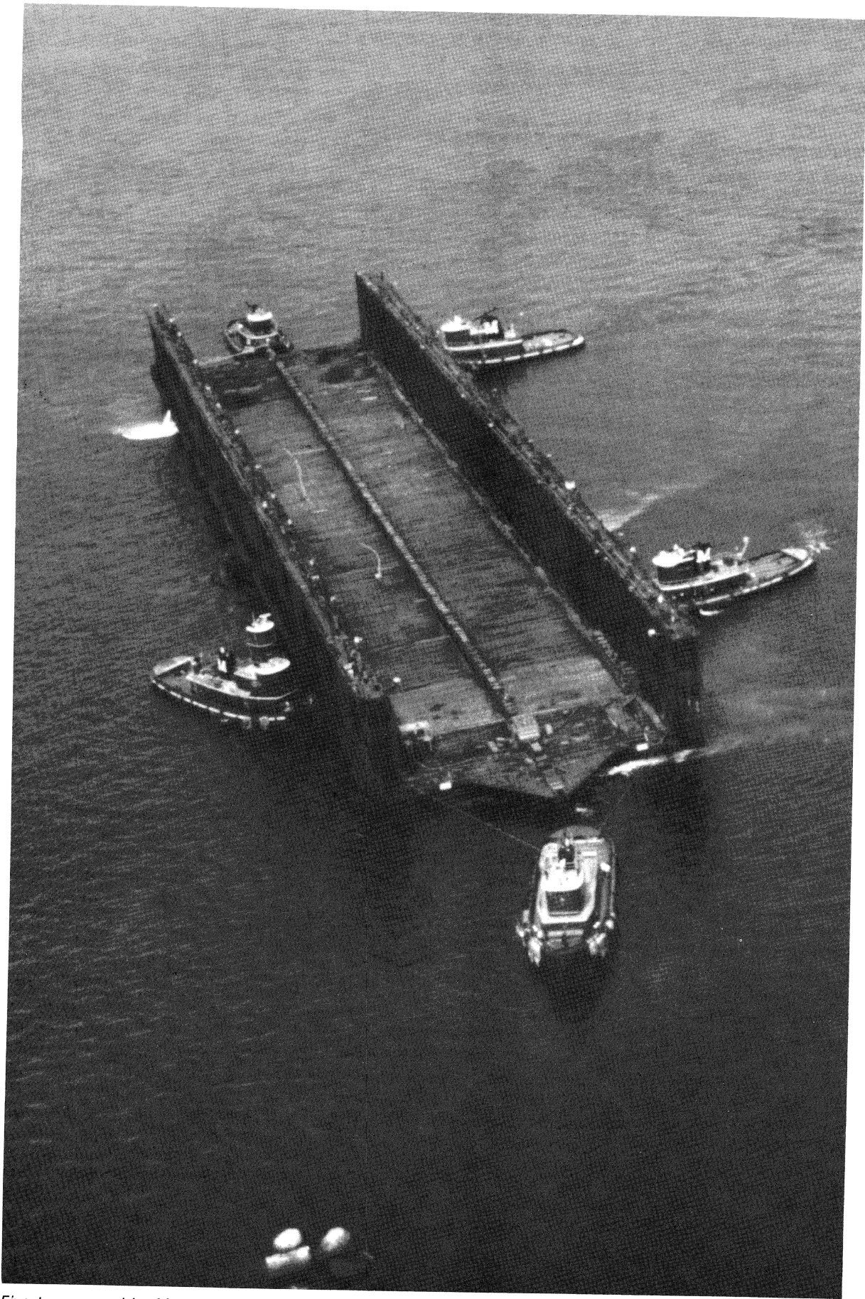
Five tugs owned by Moran Towing & Transportation Co. maneuver a 700-foot-long floating drydock across New York Harbor as part of a move involving a shipyard formerly operated by Todd Shipyards Corp.
